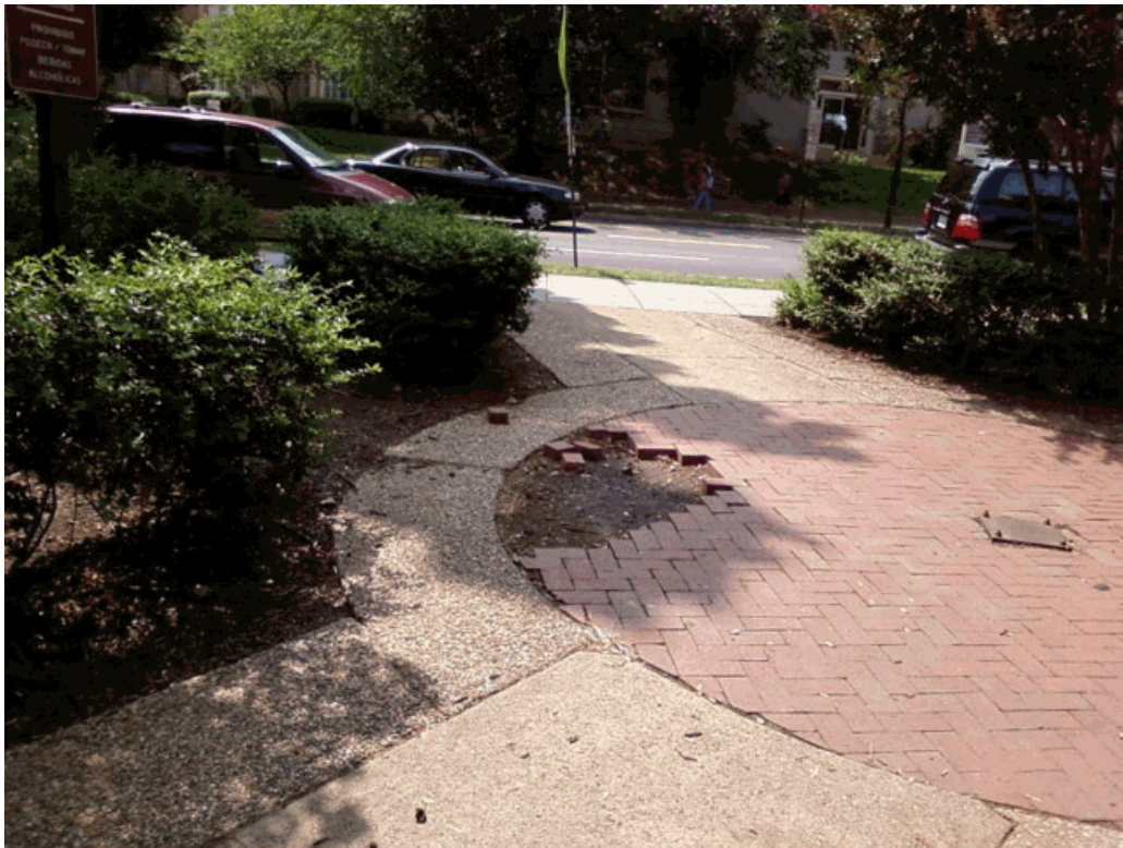
Bricks are loose and missing from the drinking fountain circle. (NCR CLP 2007).
