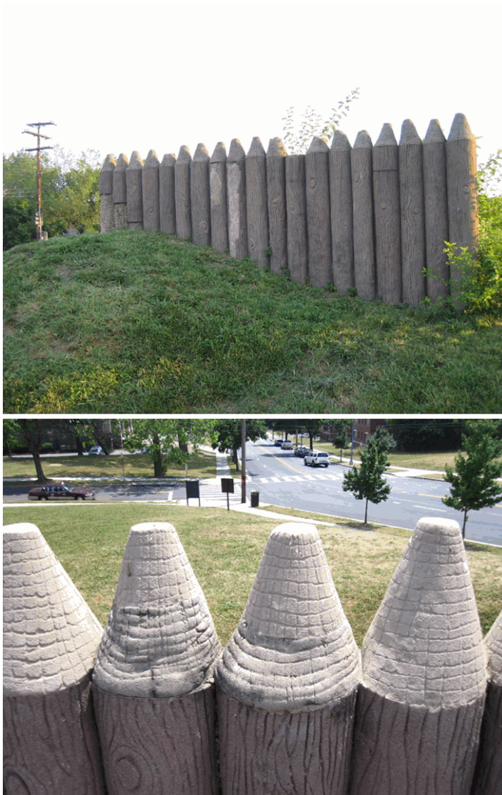
Top: revetments prior to 2010 rehabilitaion work (ROCR). Bottom: following repair. The concrete patching will blend with the color of the historic material once it has had a chance to weather (CLP June 2010).
