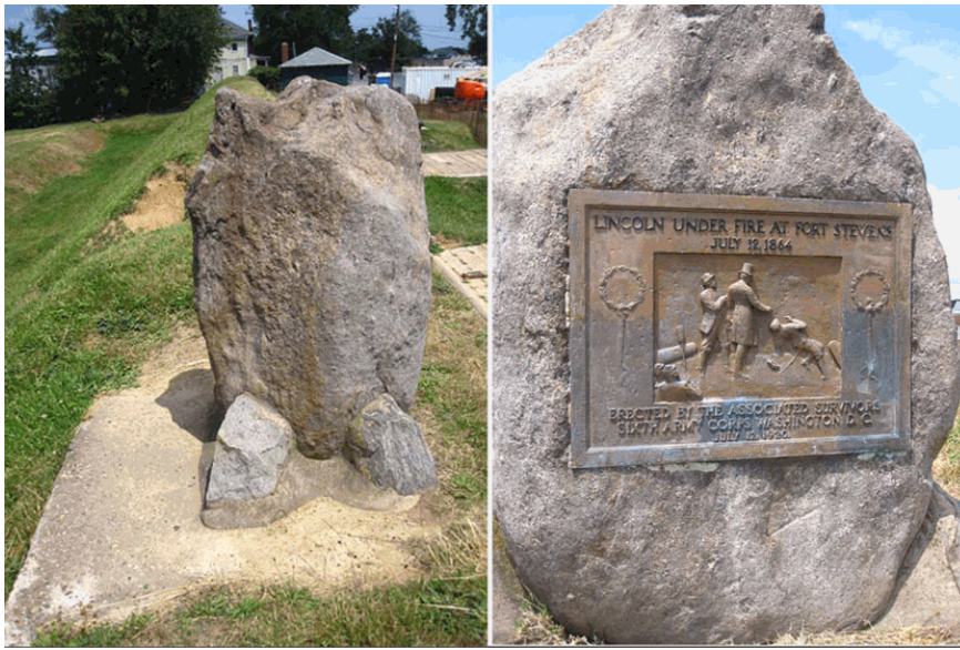
Streaking on the stone and portions of the monument's original pedestal are visible; VI Army Corps plaque showing effects of polish tests (CLP June 2010).
