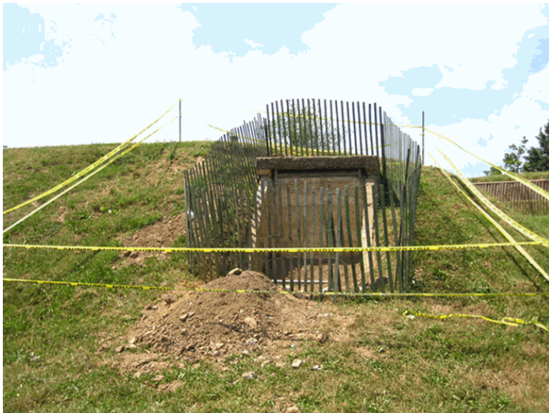
Magazine door replacement work underway, 2010 (CLP June 2010).
