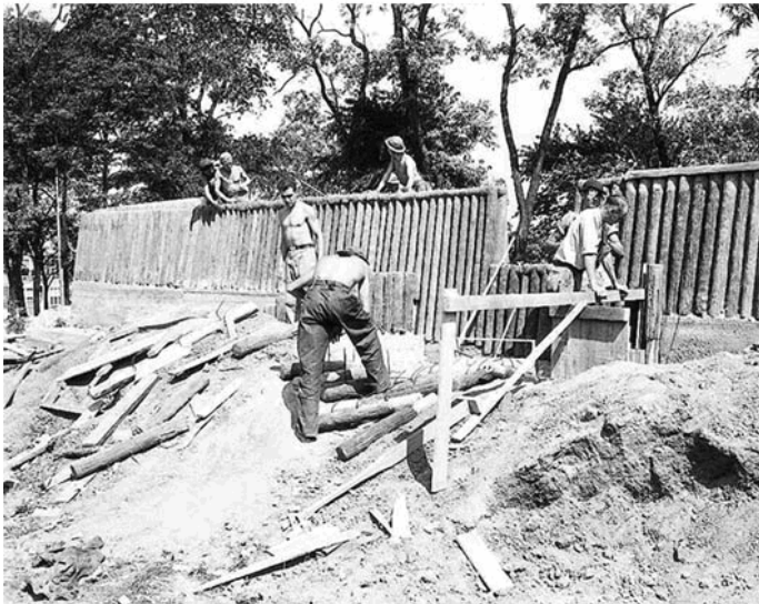
Civilian Conservation Corps reconstruction underway, 1936 (both photos, "Fort Stevens, September 16, 1936." MRCE).
