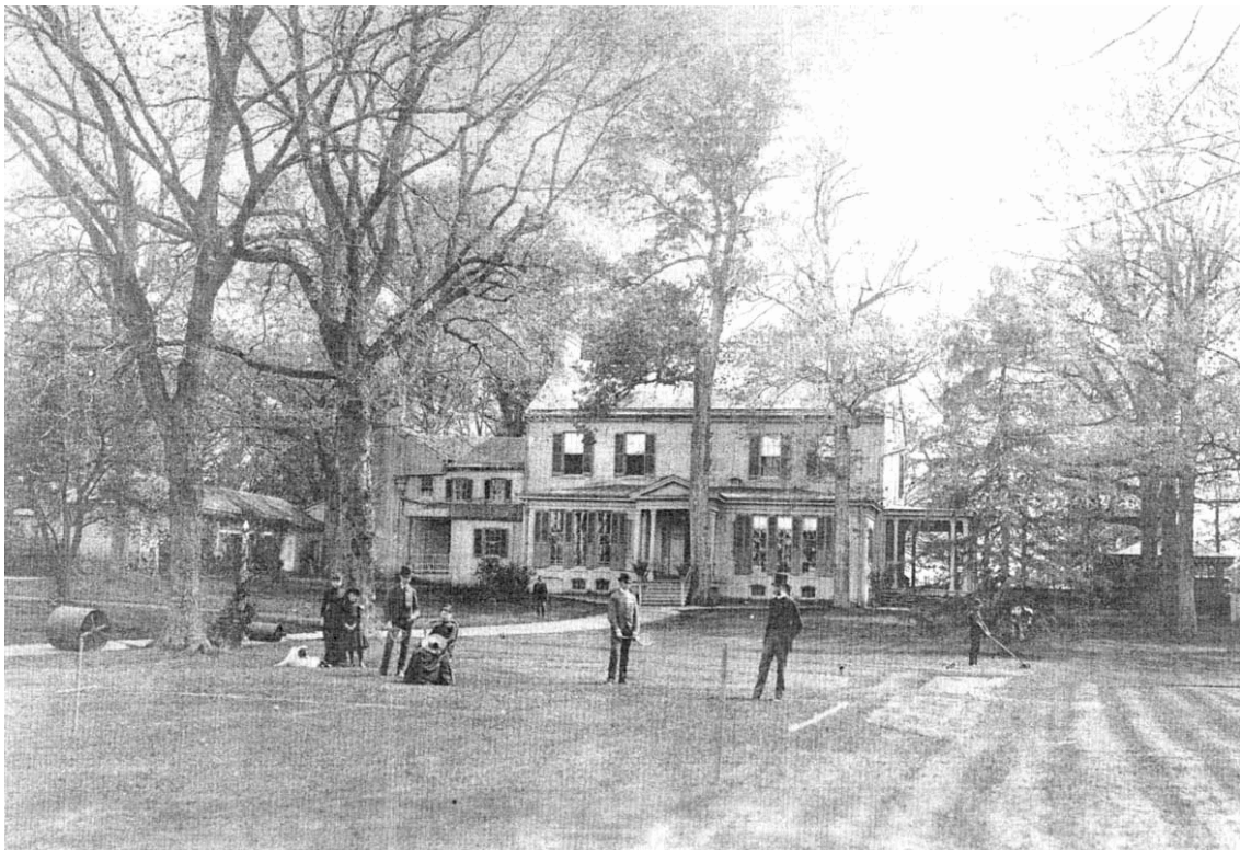
North elevation of house and grounds, no date. Note the lawn rollers on the walk on the axis north from the house, and men holding badminton rackets (Library of Congress, Prints and Photographs Division).
