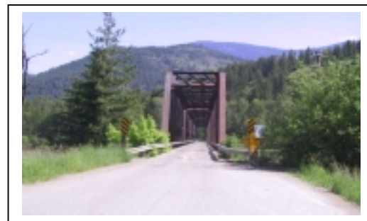
Figure 34: The bridge shown above will be converted from a vehicle to pedestrian bridge.
