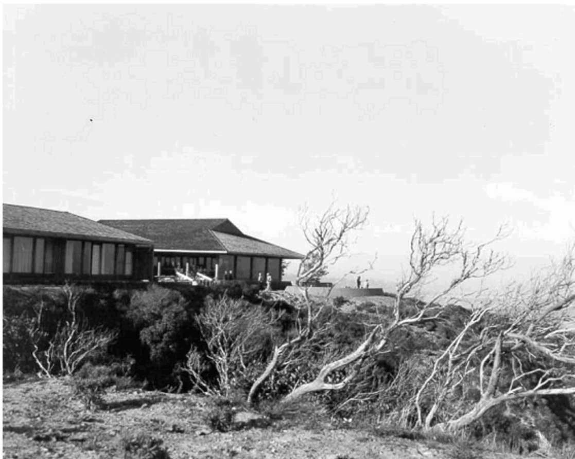
History #5: Cabrillo MN Visitor Center. View of Administration and View Building. 1968. Cabrillo NM Interpretation Division Photo Collection.
