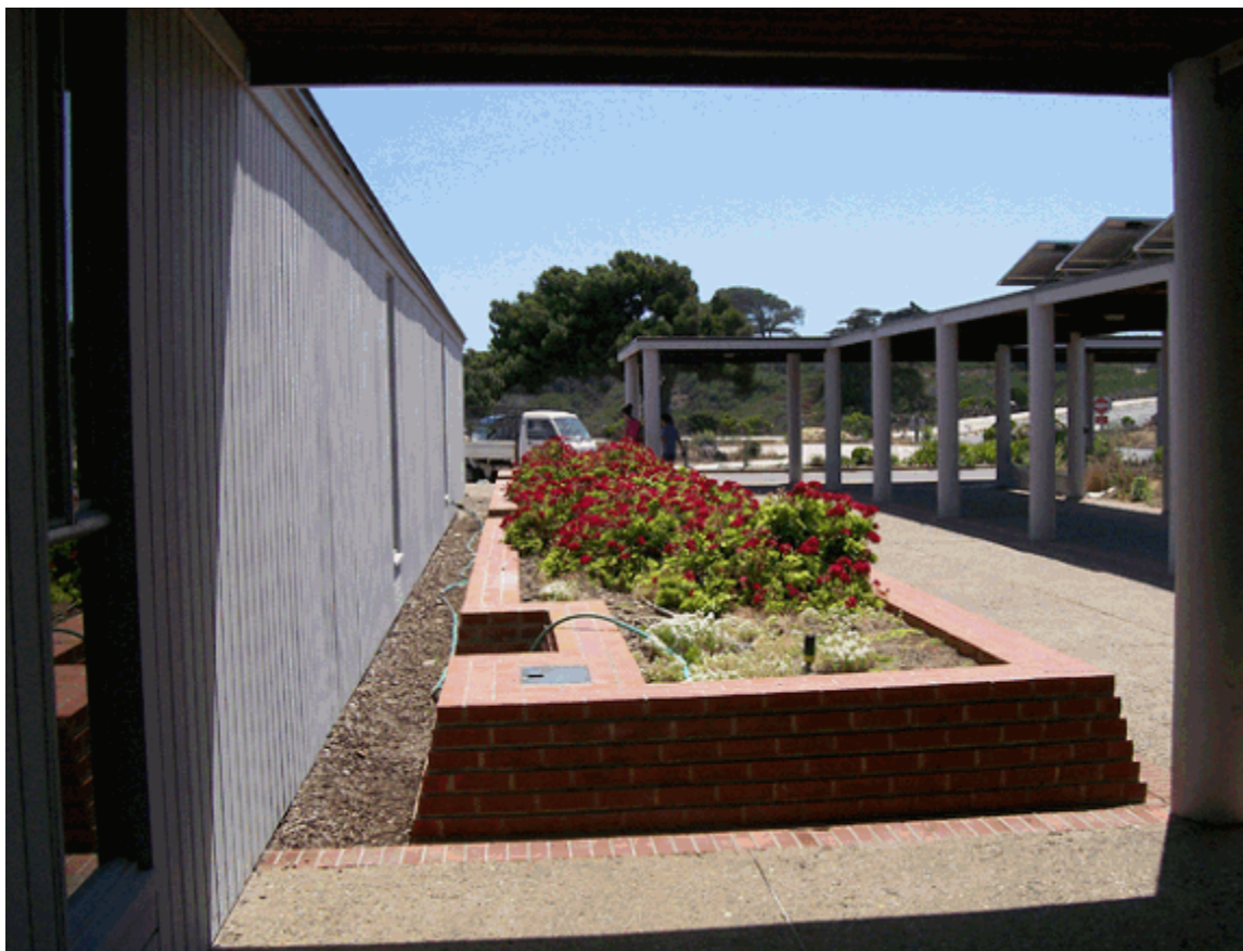
Buildings and Structures #2: Fountain, view looking south Photo by Jason M. Richards, NPS CABR July 31, 2008
