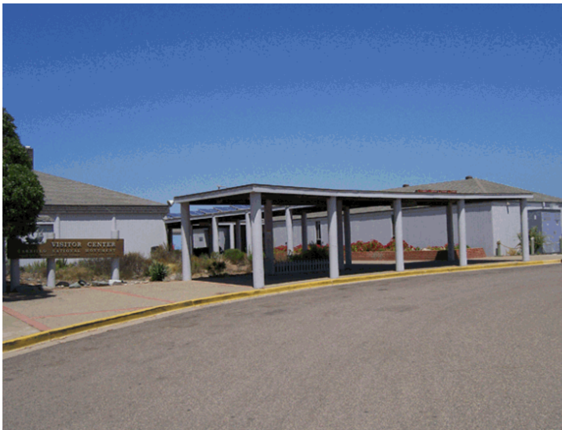
Buildings and Structures #1: Visitor center entrance and pergola, view looking northeast Photo by Jason M. Richards, NPS CABR July 31, 2008
