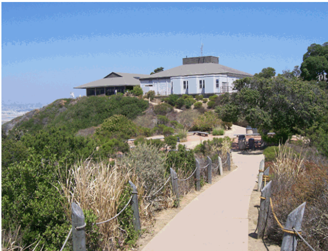
Buildings and Structures #5: Ballast View Overlook, view looking east Photo by Jason M. Richards, NPS CABR July 31, 2008
