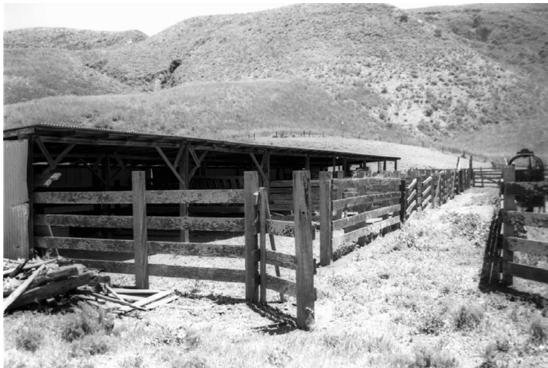
Buildings and Structures #3: A view along the horse barn within the corral complex. The cattle squeeze is on the right. (PGSO, CLI, CHIS-N-0008-5, 2002)
