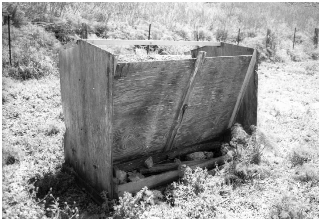
Small Scale Features #6: A view of the eastern feed crib located in the corral complex. (PGSO, CLI, CHIS-N-0008-13, 2002)
