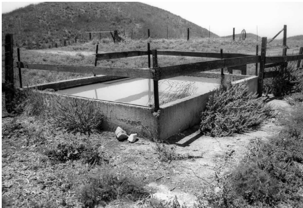
Small Scale Features #5: The western concrete trough completely within the corral complex at Rancho del Norte. (PGSO, CLI, CHIS-N-0008-14, 2002)
