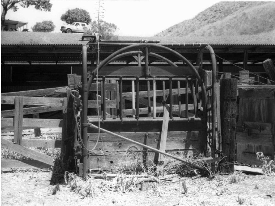
Small Scale Features #1: The metal cattle squeeze, located near the horse barn and medicine shed. (PGSO, CLI, CHIS-N-0008-4, 2002)
