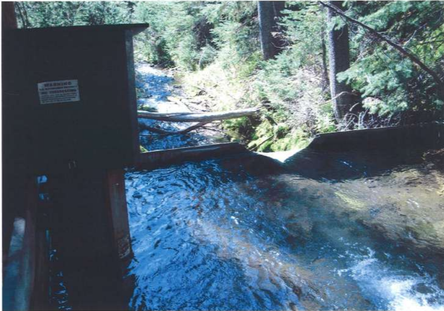
Cross Section: Annie Spring Weir USGS Gaging Station 11503000, Annie Spring near Crater Lake, Oregon Annie Spring Weir located below Rim Drive bridge. View from upstream to downstream.
