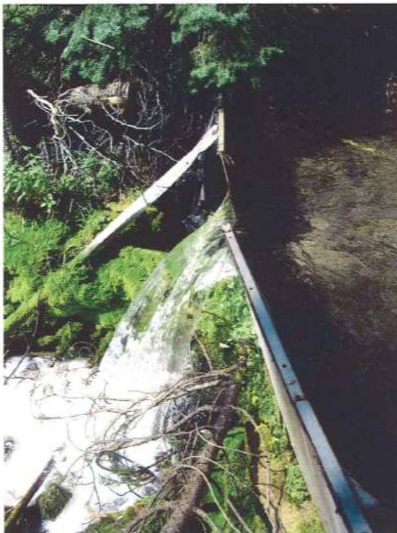
Cross Section: Annie Spring Weir USGS Gaging Station 11503000, Annie Spring near Crater Lake, Oregon Annie Spring Weir located below Rim Drive bridge. View from left bank to right bank.
