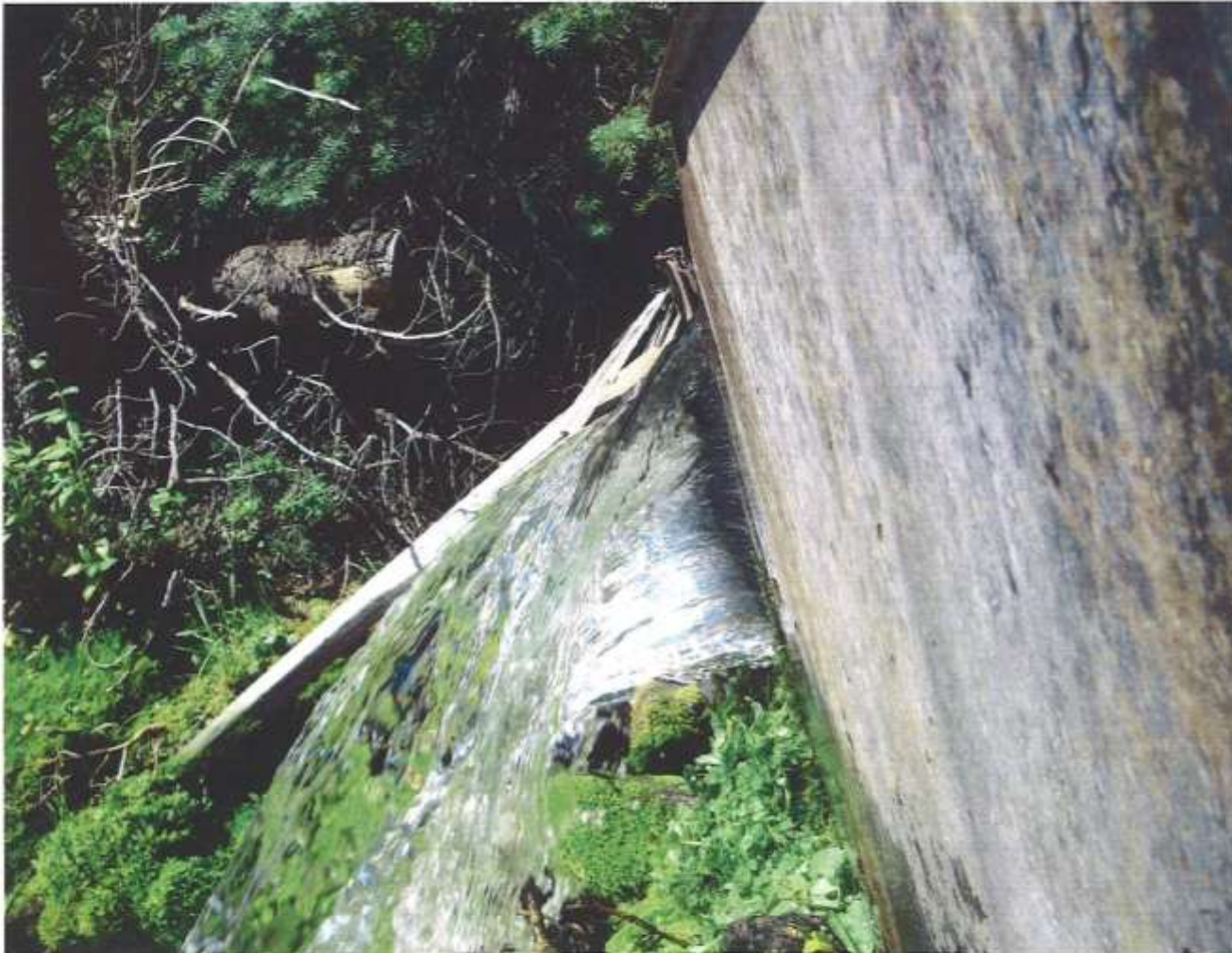
Cross Section: Annie Spring Weir USGS Gaging Station 11503000, Annie Spring near Crater Lake, Oregon Annie Spring Weir located below Rim Drive bridge. View from left bank to right bank.
