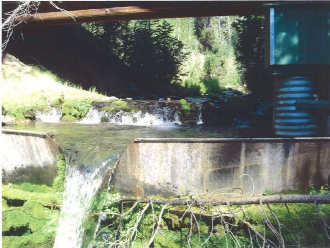
Cross Section: Annie Spring Weir USGS Gaging Station 11503000, Annie Spring near Crater Lake, Oregon Annie Spring Weir located below Rim Drive bridge. View from downstream to upstream.
