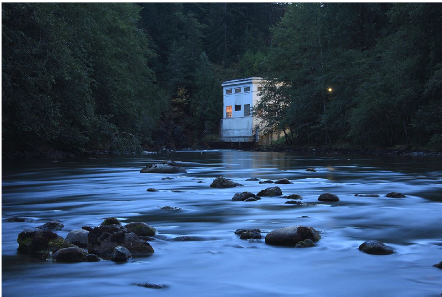
The Glines Canyon dam power house. Photo by John McMillan, NOAA
