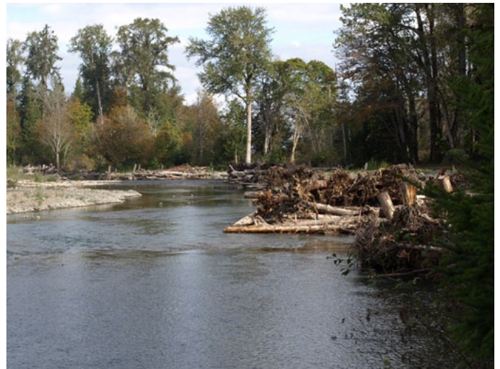
Engineered log jams installed in the lower Elwha River. Photo by Mike McHenry, Lower Elwha Klallam Tribe
