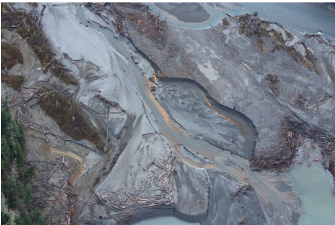
The former Lake Mills reservoir in transition. Photo by the National Park Service
