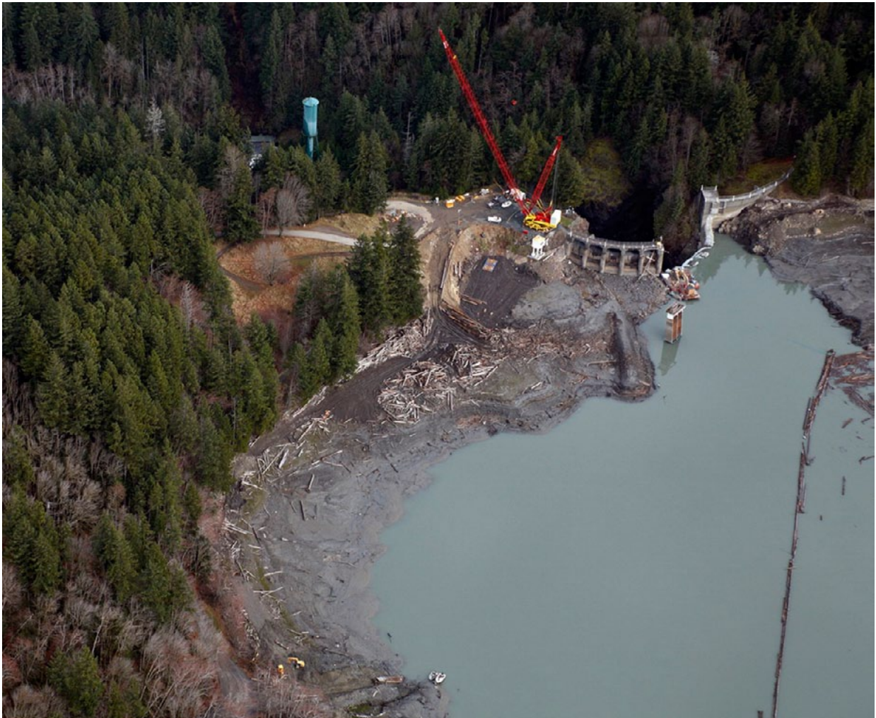
An aerial view of the Glines Canyon dam during deconstruction. Photo by John Gussman, Doubleclick Productions
