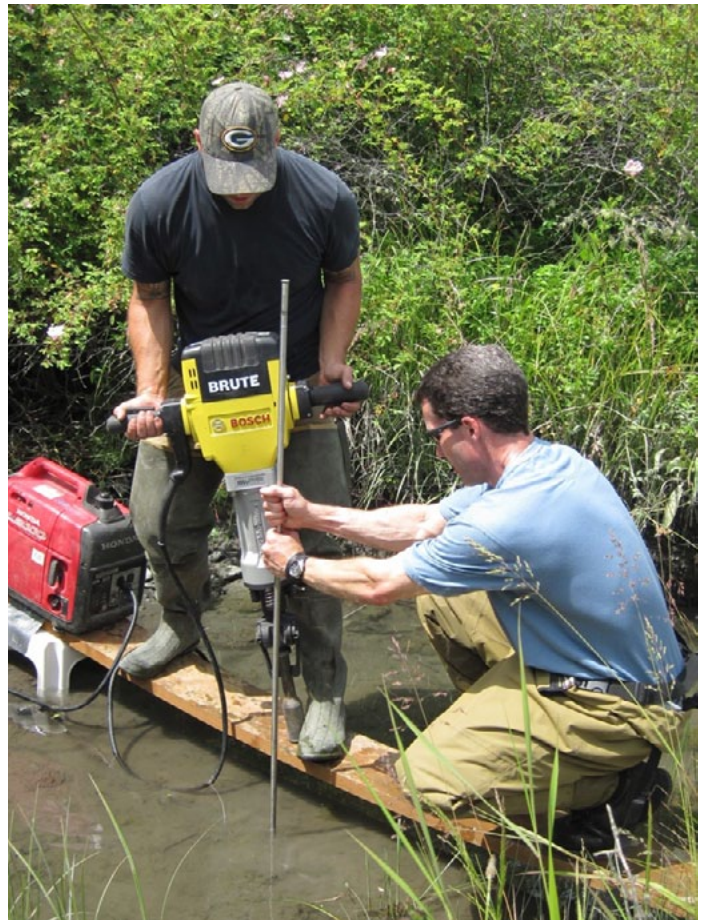
Lower Elwha Klallam Tribe scientists install equipment to monitor sediment dynamics in the Elwha River Estuary. Photo by the Lower Elwha Klallam Tribe
