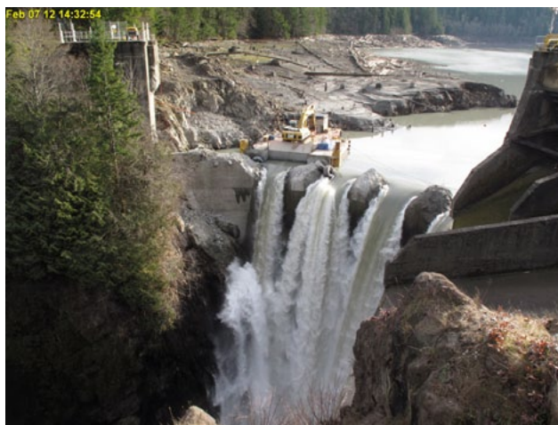
Glides Canyon Dam during deconstruction, February 1st, 2012. Photo by the National Park Service
