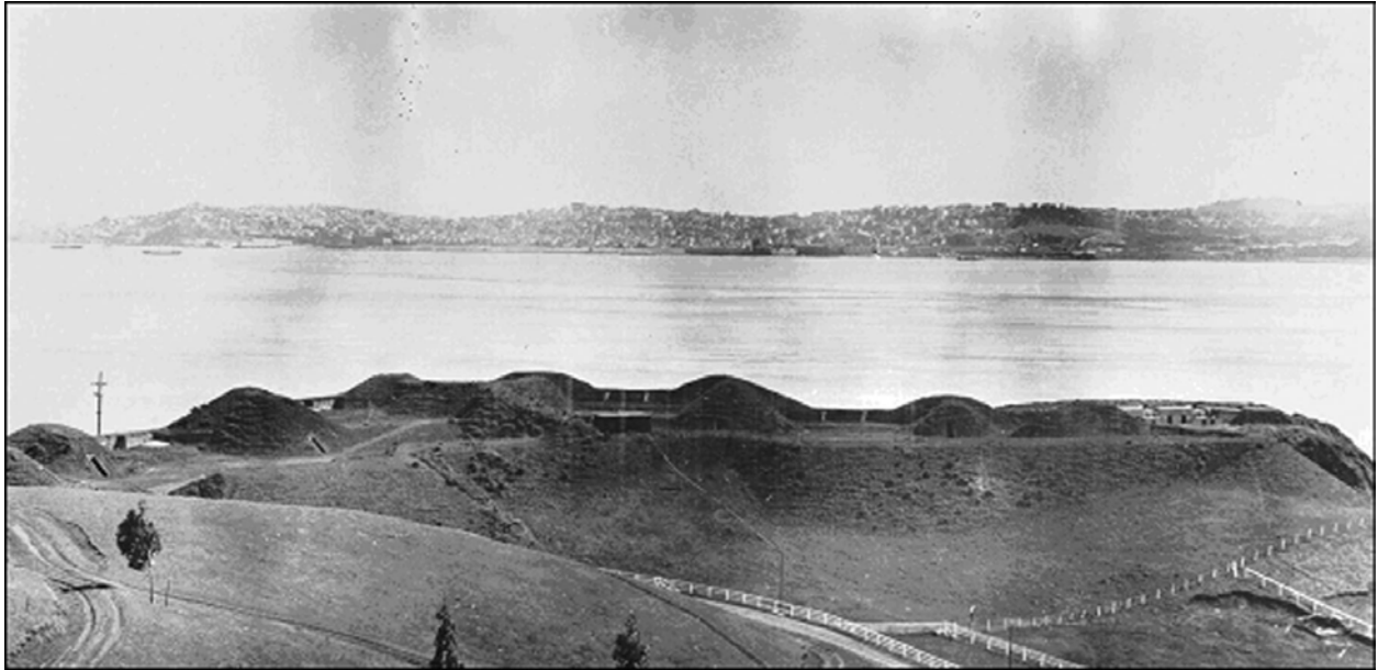
The silhouette of Cavallo Battery against the San Francisco Bay illustrates the extensive use of earth works in early battery construction. (Circa 1914, GGNRA collection)
