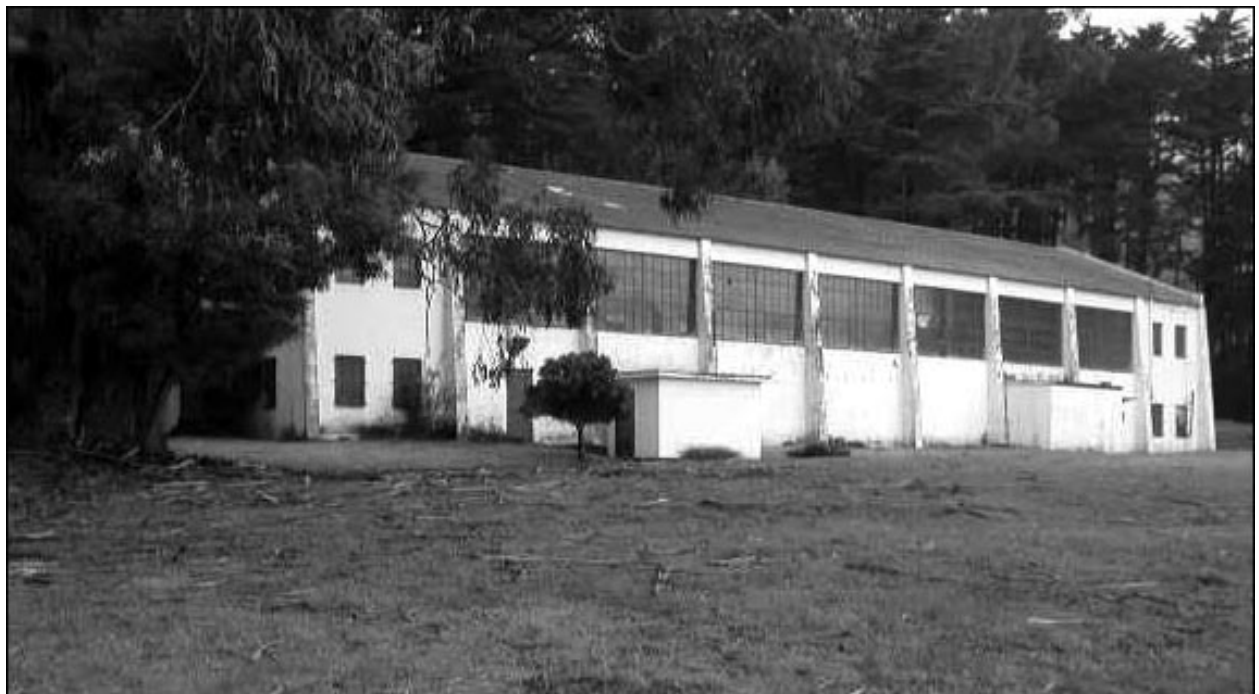
This warehouse on the south-west edge of the parade ground represents one of the utilitarian buildings on the site. (NPS, 2002)
