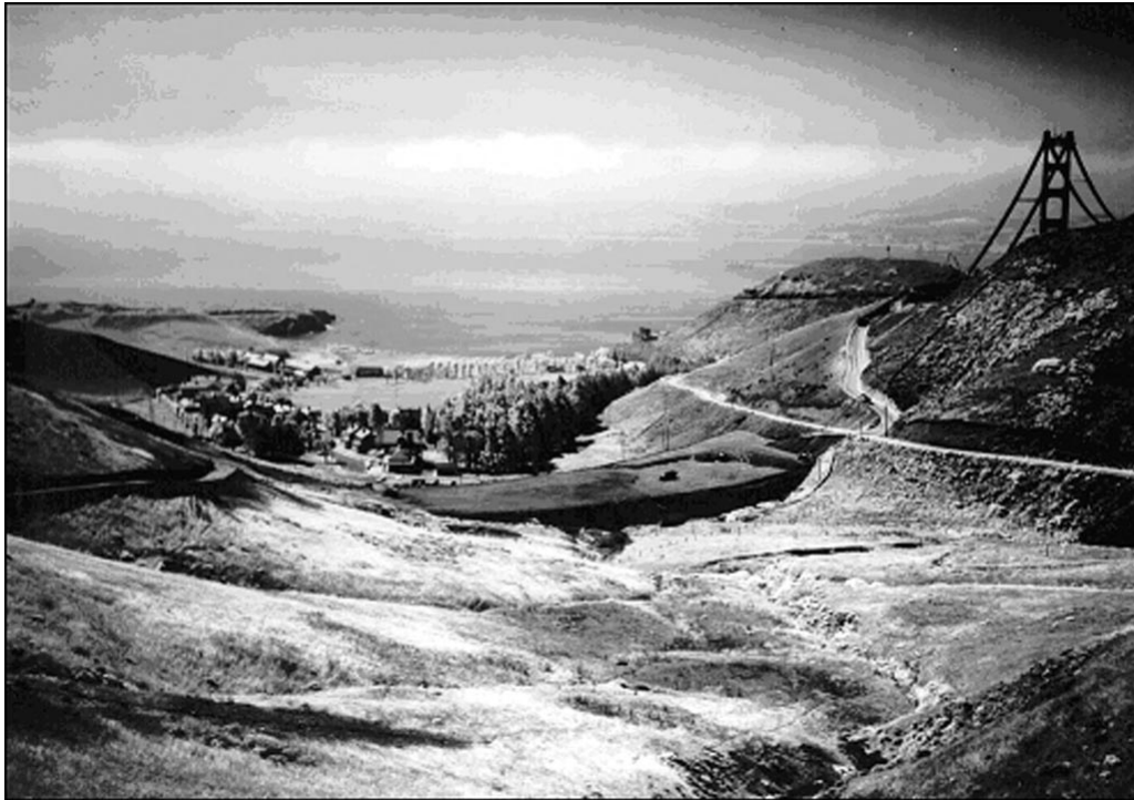
Construction of the Golden Gate Bridge and its approaches dramatically altered the Fort Baker landscape as well as the circulation system. Construction of the Sausalito Lateral is shown in the foreground. (Circa 1936, California Historical Society)
