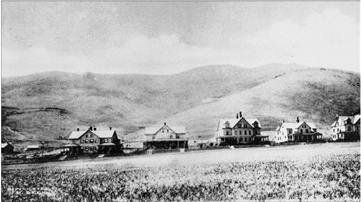
The buildings located on Murray Circle were constructed on a bench surrounding the Parade Ground. (Circa 1905, GGNRA collection)
