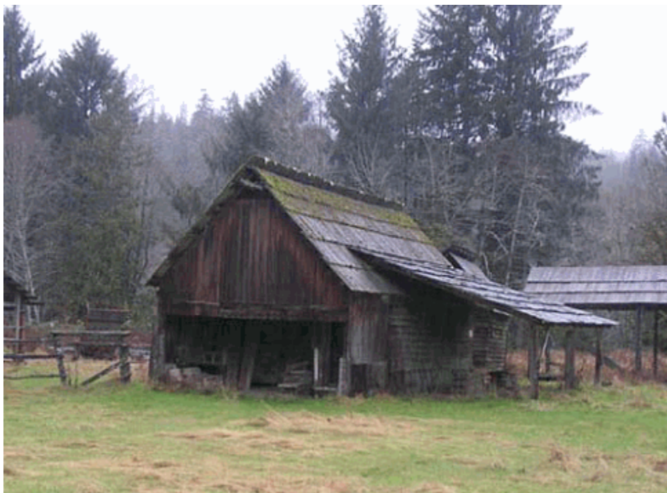
Root House (or Tack Shed) (contributing). (PWRO staff, 2006)
