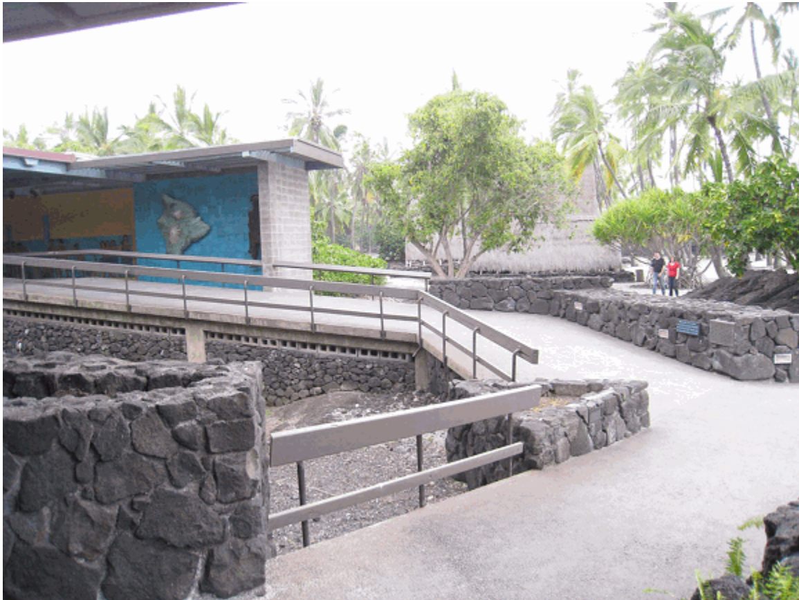
Circulation #2: Ramped concrete walkway adjacent to lanai (PWRO, May 2009).
