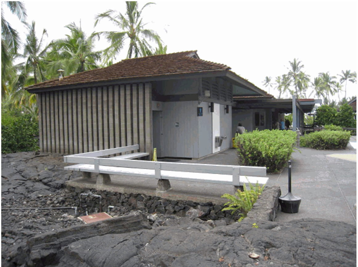
Buildings and Structures #1: Comfort Station, view looking southwest. (PWRO May 2009)
