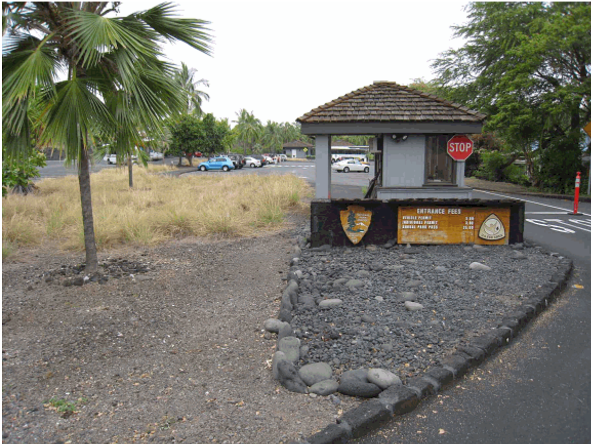
Buildings and Structures #4: Entrance kiosk, view looking south. (PWRO May 2009)
