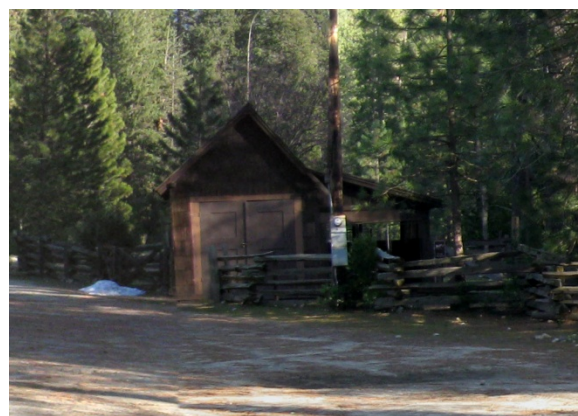
Army Tack Room (Contributing) LCS ID: 005799 Structure No: 4105
