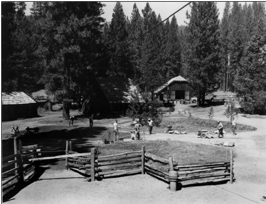
Historic photo taken from north end of the covered bridge looking north. Workers are installing soil cement pathways. Transplanted trees in grass “islands” are visible behind them. 1962 (YOSE archives, Box 183, Press Release Folder)
