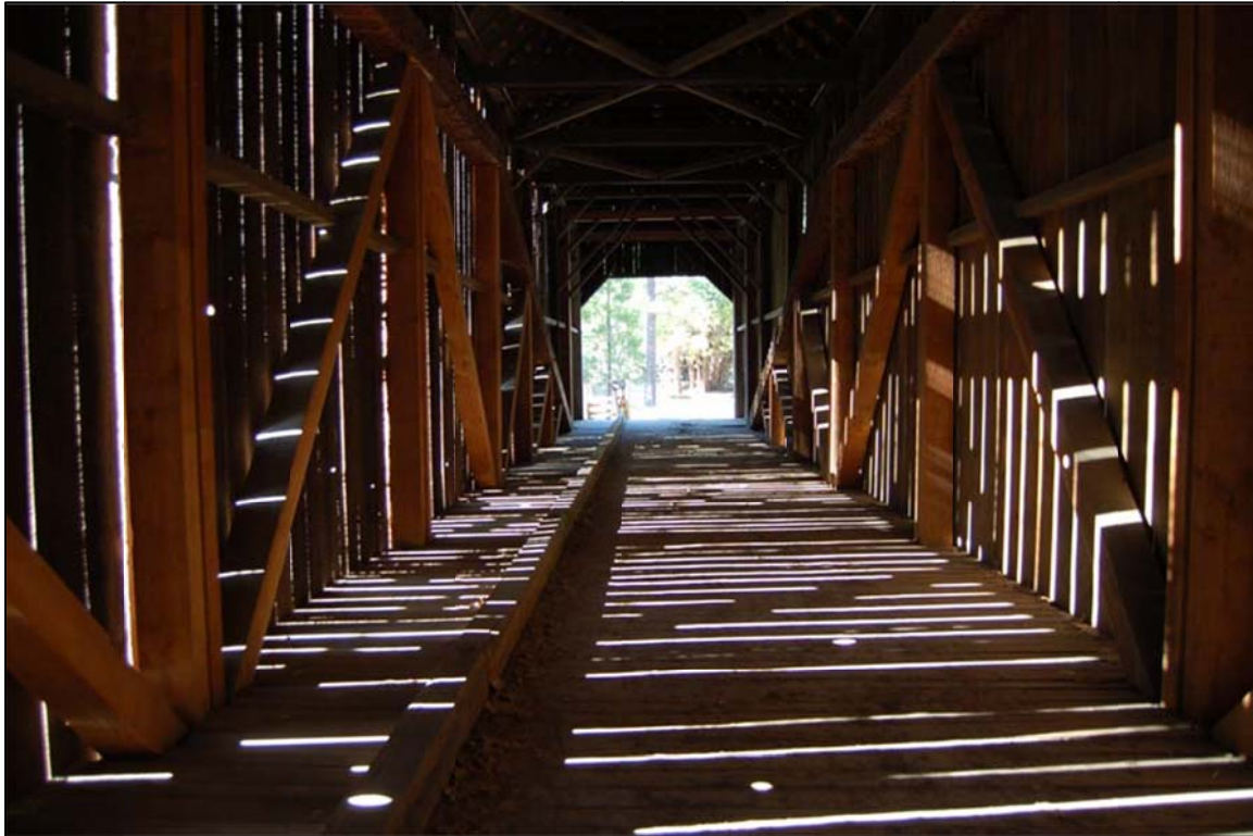
View through the covered bridge into the Pioneer Yosemite History Center. (YOSE 2010)
