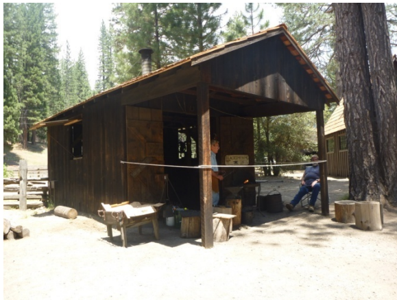
Blacksmith Shop (Non-Contributing/Managed as a Cultural Resource) LCS ID: 05805 Structure No: 4114
