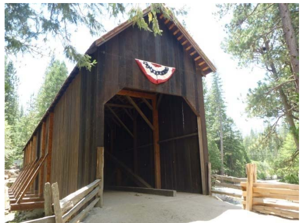
Wawona Covered Bridge (Contributing) LCS ID: 005838 Structure No: 4134
