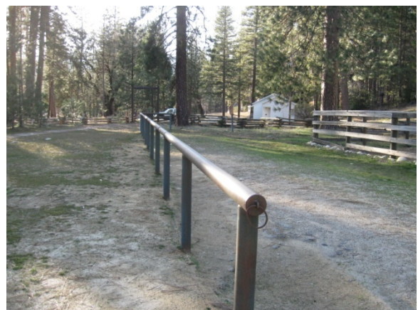
Hitching Posts (2 of 2) (Contributing)
