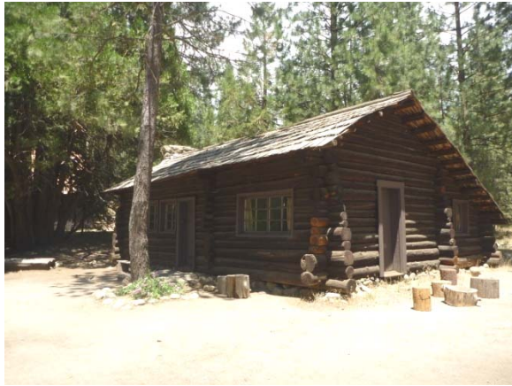
Crane Flat Ranger Cabin/Ranger Patrol Cabin (Contributing) LCS ID: 005800 Structure No: 4106
