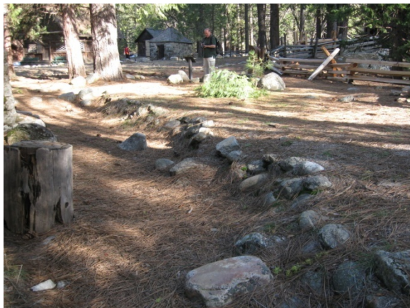
Retaining Walls (3 of 3) (Contributing)
