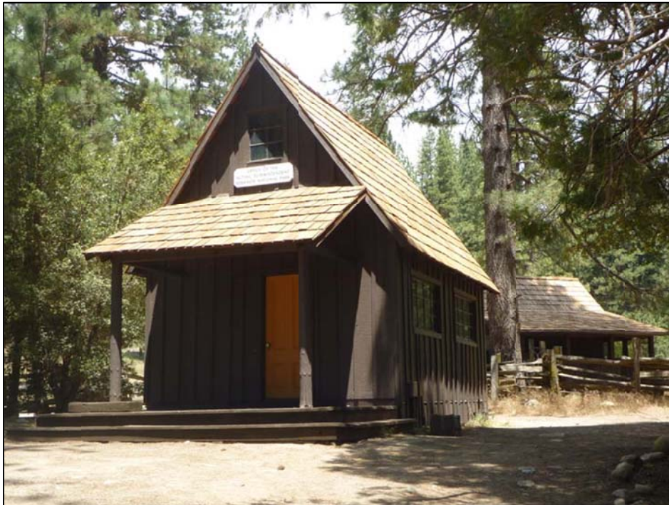
The Acting Superintendent's Headquarters in the foreground with the Army Tack Room visible in the rear. (YOSE 2010)
