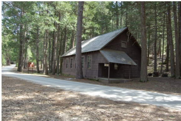
Chinese Laundry/Laundry/Carriage Shop (Contributing) LCS ID: TBD Structure No: 4132
