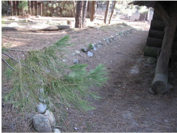
Retaining Walls (1 of 3) (Contributing)
