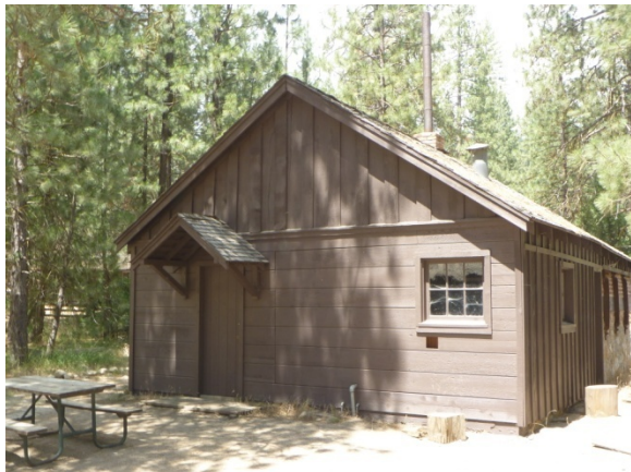
Degnan's Bakery (Non-Contributing/Managed as a Cultural Resource) LCS ID: 005784 Structure No: 4136
