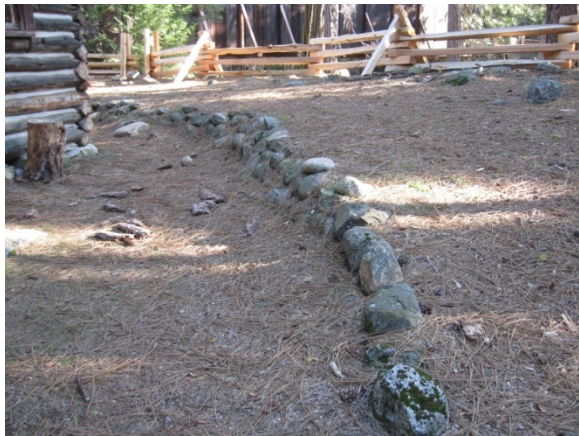
Retaining Walls (2 of 3) (Contributing)
