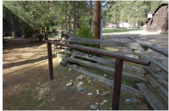
Hitching Posts (1 of 2) (Contributing)
