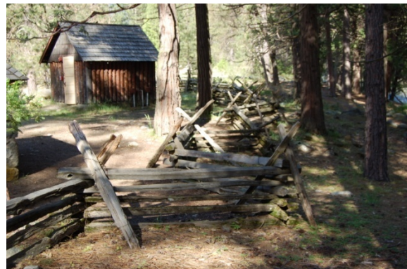
Wells Fargo Utility Building (Contributing) LCS ID: TBD Structure No: 4103
