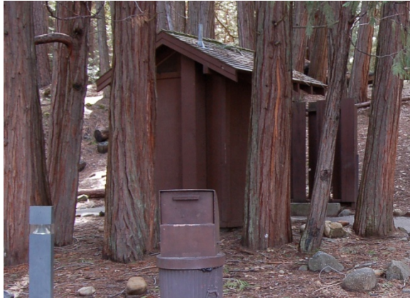
Pit Toilet/Pioneer Yosemite History Center Comfort Station (Non-Contributing) Structure No: 4108
