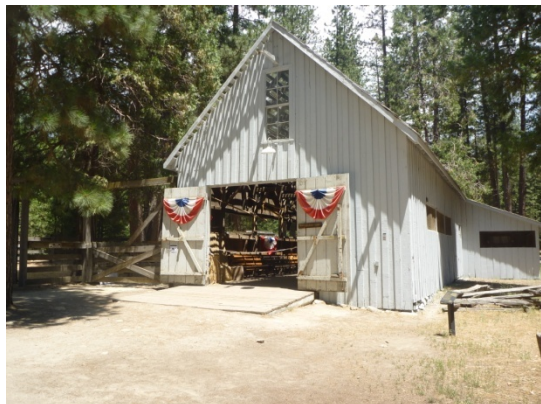
Wawona Grey Barn/ Washburn Barn (Contributing) LCS ID: 005796 Structure No: 4100
