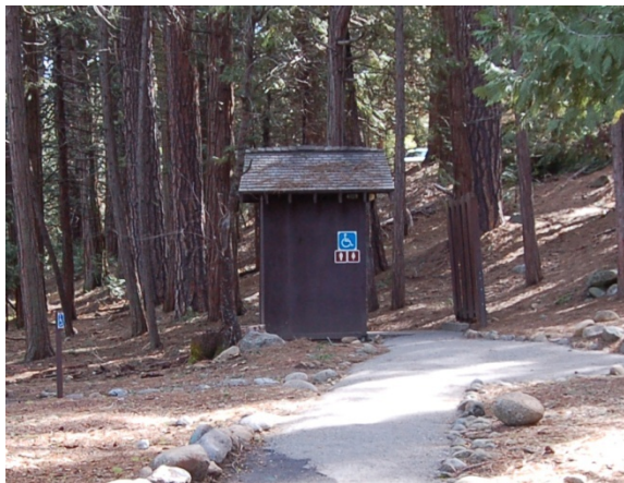
Pit Toilet/Pioneer Yosemite History Center Comfort Station (Non-Contributing) Structure No: 4109
