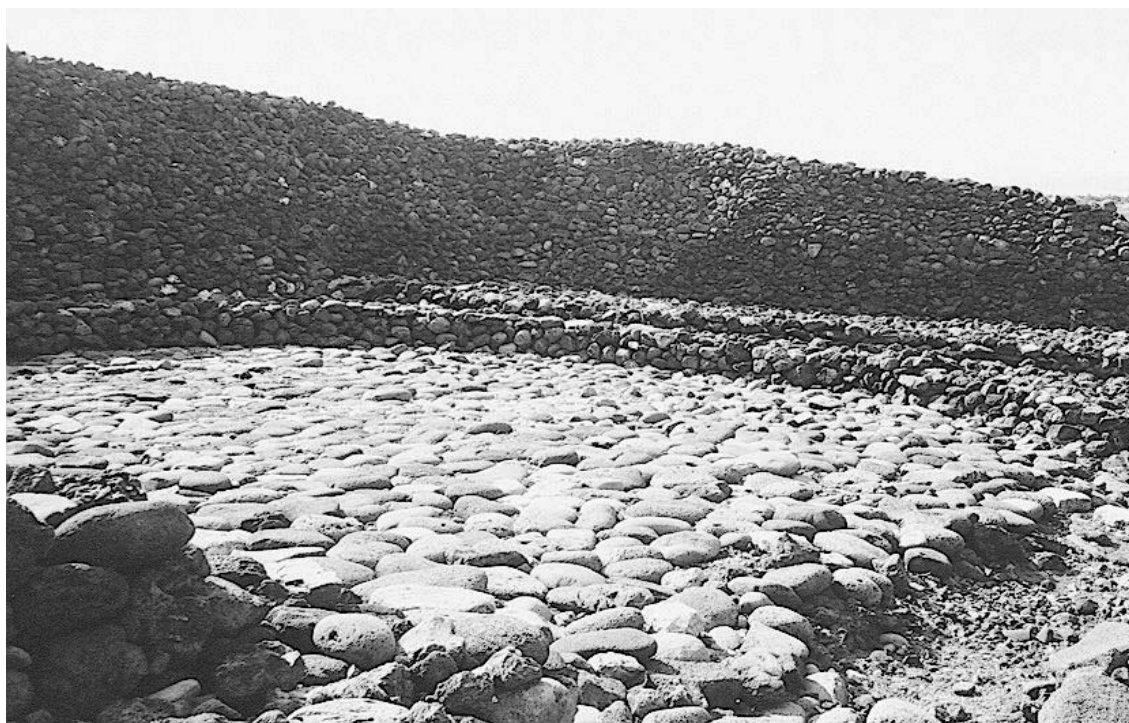
Contemporary photo of stonework on main platform within Pu'ukohola Heiau (CLI Team/PISO/2001).
