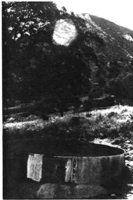
Coronado, Brown Allotment Spring, looking West. Drinking tank in foreground of photo is supplied by Brown Allotment Spring. Montezuma Peak is in the background of the photo. 2000 feet of pipe is used to convey water from the spring to this tank. This site is on Forest Service land and still in use.
