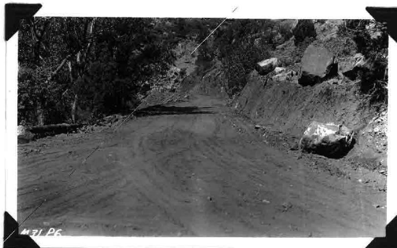
No. M31P6 Reconstructed road, - near pipe line.
