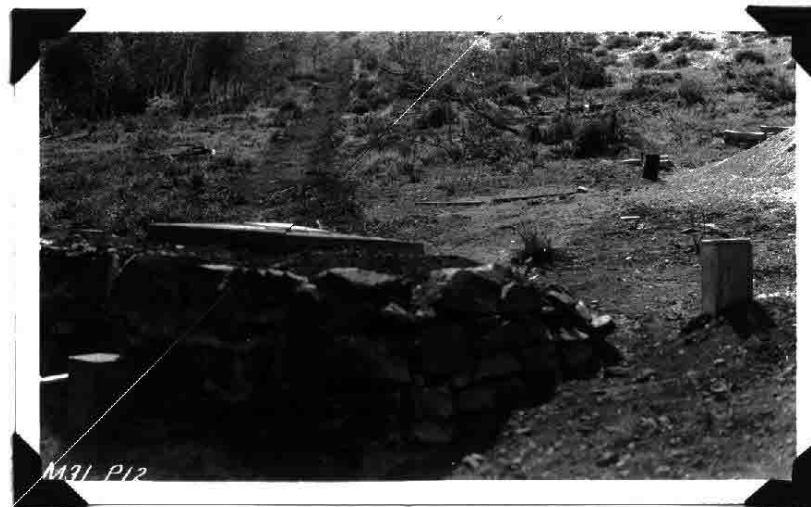
No. M31P12 Collection box. Note lines to springs.
