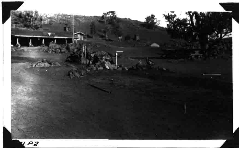
No. MS1P2 Camp Ground and Lodge - Note hydrants.
