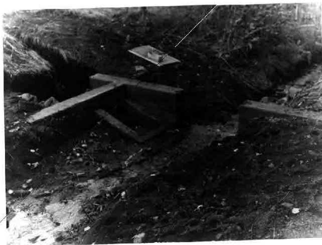
Water diversion structure Point "B" following stripping of forms. 9/24/62
