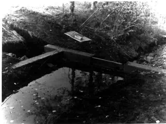
Water Diversion Point "B" Looking Downstream
