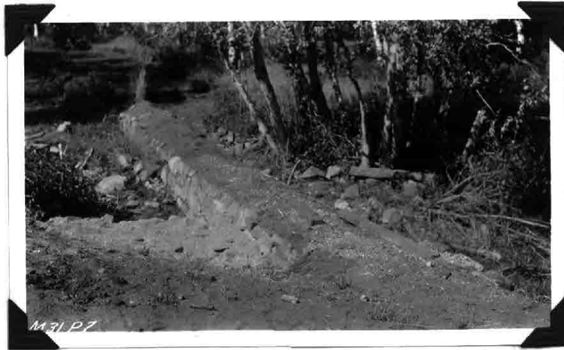
No. M31P7 Main supply line. Showing method of crossing creek.
