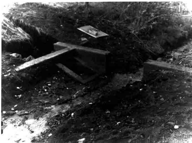
Water diversion structure Point "B" following stripping of forms. 9/24/62
