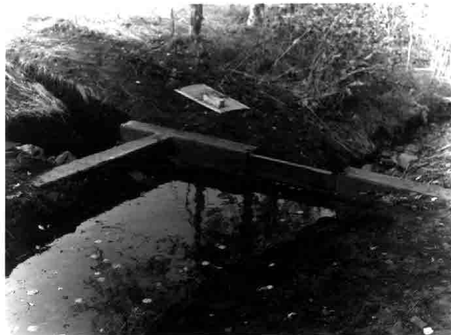
Water Diversion Point "B" Looking Downstream
