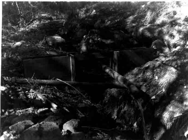
Forms set preparatory to pouring concrete for water diversion Point "B". 9/18/62
