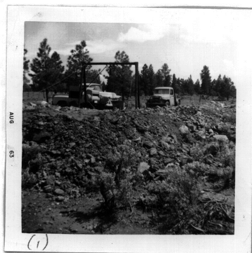
During digging operation - note material in foreground which was removed from well - note compressor and "A" frame and hoist used during digging operation.
