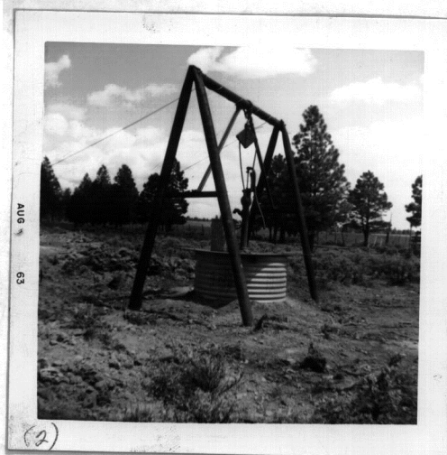
Completed well including hand pump installation - "A" frame has been removed and area cleaned since photo.
