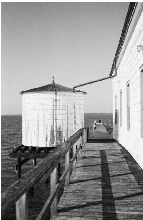
Fig. 36: View north of the cistern and walkway at the boathouse [Photo: NPS, 2000].
