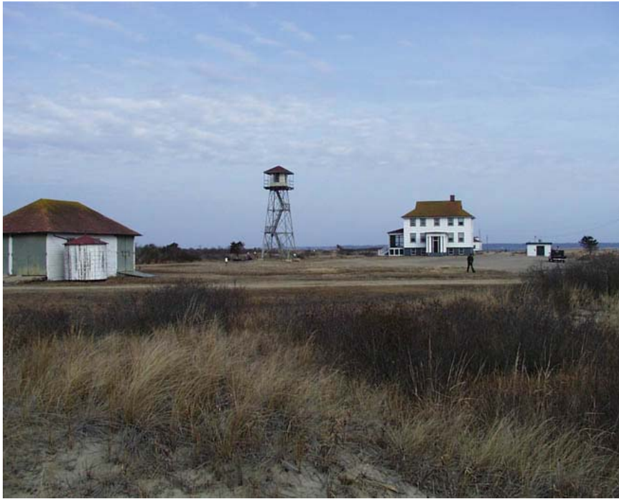
Fig. 25: View north showing the relationship of the structures in the core area [Photo: NPS, 2000].
