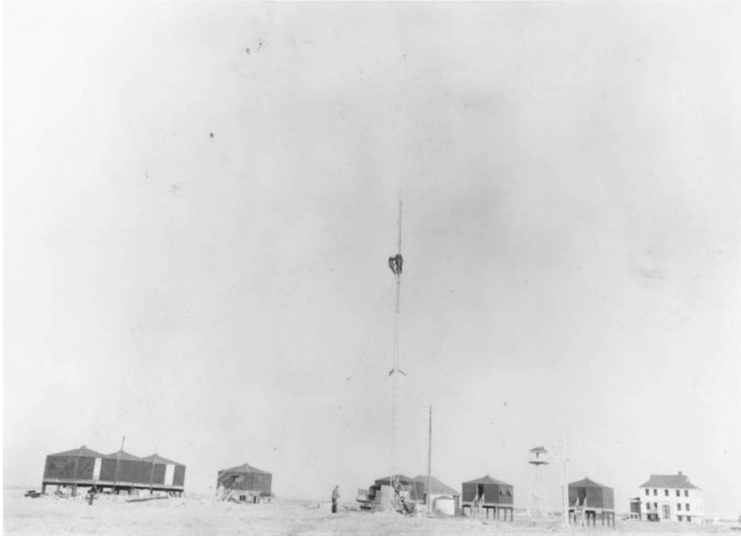
Fig. 15: The station complex in 1943 looking north. [U.S.C.G. archives, Washington D.C., Report on Construction of Radiator Tower, 1943].
