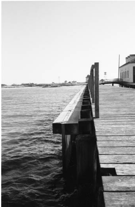
Fig. 37: View south of the remaining breakwater structure attached to the wharf [Photo: NPS, 2000].
