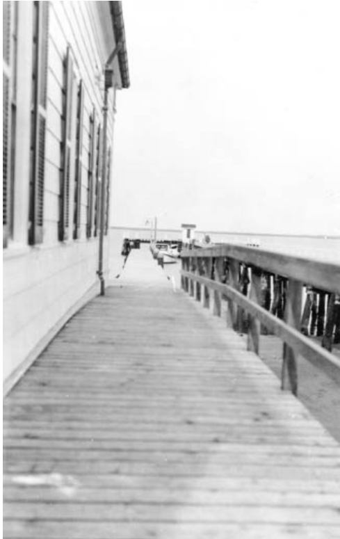
Fig. 14: Looking north from the boathouse walkway. Note the pump house [U.S.C.G. archives, Washington D.C., Feb. 16, 1939].
