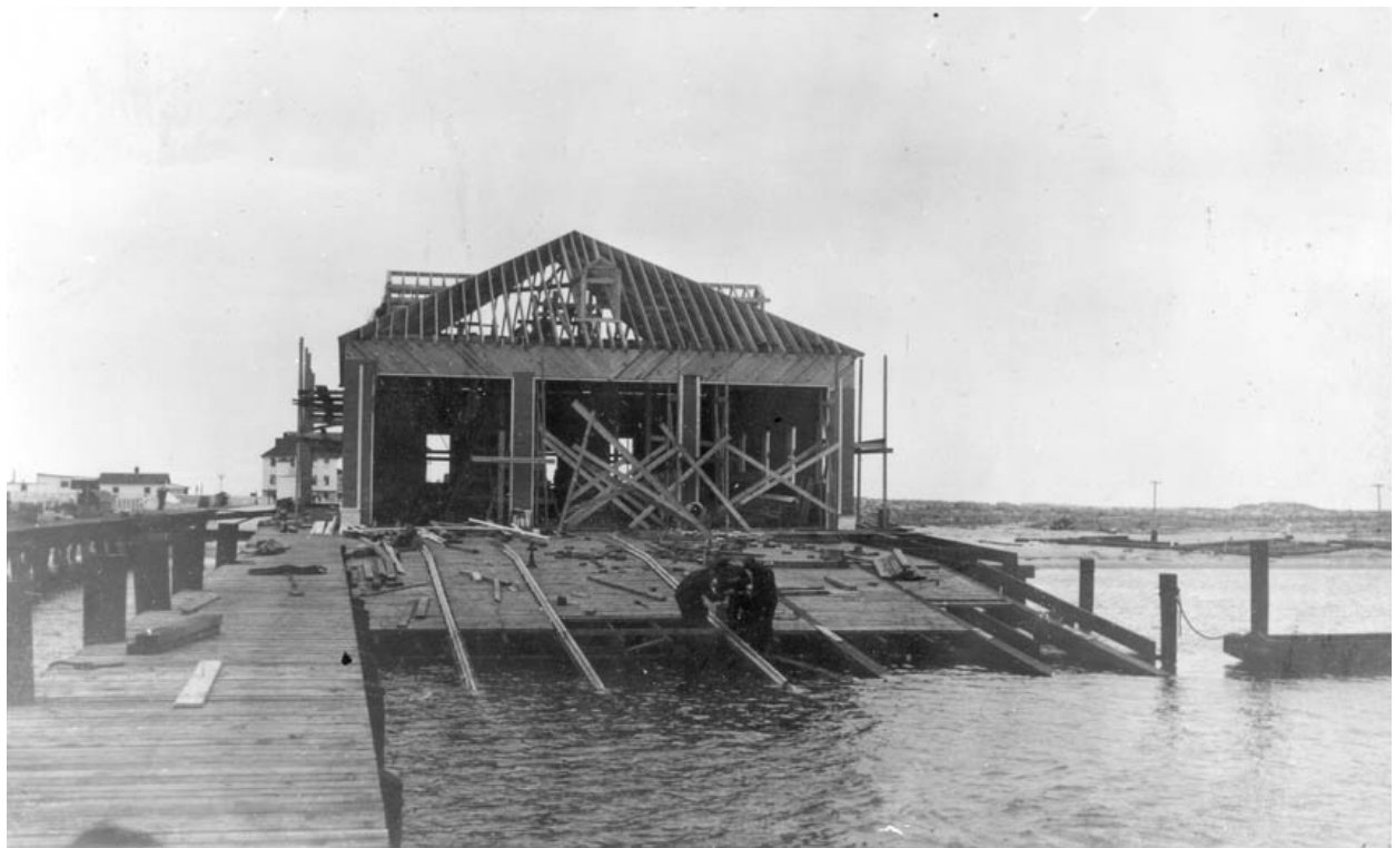
Fig. 13: The 1939 boathouse during construction, looking south [U.S.C.G. archives, Washington D.C., Dec. 1938].
