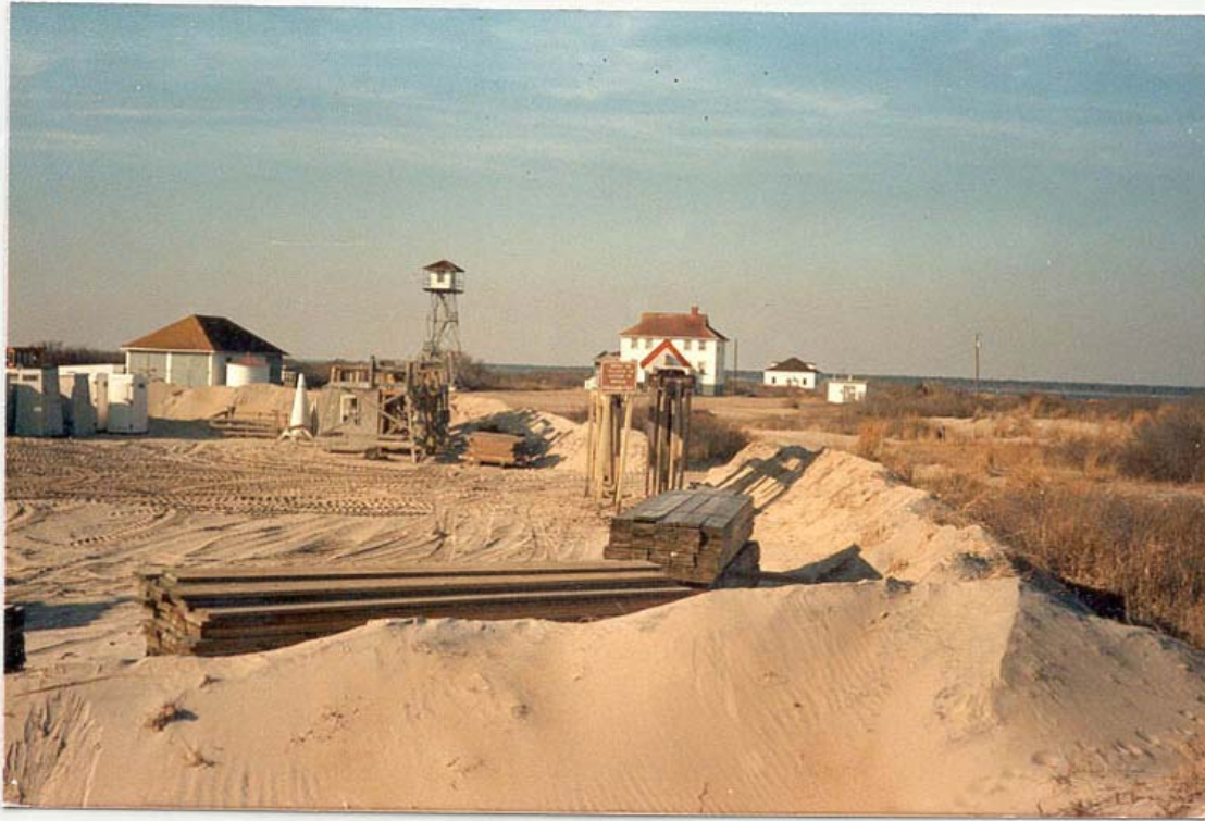
Fig. 21: View north from "maintenance yard" created by park staff in the 1980's (Photo courtesy of Mel Olsen, ASIS).
