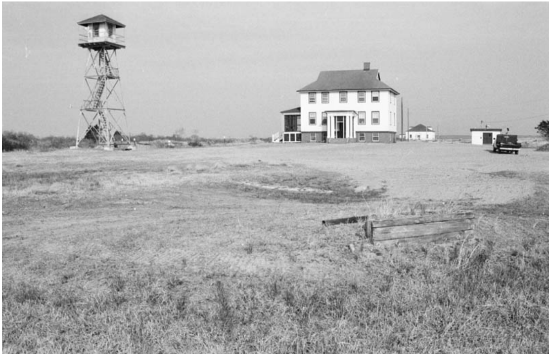
Fig. 28: View looking north of the station house on a high knoll with gentle slopes [Photo: NPS, 2000].
