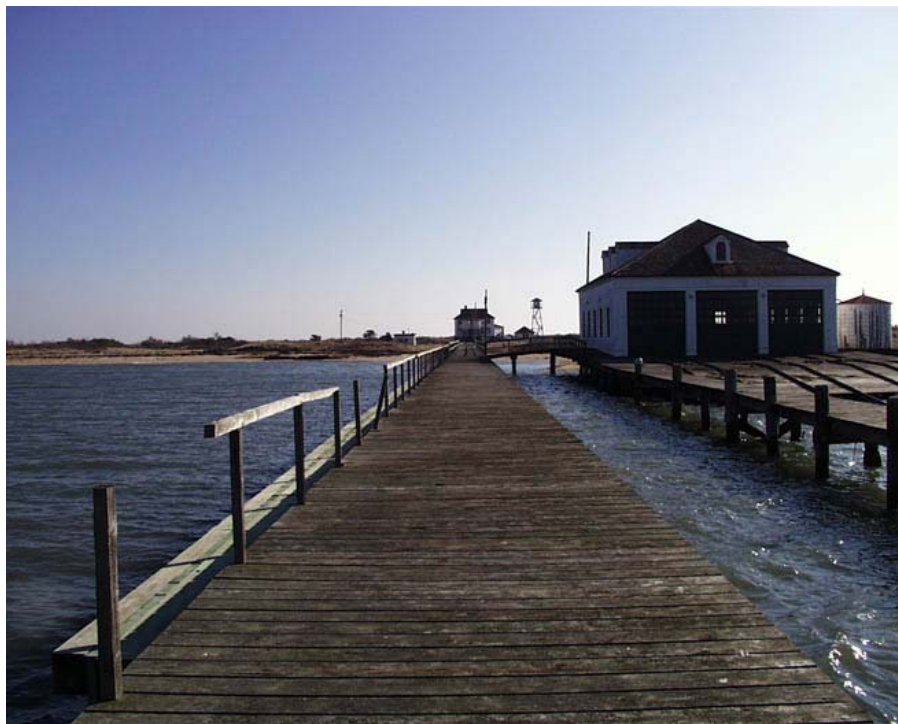
Fig. 24: View south from the wharf. Note the linear arrangement of the structures [Photo: NPS, 2000].
