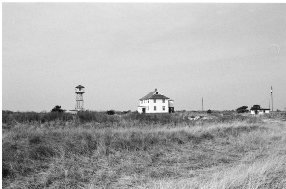
Fig. 31: View looking east from a road trace. Compare with Fig. 17 [Photo: J. Hau, NPS, 2000].
