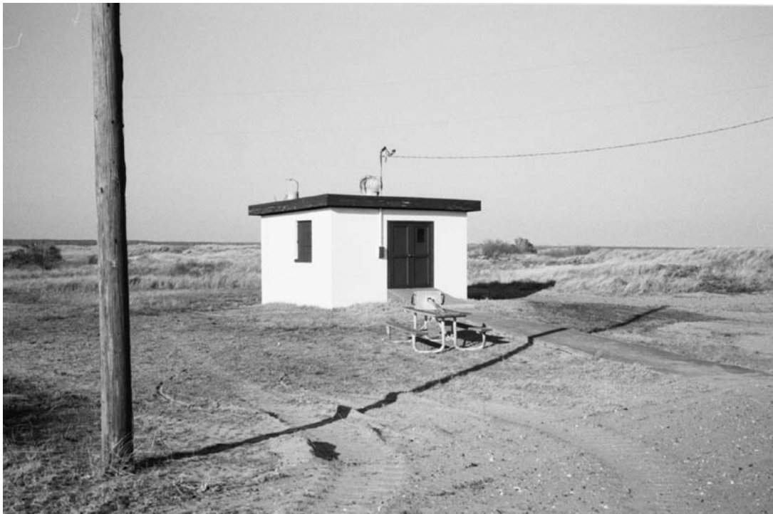
Fig. 38: View northeast of the 1959 generator house [Photo: NPS, 2000].
