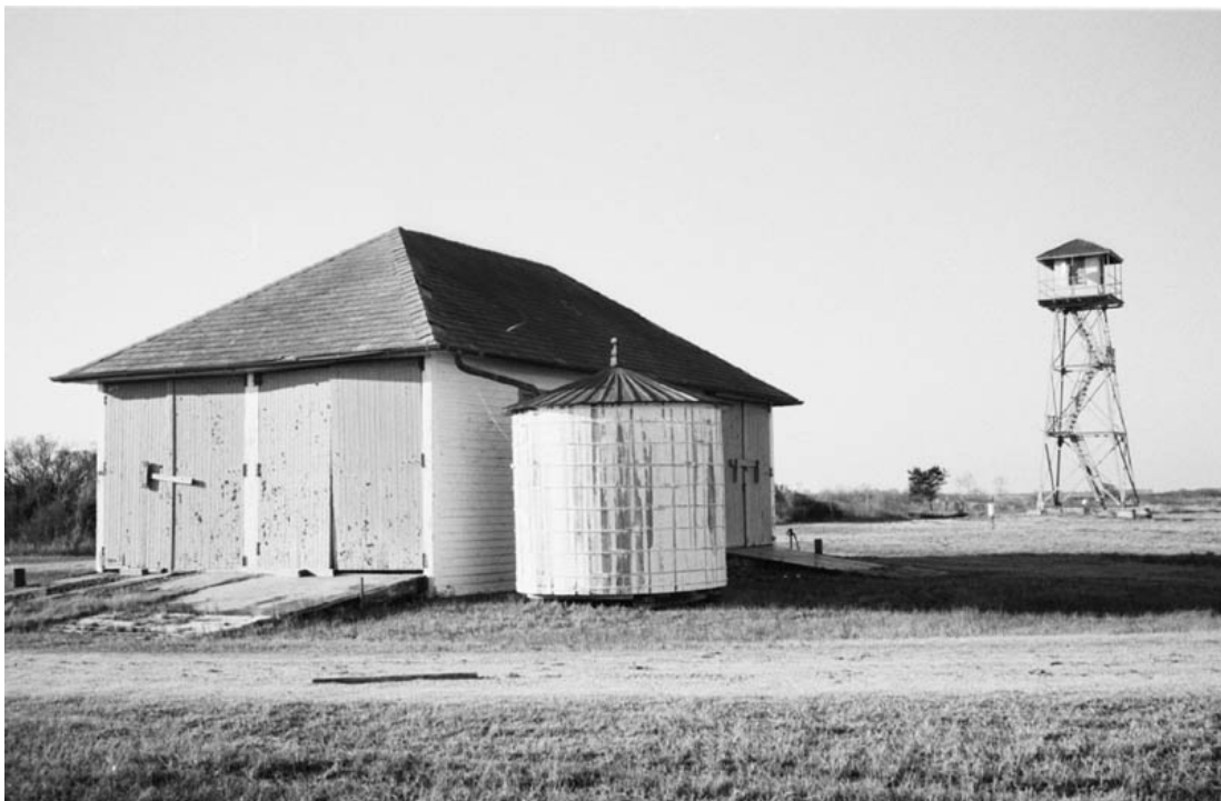
Fig. 34: View northwest of the garage [1922 boathouse] and cistern [Photo: NPS, 2000].
