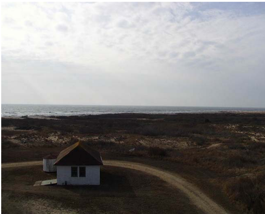
Fig. 41d: Views from the tower beginning north at the cove (a) and moving clockwise [Photo: NPS, 2000].
