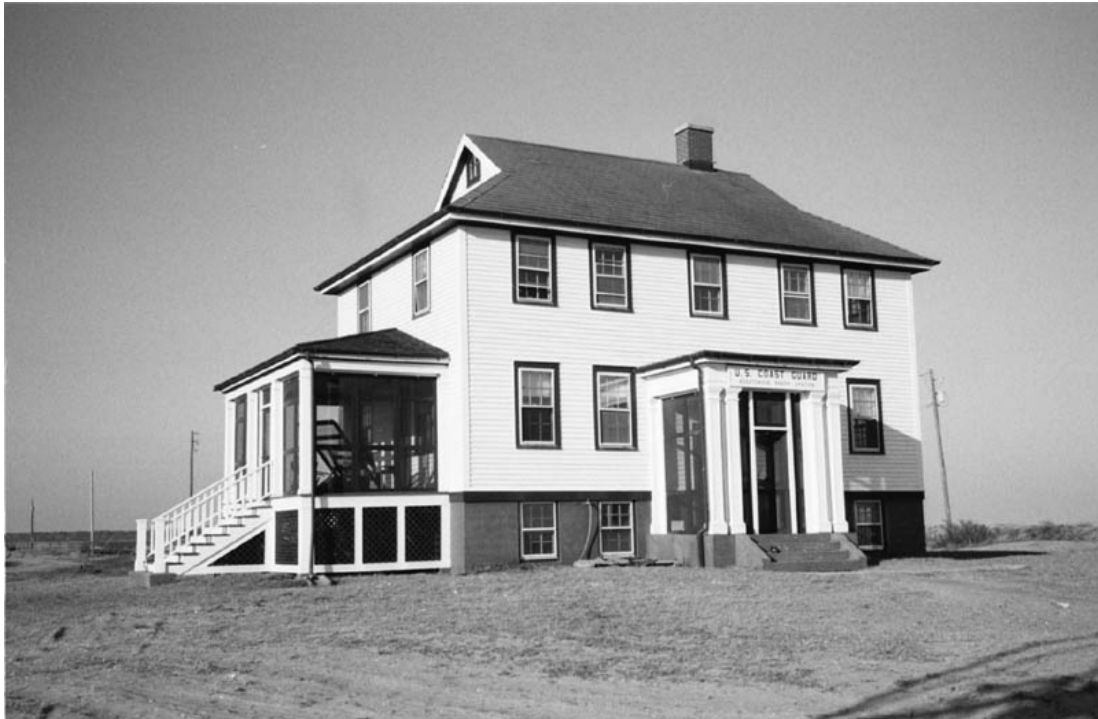
Fig. 33: 2000 view of Assateague Beach Station House looking Northeast [Photo: NPS, 2000].
