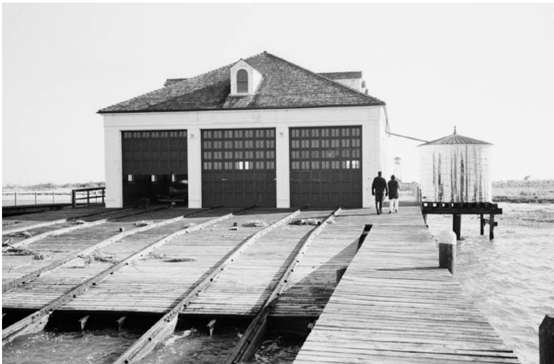
Fig. 26: The 1939 boathouse with a marine railway for launching boats and access to the station from the cove [Photo: NPS, 2000].
