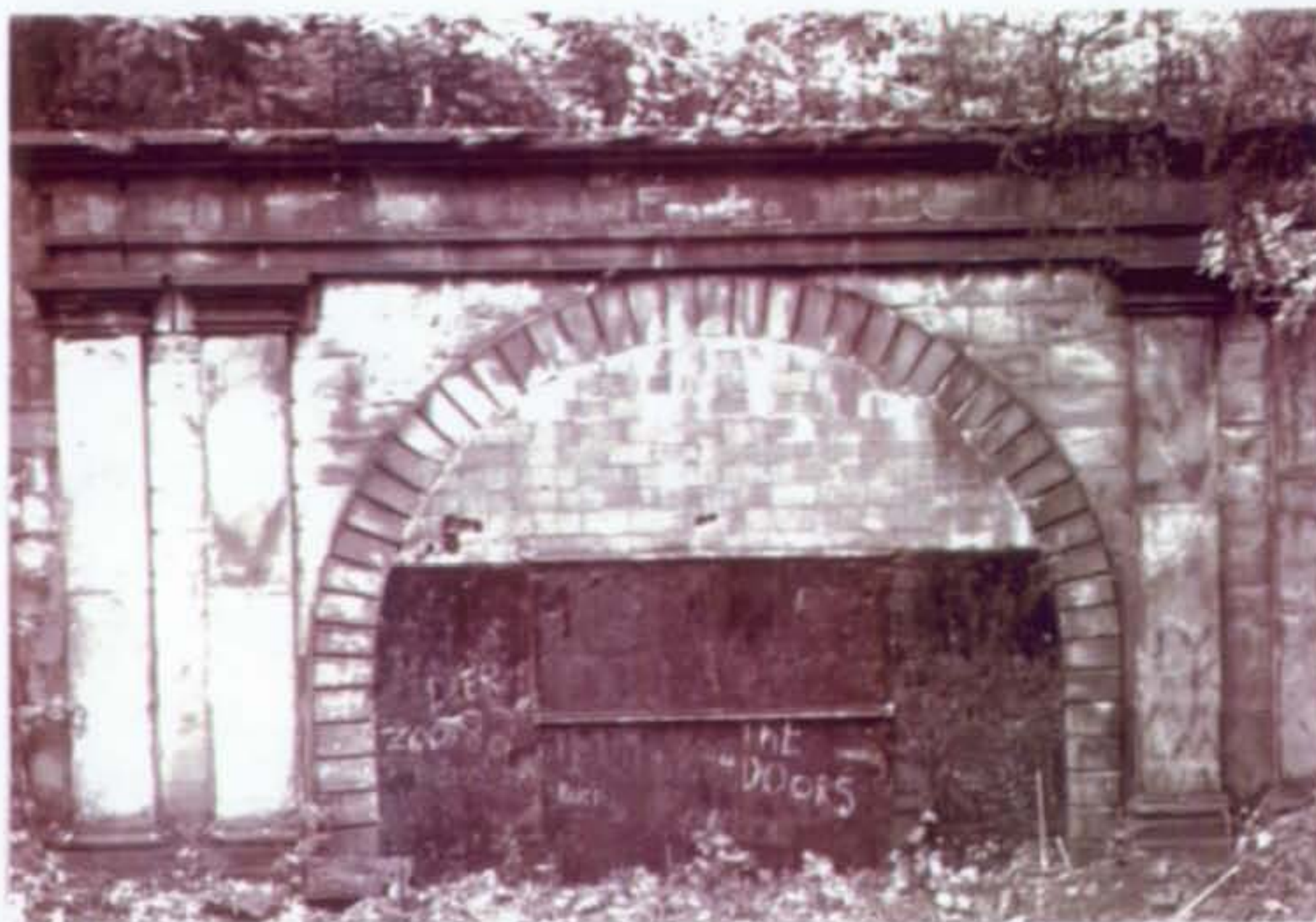
1990 Graffiti on parapet facing.
