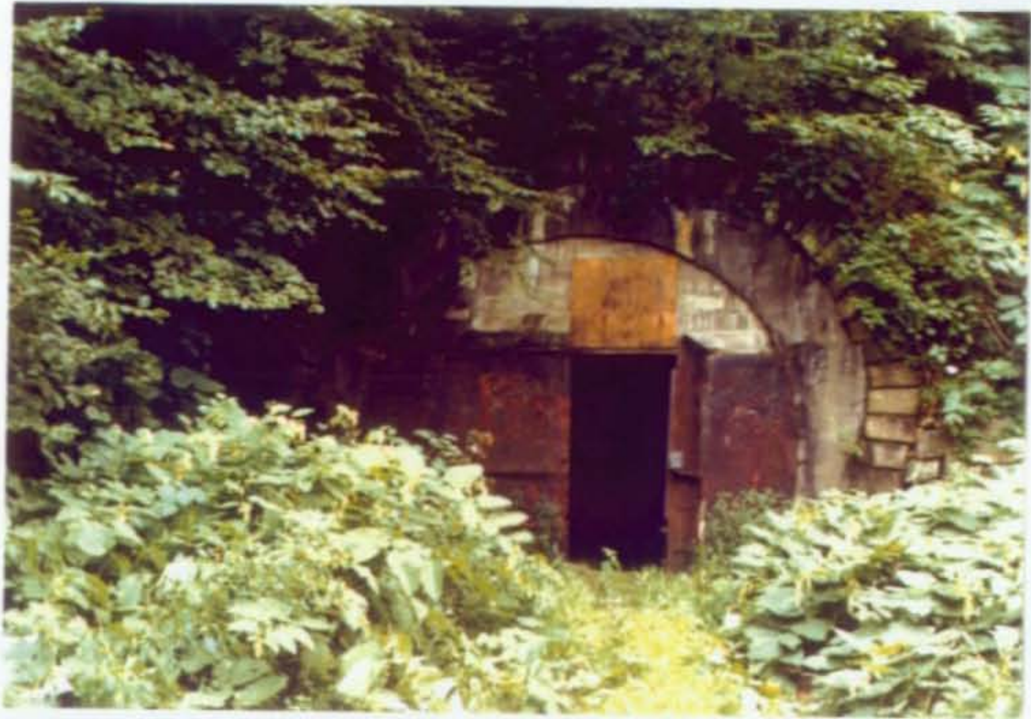
East End, 1990 Overgrown Entry. Concrete liner with concrete block infill.
