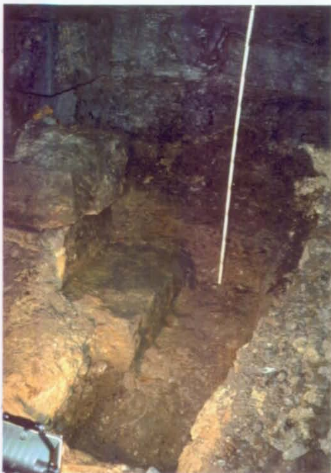
Test Pit No. 3: Foundation for east masonry lining at Sta. 7+46.
