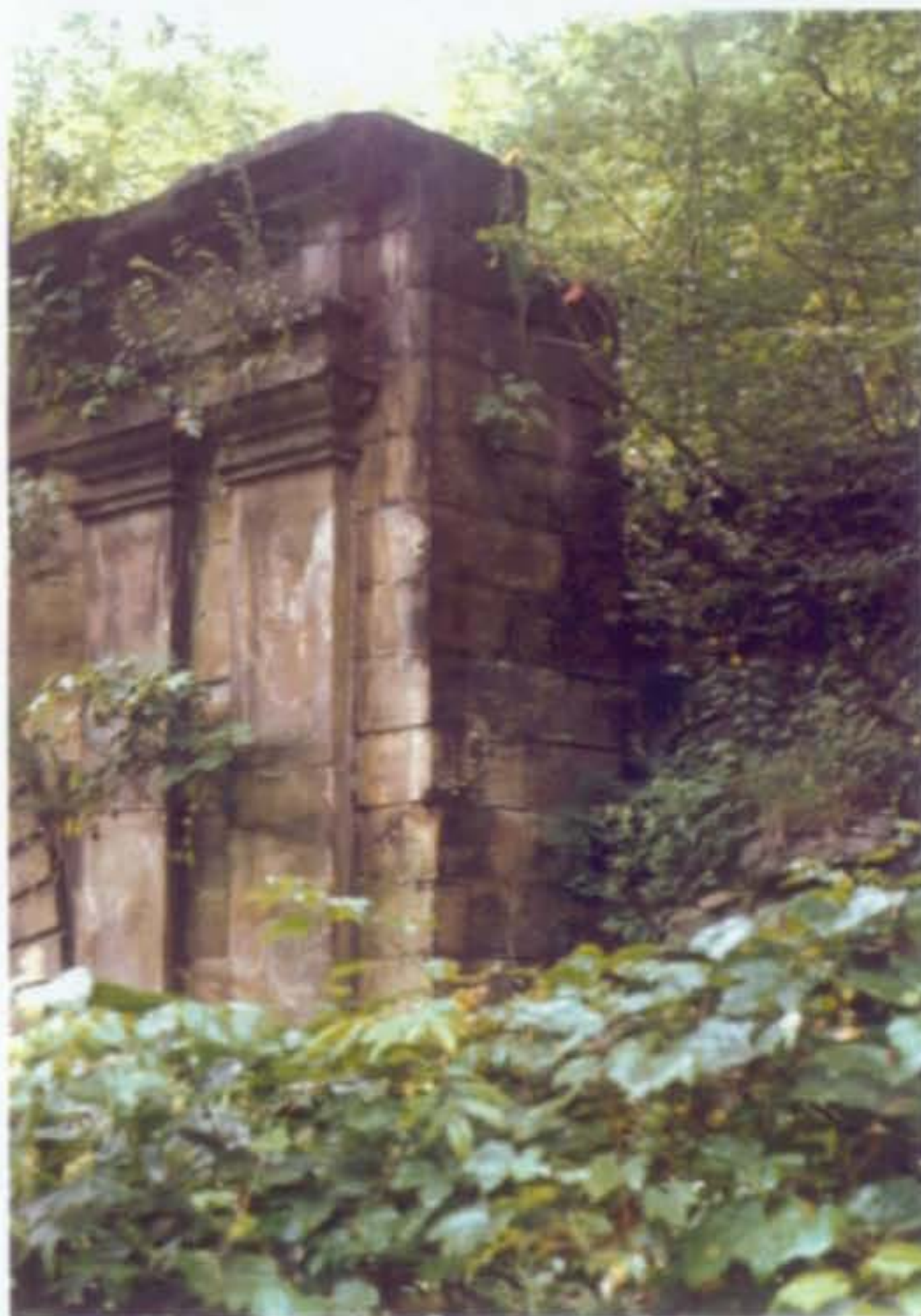
West End, 1990 Only portion of retaining wall remains. Grade is substantially higher than historically.
