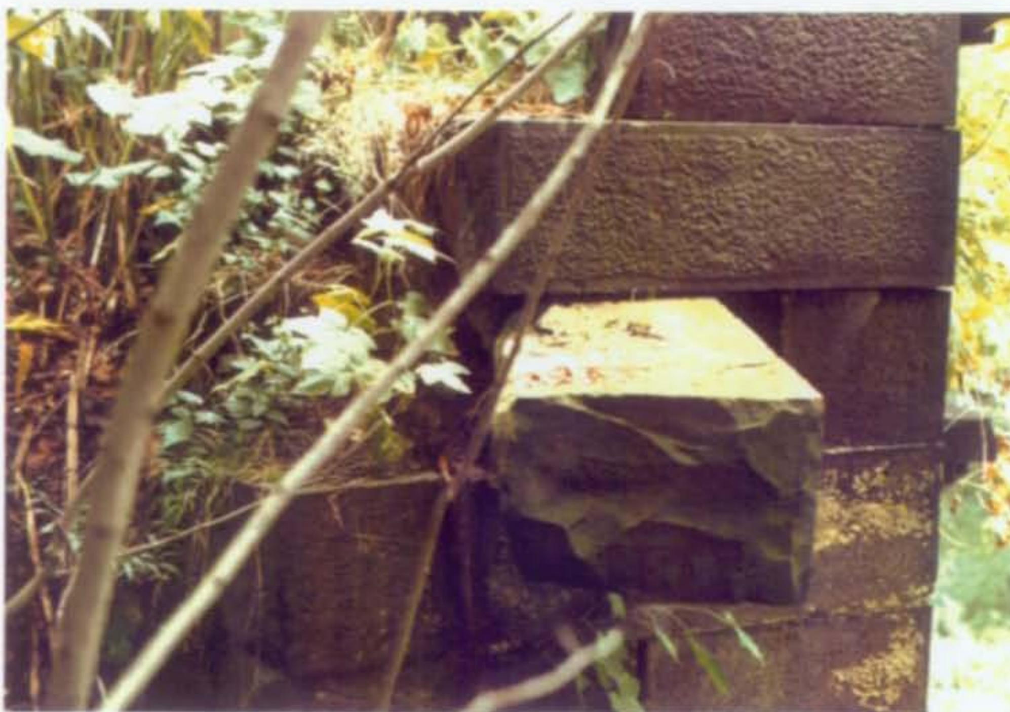
West End, 1990 Parapet stones, north end wall. Stone is rotated \pm 70^\circ from original. One stone has fallen and lies at facade base.
