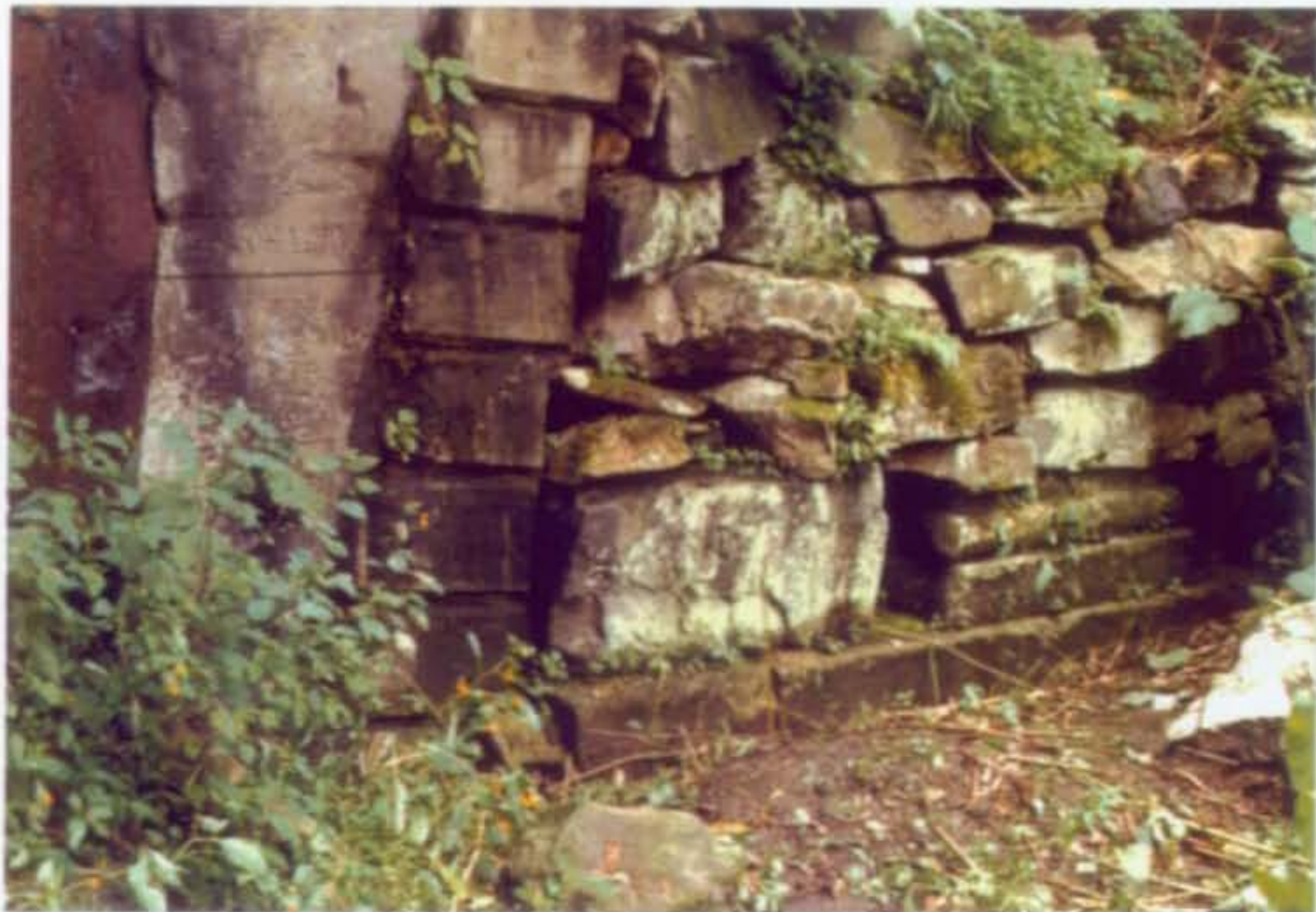
East End, 1990 Concrete lining conforms to dislodged stones. Rubble stone was used as retaining between arch stones and column base remnant.
