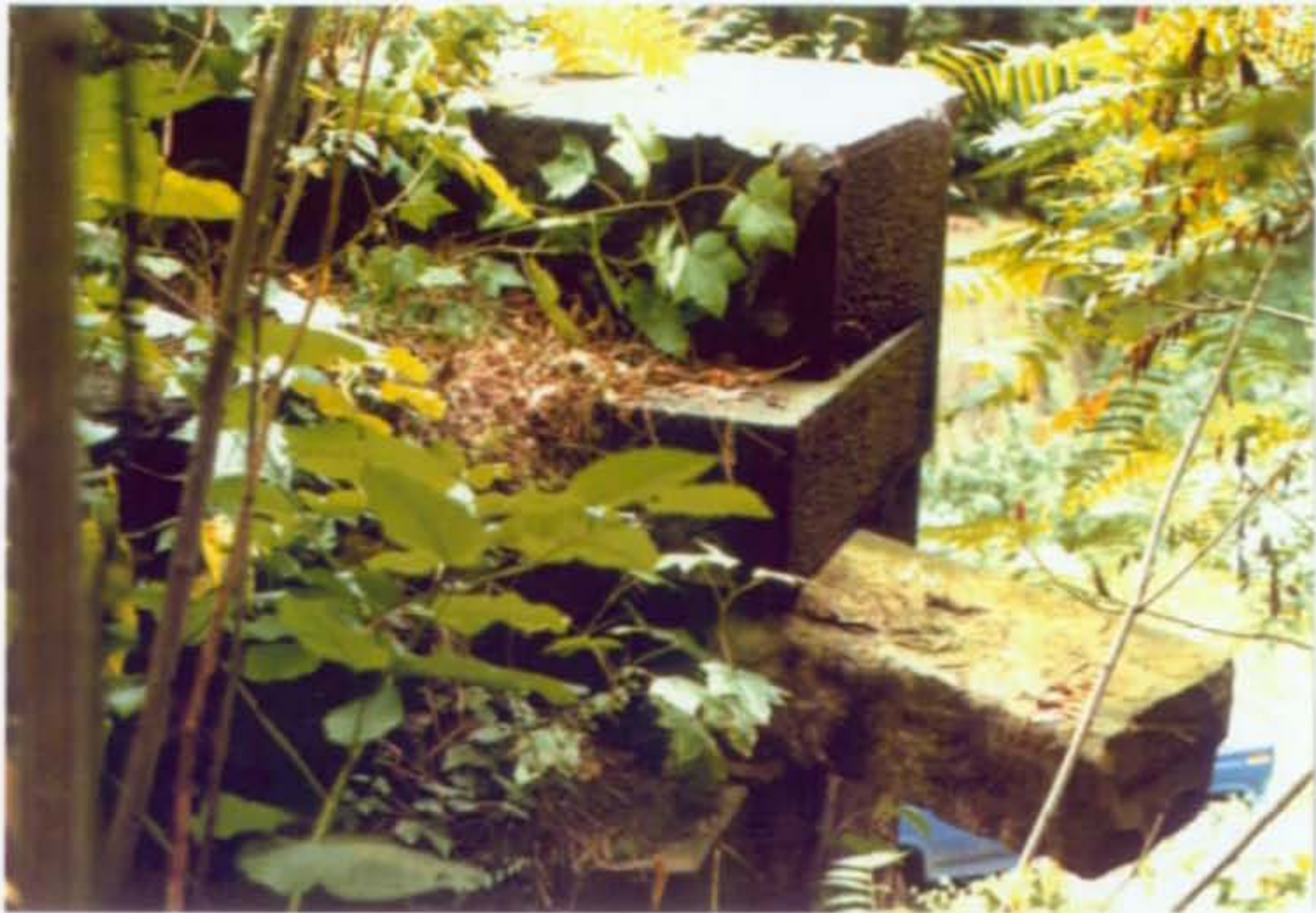
West End, 1990 View of rear of north end of parapet. Note rotated stone.
