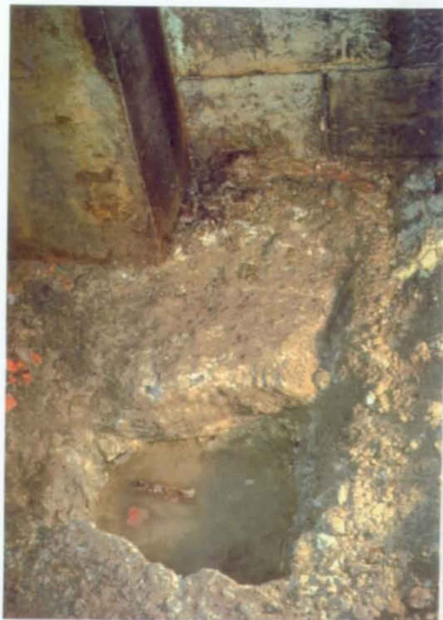
Test Pit No. 4: Foundation for concrete and masonry lining at Sta. 8+50.
