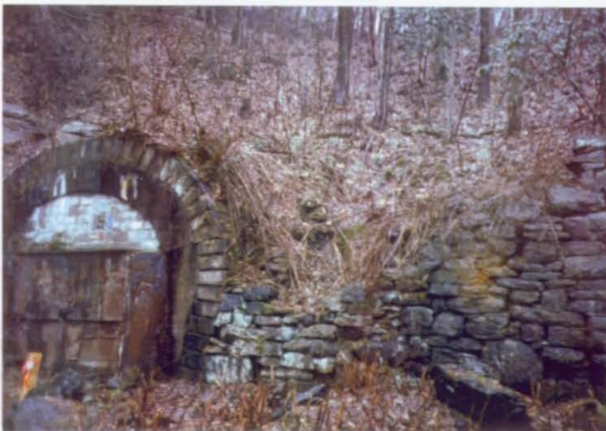
Eroded backfill slope to north of east portal. Note collapsed retaining wall, trees and remnant of original portal facade (center bottom of photo).
