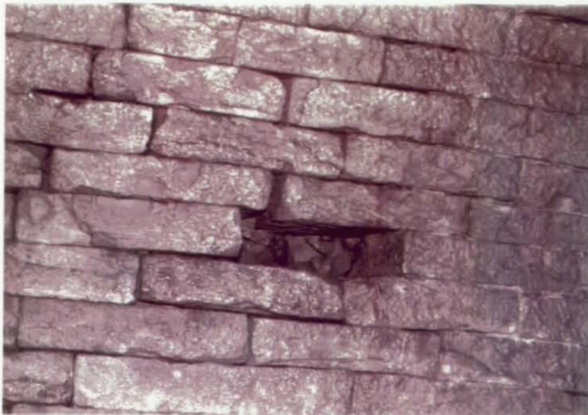
Missing arch crown block at Sta. 1+03. Note rubble backfill above masonry lining.
