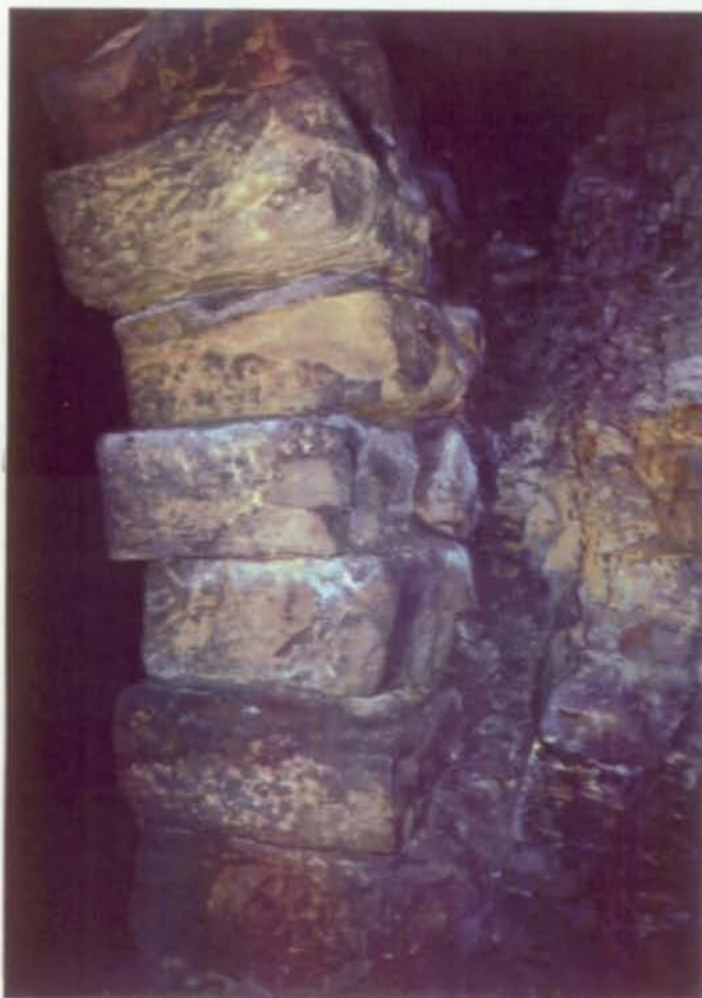
Masonry lining at Sta. 7+50. Note annular space between masonry and rock wall.
