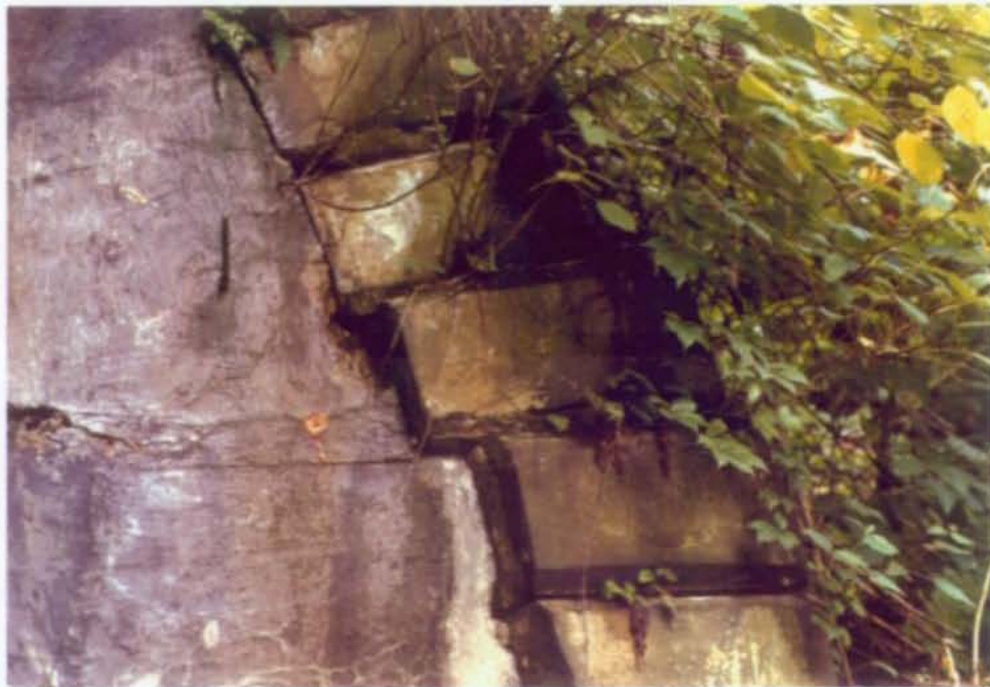
East End, 1990 Dislodged arch stones at north side. Stones have moved slightly from concrete lining indicating continued failure.
