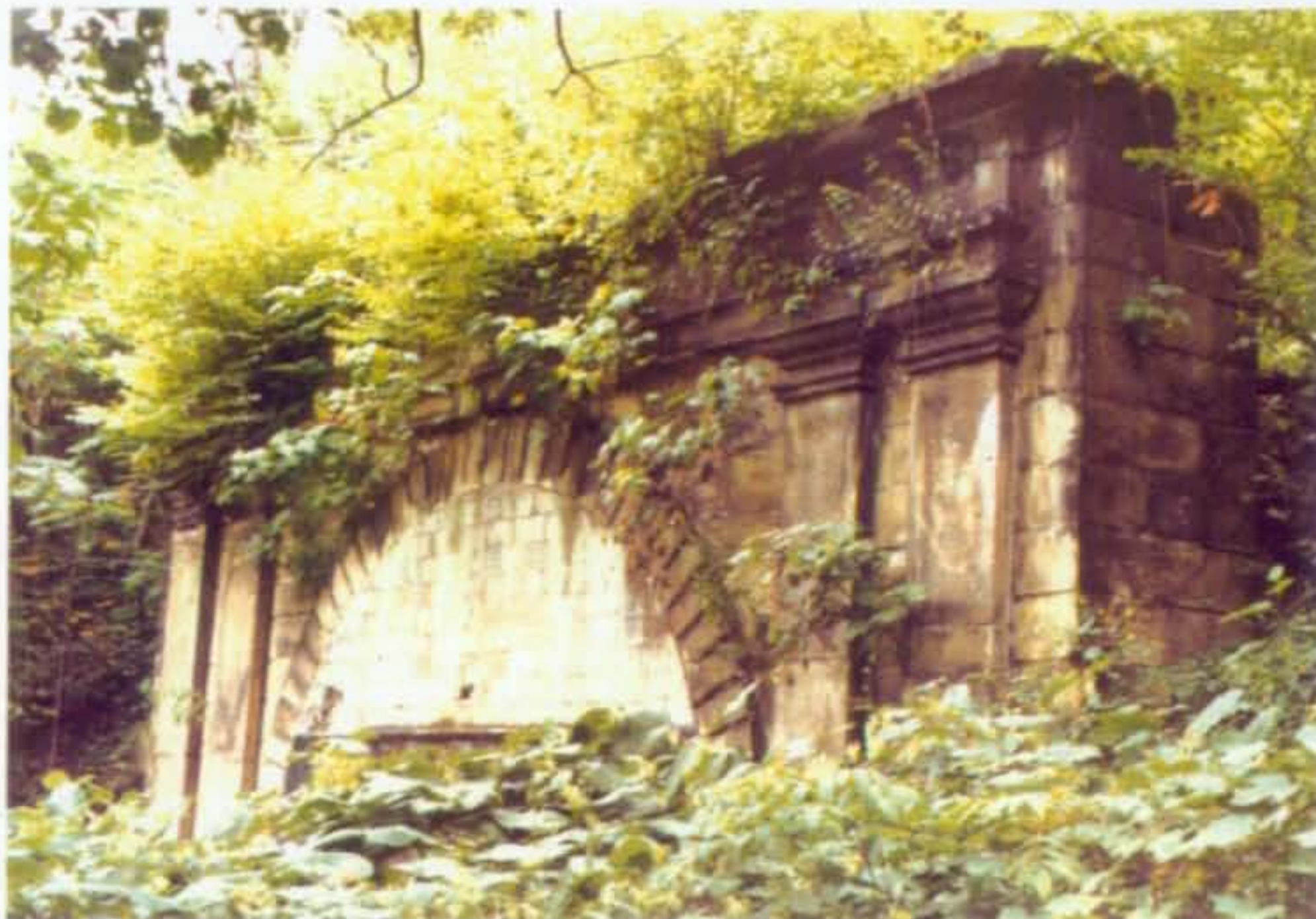
West End, 1990 View from southwest. Retaining wall less than half original height. Plant growth aids deterioration.
