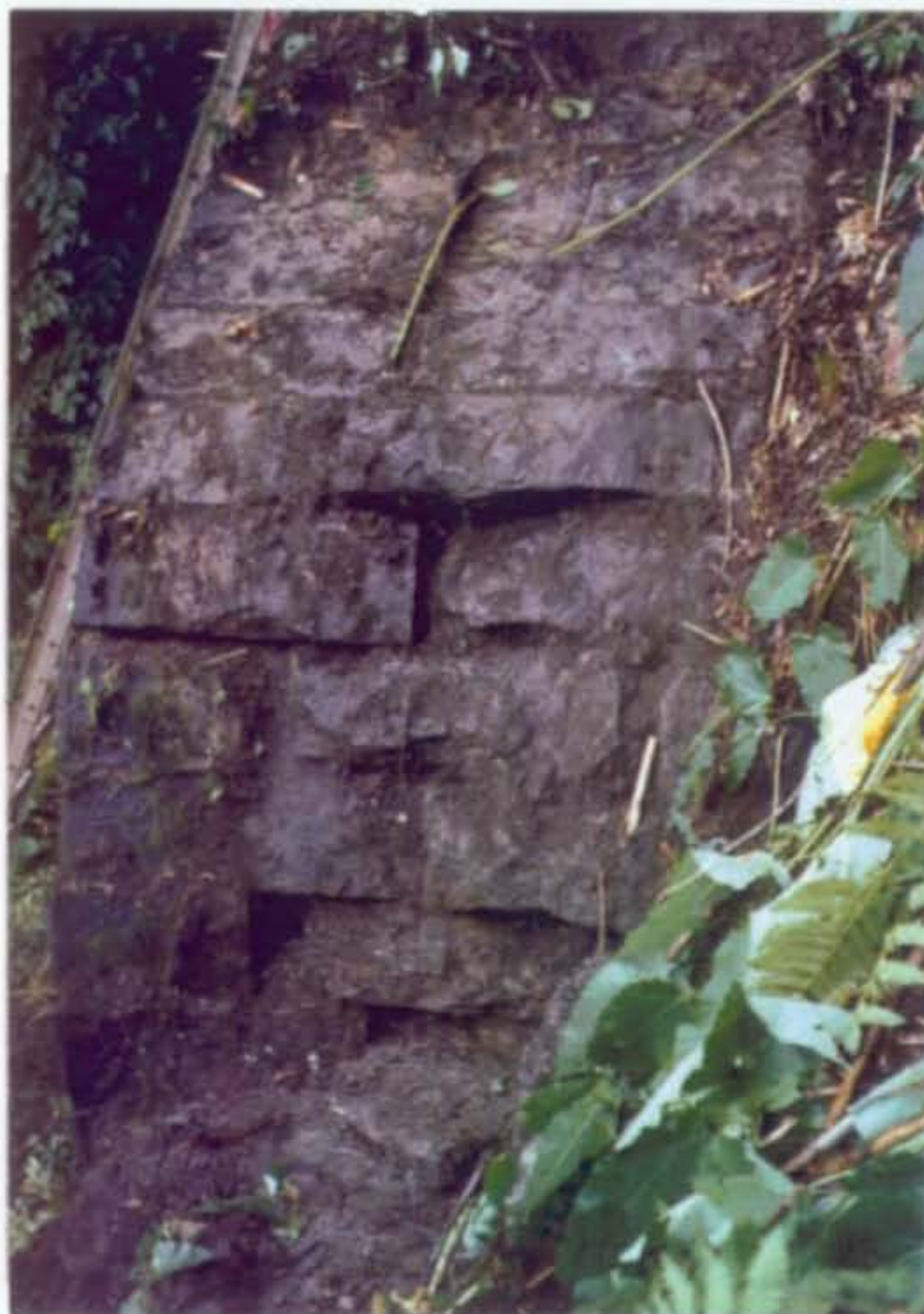
Test Pit No. 5: Foundation for west portal facade at Sta. 0+00.
