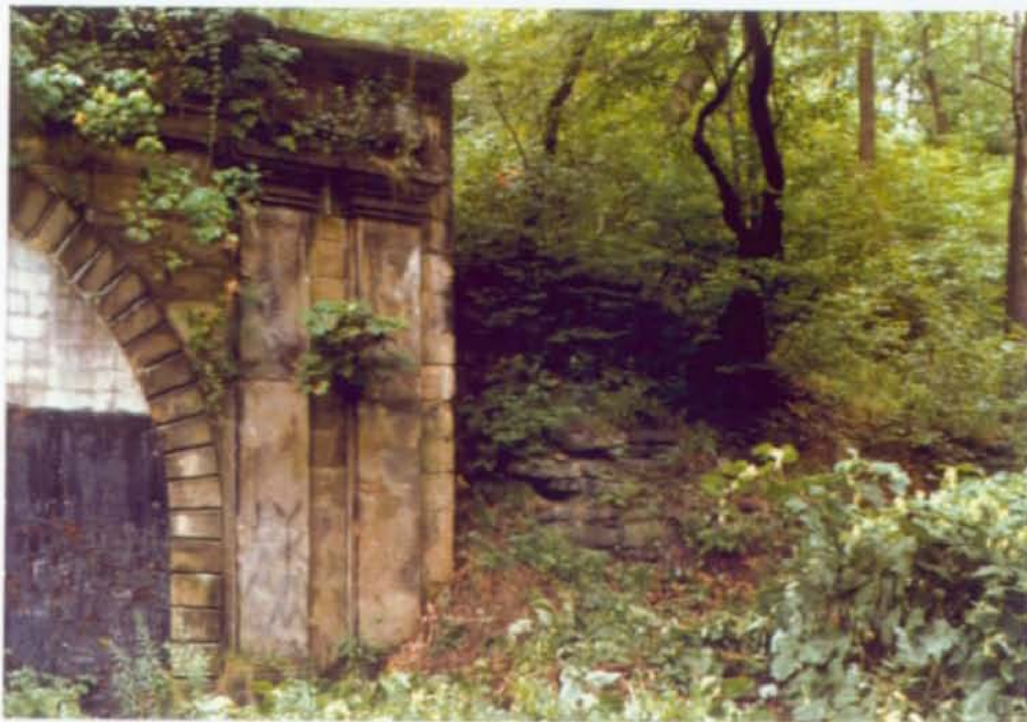
West End, 1990 Only portion of retaining wall remains. Grade is substantially higher than historically.
