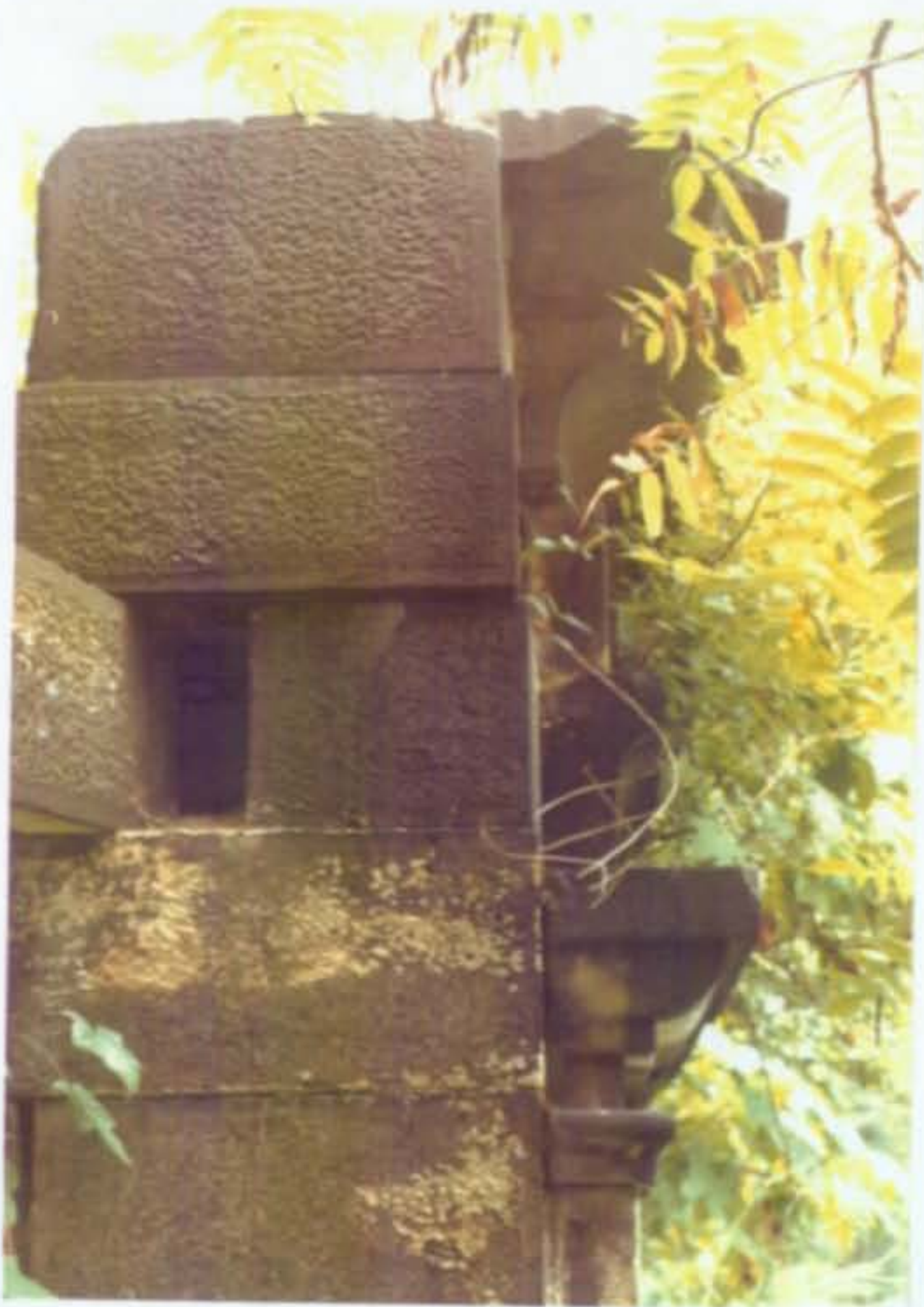
West End, 1990 Elevation of north end. Note pebbled texture and stone tooling.
