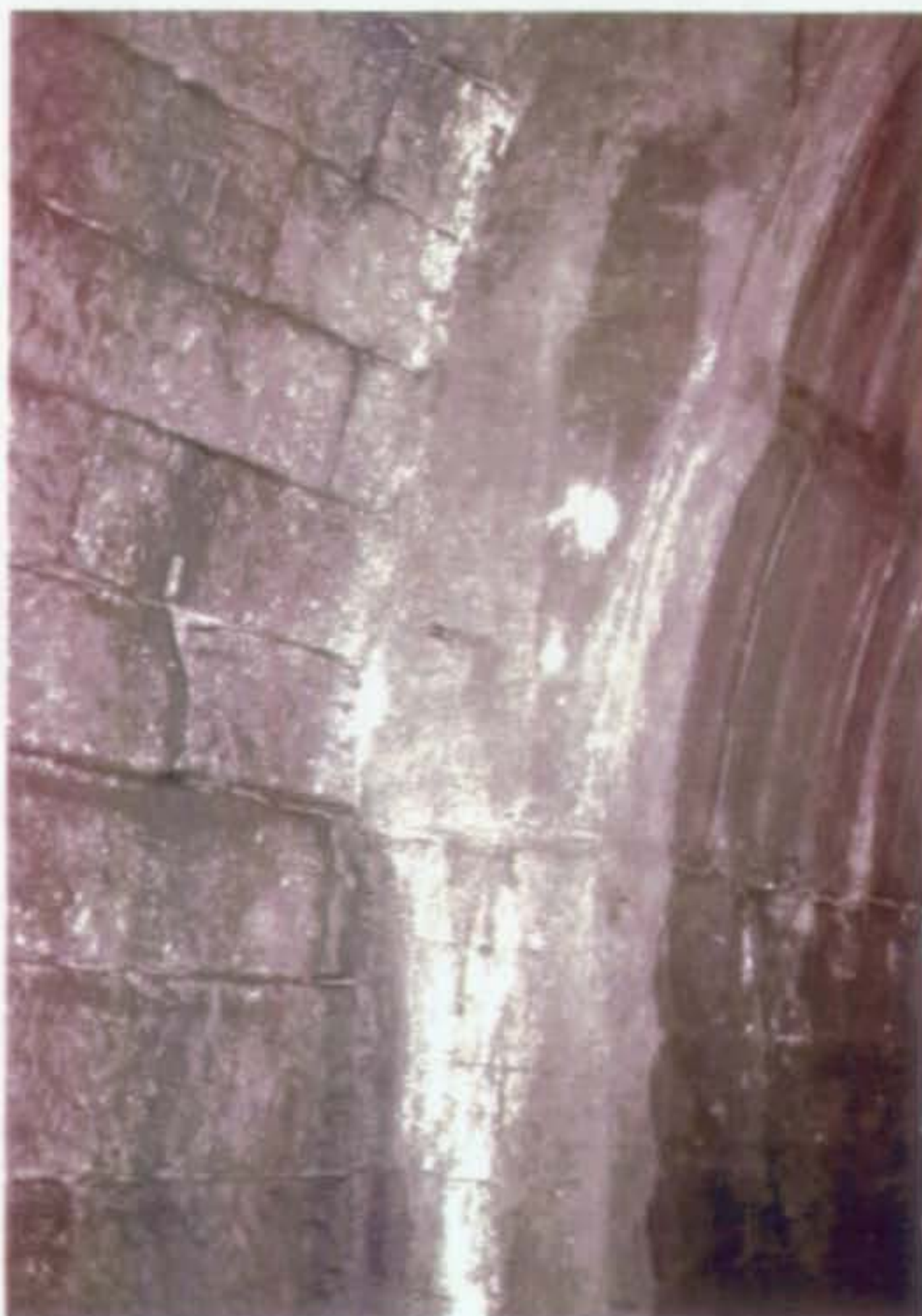
West End, 1990 View of displaced stone near top of north side.
