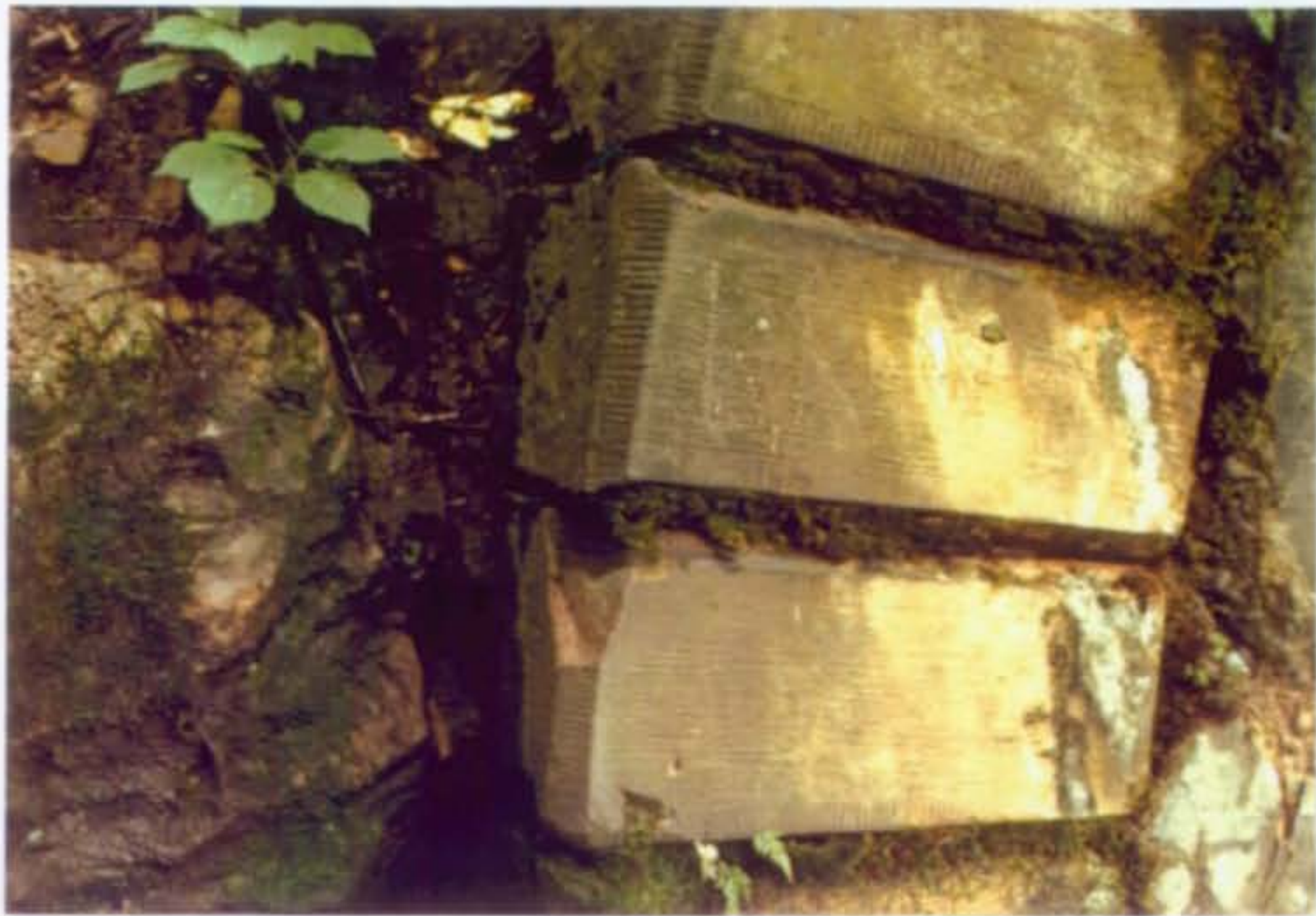
East End, 1990 Beveled and tooled arch stones.
