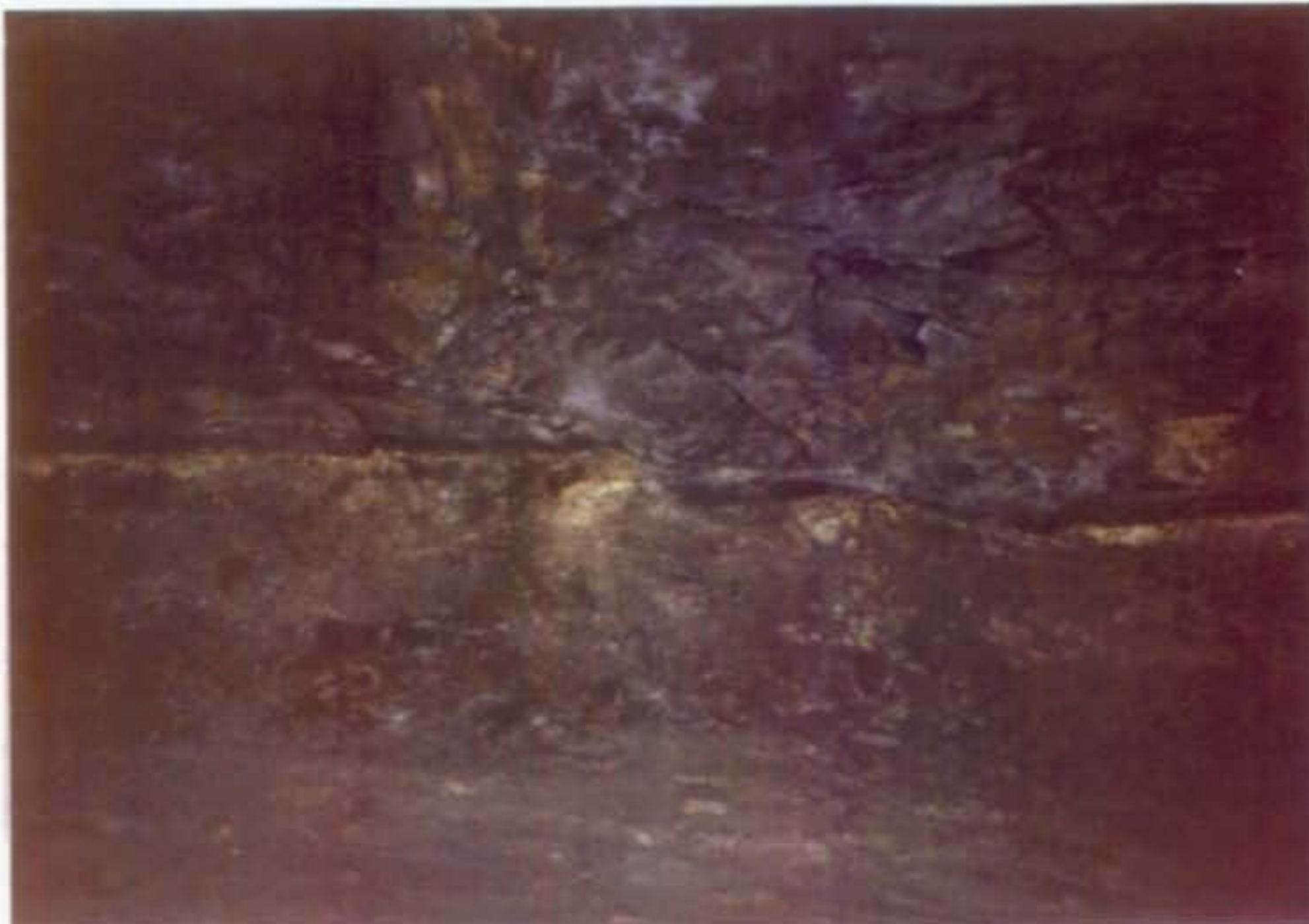
Fault with displacement of coal bed near Sta. 6+50.
