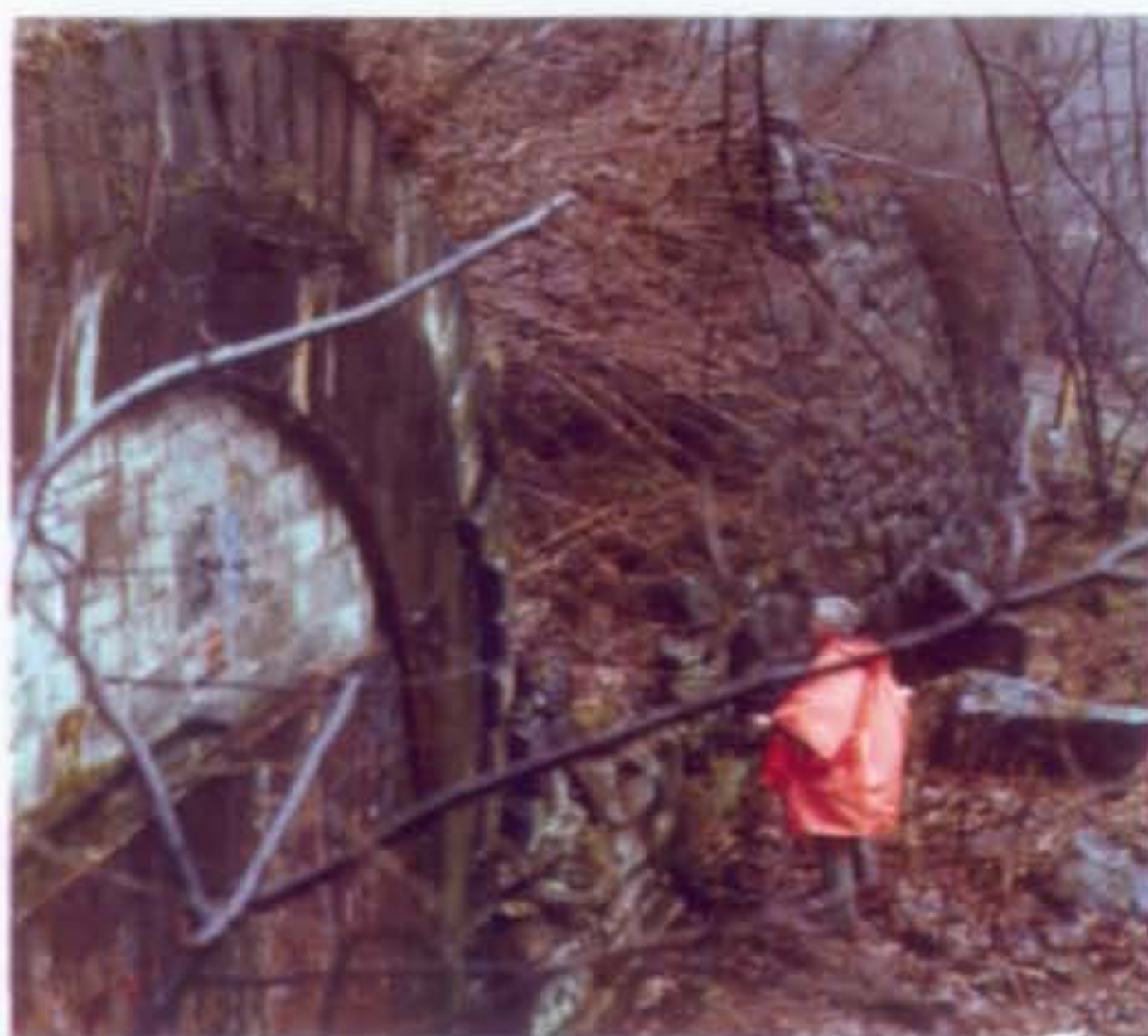
East End, 1990 View illustrates relative height of dry-laid retaining wall.
