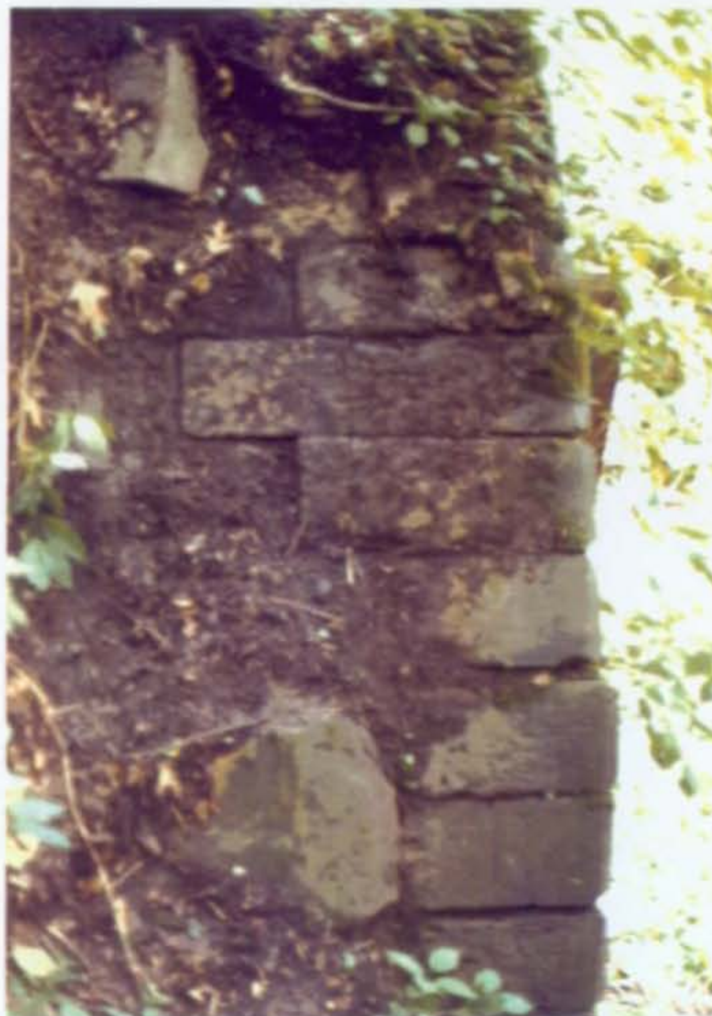
East End, 1990 View of arch construction at south side. NOTE: Two stone lengths at beginning of coursing. Earth cover is non-existent.
