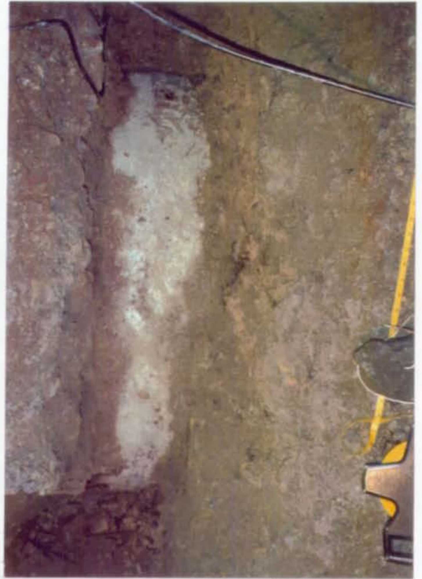
Test Pit No. 2: 48 inch outside diameter concrete water supply line at Sta. 3+00.
