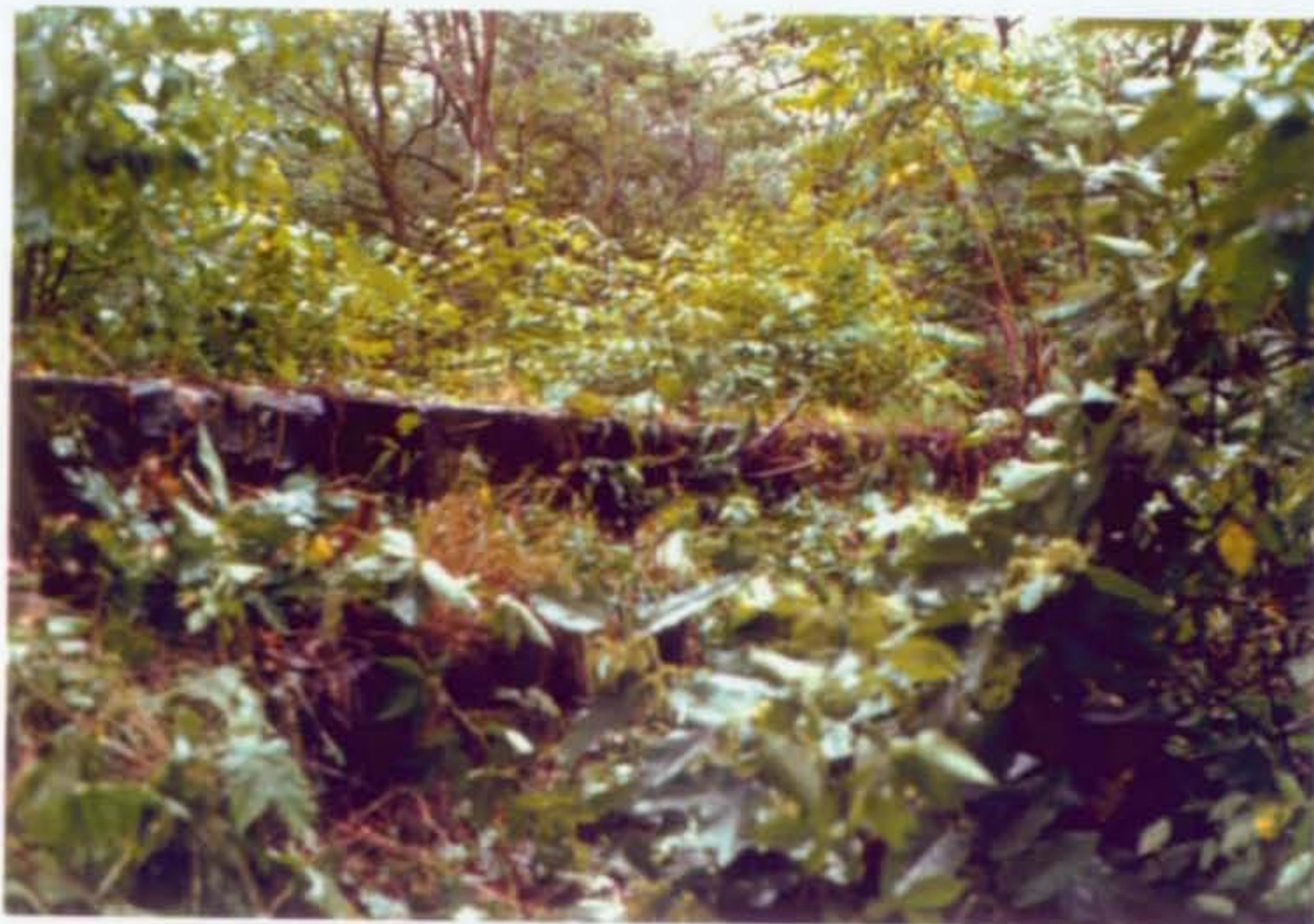
West End, 1990 Rear of facade parapet.
