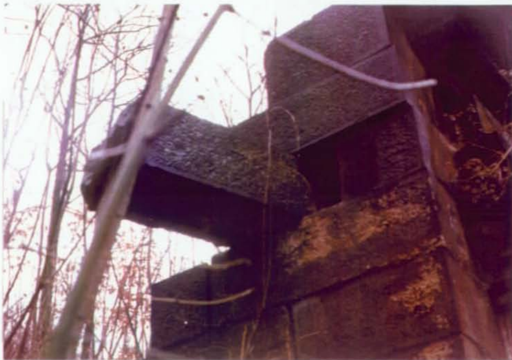
West End, 1990 View of displaced stone near top of north side.
