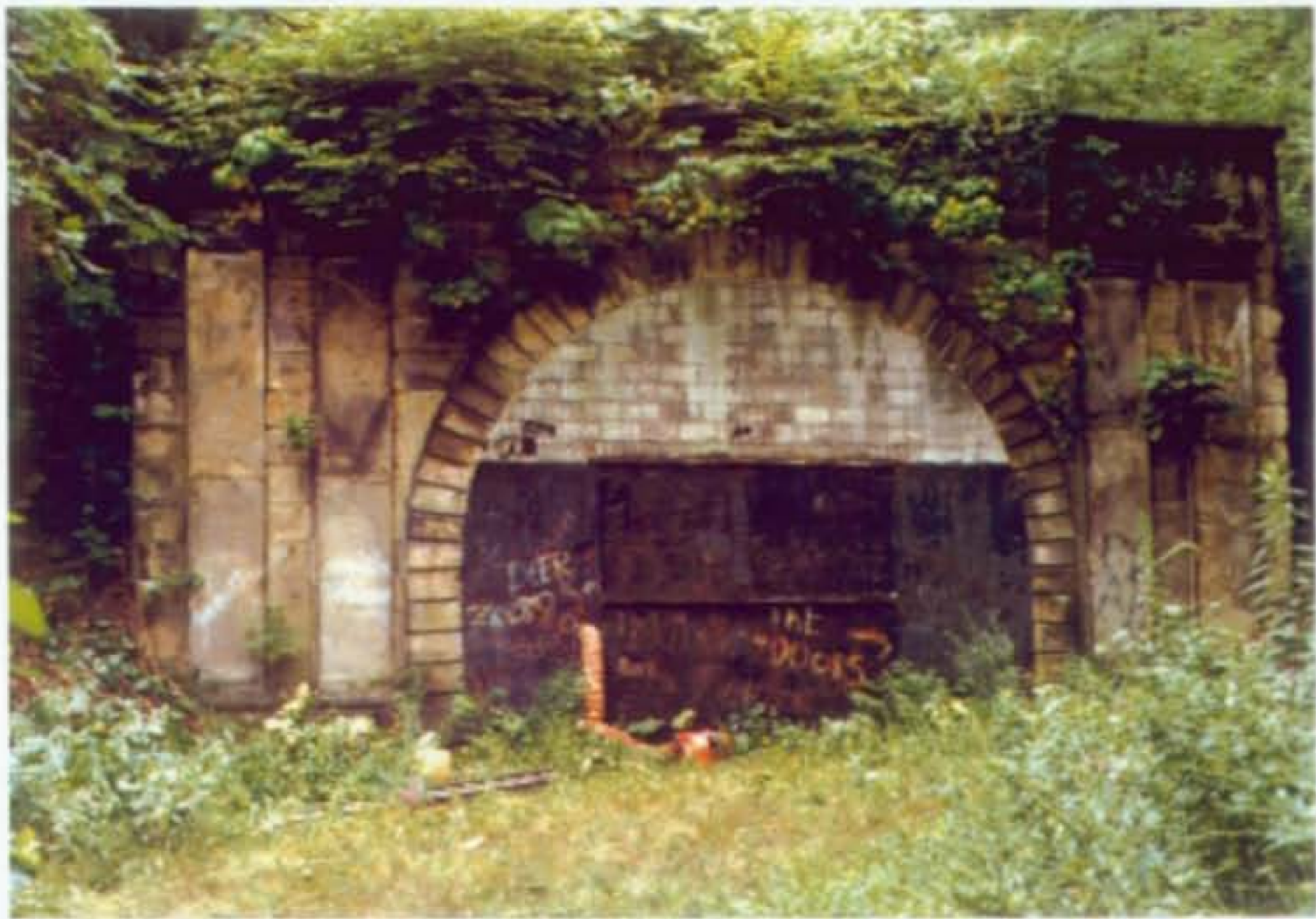
West End, 1990 Retaining walls are missing. Grade has sloughed and covers portions of stone base. Excessive growth aids deterioration.
