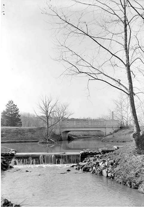
Memorial Bridge showing check dam, stone edging around pool, and tree planted on small island. (APCO n.d. file 102/2497)
