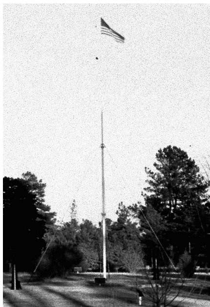
Figure 11. The new iron flagstaff installed in October 1930, from a detail of a 1930 photograph (Poplar Grove CLR:86, The Library of Virginia, from Virginia Room Exhibit at the 1939 World's Fair, image/WF/05/06/017).
