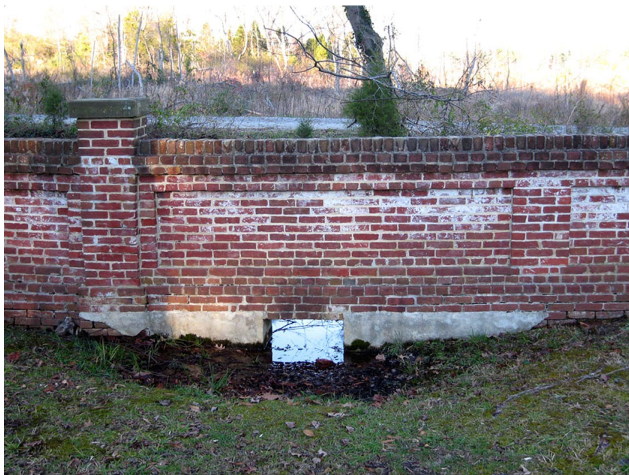
Figure 25. The brick inclosure wall, showing one of the eight drainage holes (SUNY ESF, 2006).
