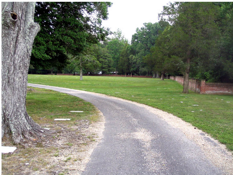
Figure 21. The main drive, looking east from near the rostrum showing asphalt paving with gravel surface coat (SUNY ESF, 2006).
