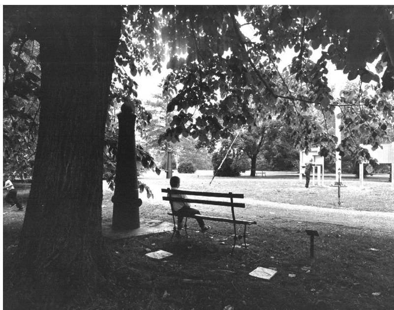
Figure 14. July 1968 view northeast across the center of the cemetery. Note signs near the flagstaff installed in c.1957 (Poplar Grove CLR:115, Photograph by Fred Bell, June 2, 1968, Poplar Grove administrative records, Petersburg National Battlefield).
