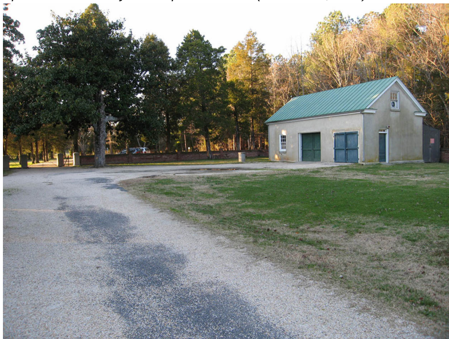
Figure 20. The garage and service yard, looking west from the burial grounds toward the cemetery entrance gate (SUNY ESF, 2006).
