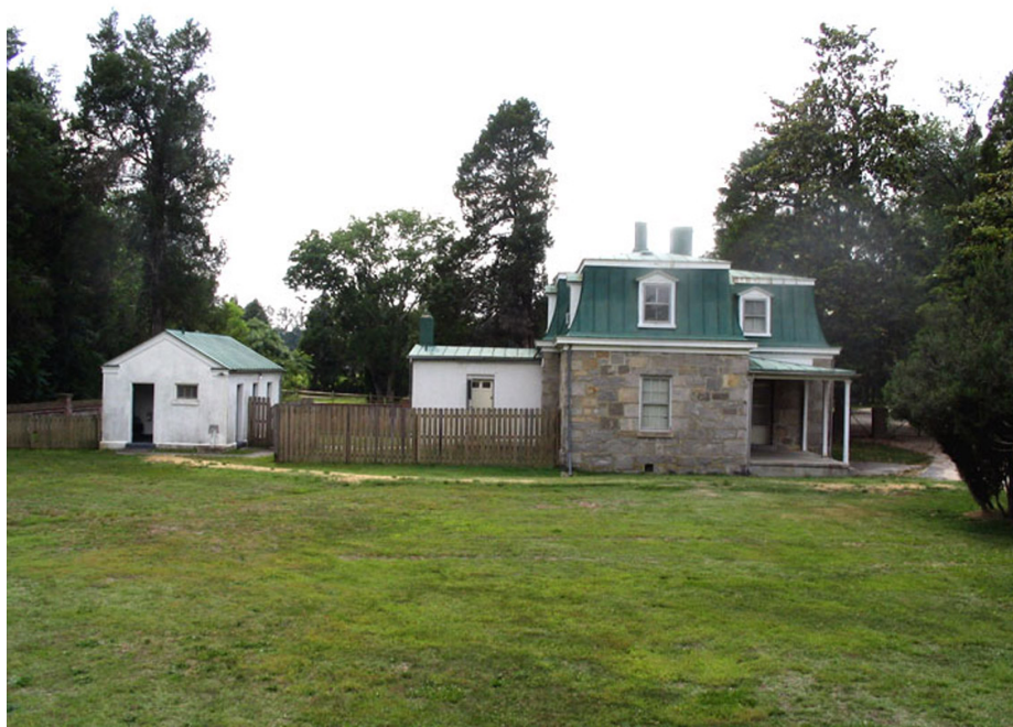
Figure 28. The east side of the lodge with its rear kitchen wing addition and the restroom building at image left (SUNY ESF, 2006).
