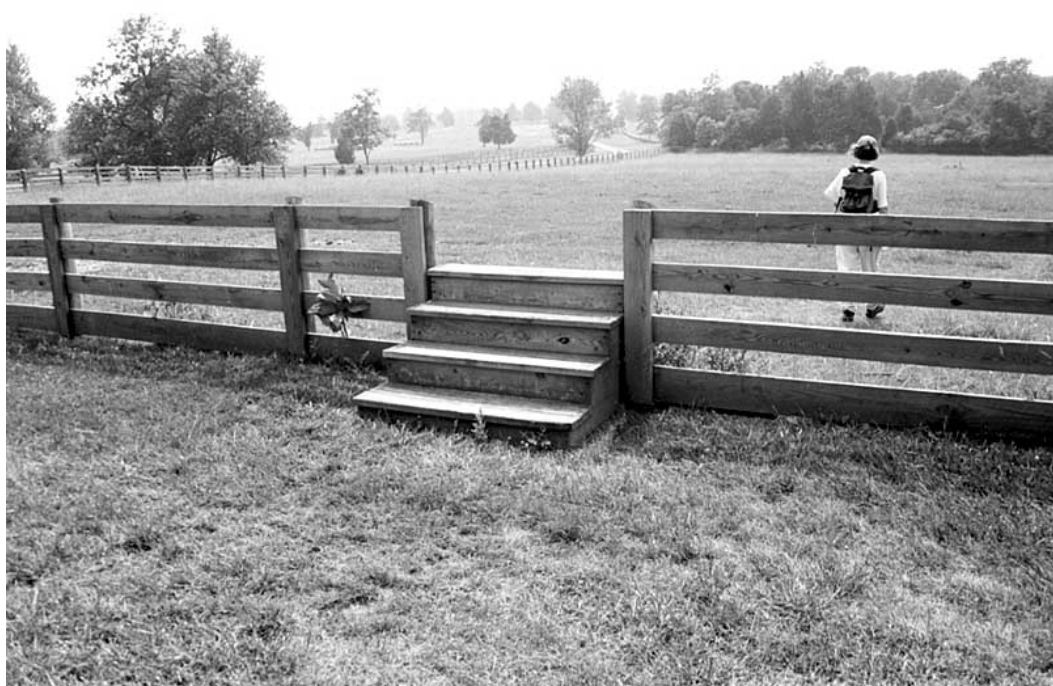
Example of three-step stile. (PHSO 1999)
