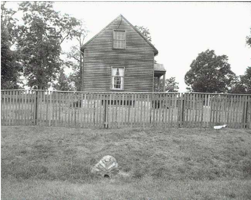
Unusual fieldstone and clay pipe culvert east of Jones Law Office. (PHSO 1999)
