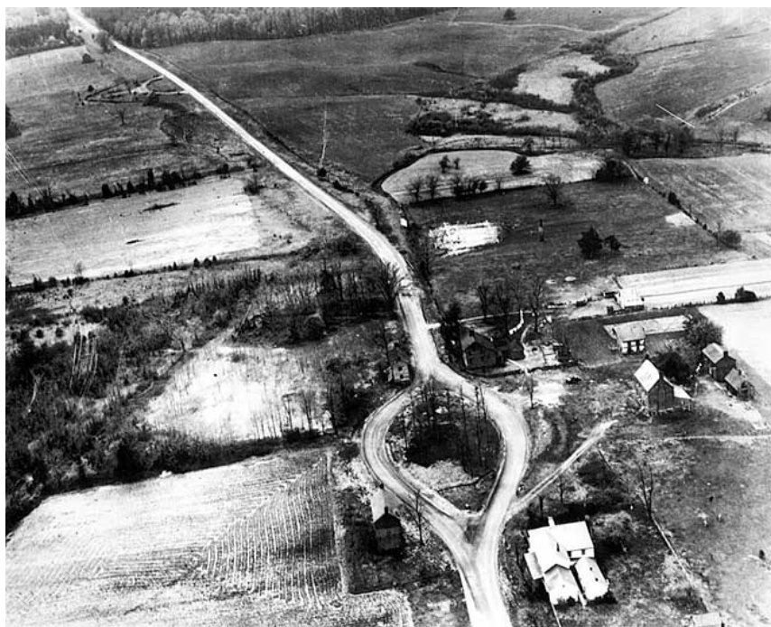
Aerial overview of Appomattox Court House in 1937. (APCO 1937, file 241)
