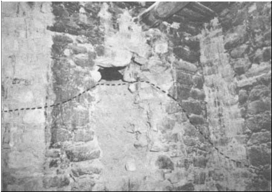
PLATE 10—Lower Room 11, recent break and fill line. Lower Room 11, showing hole made by vandals to gain entrance to unexcavated Room 10 and from which a considerable amount of fill drifted into Room 11. Dashed line indicates level of fill before excavation.
