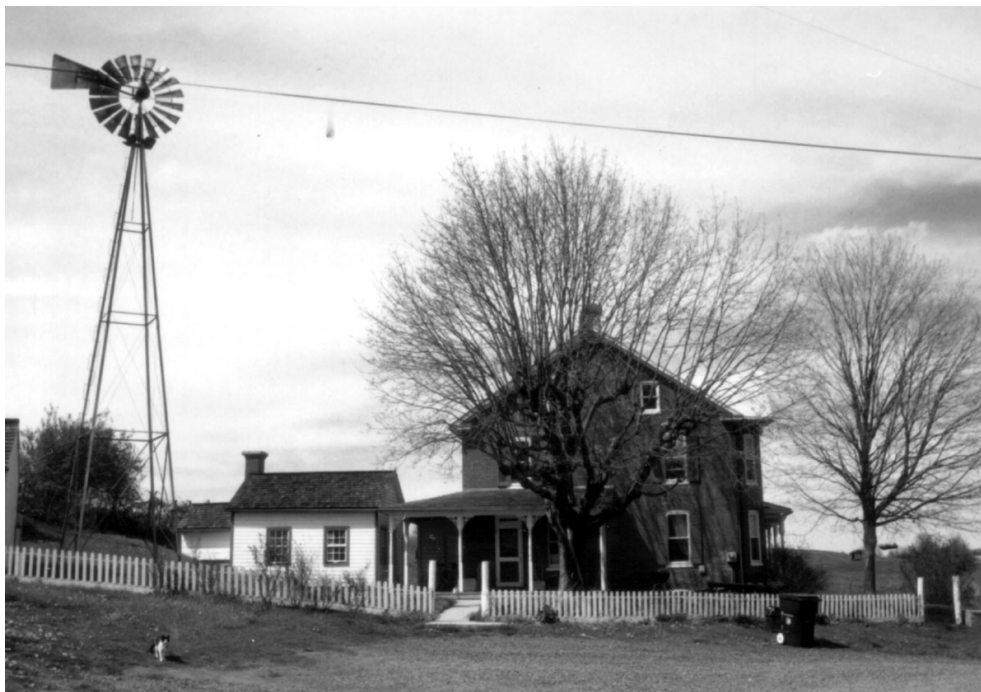
Redding Farmhouse, north façade, 2000. The summer kitchen is to the left.
