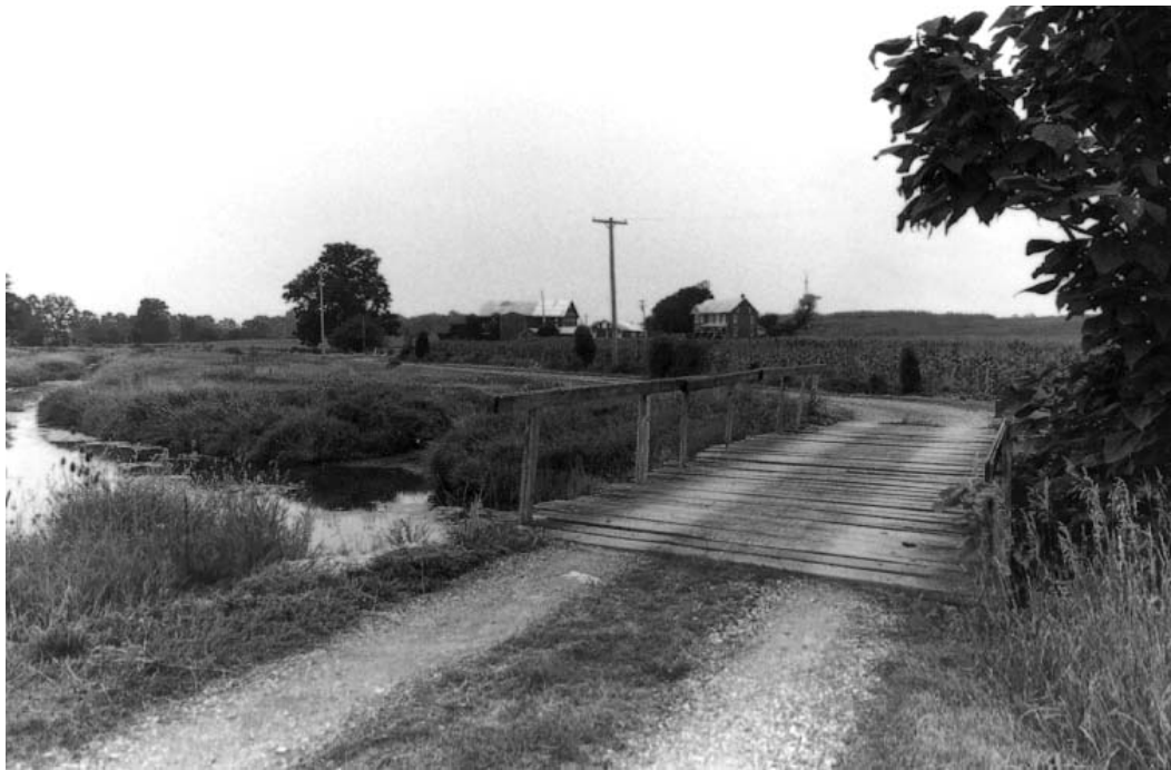
Bridge over Willoughby's Run, replaced in 1996.
