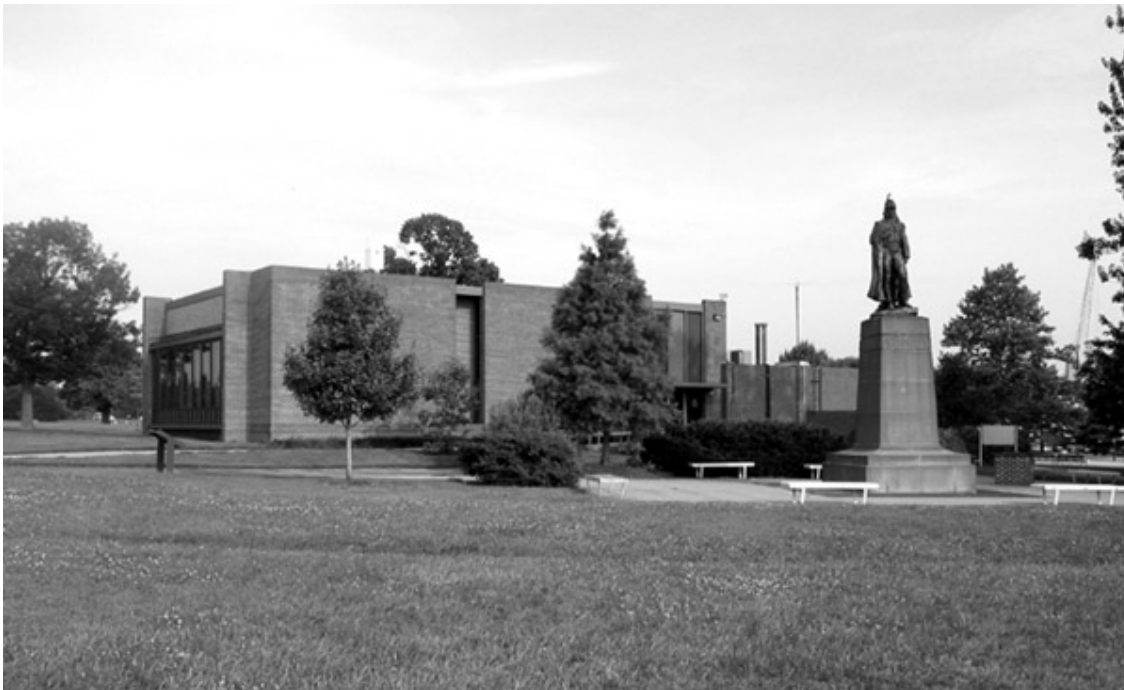
Figure 22: Visitor Center, built 1963-64 during the period MISSION 66 period and located approximately 300' north of the Fort. It exhibits a functional contemporary design typical of late 1950s and early 1960s modern architecture. OCLP, July 2003.
