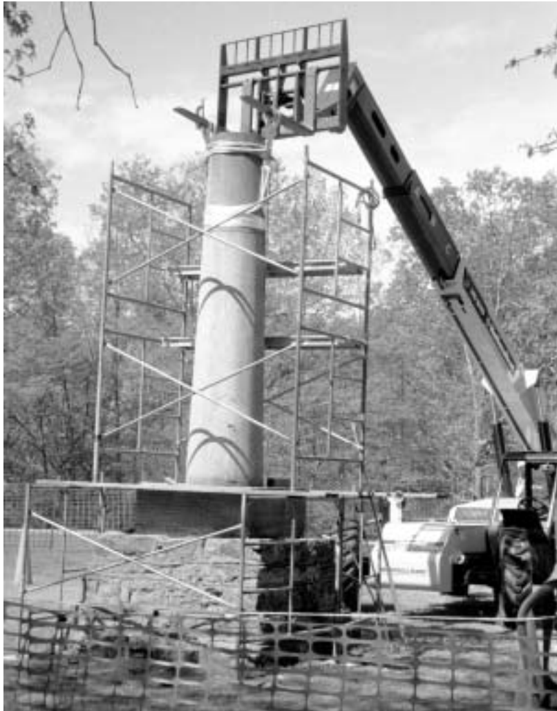
Figure 30. Base of Monument during rehabilitation, 2000.
