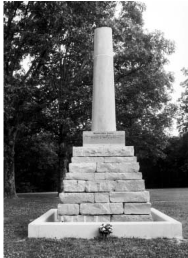
Figure 31. Monument after rehabilitation, 2002.
