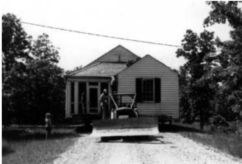
Figure 28. Superintendent's residence being moved, 1960.
