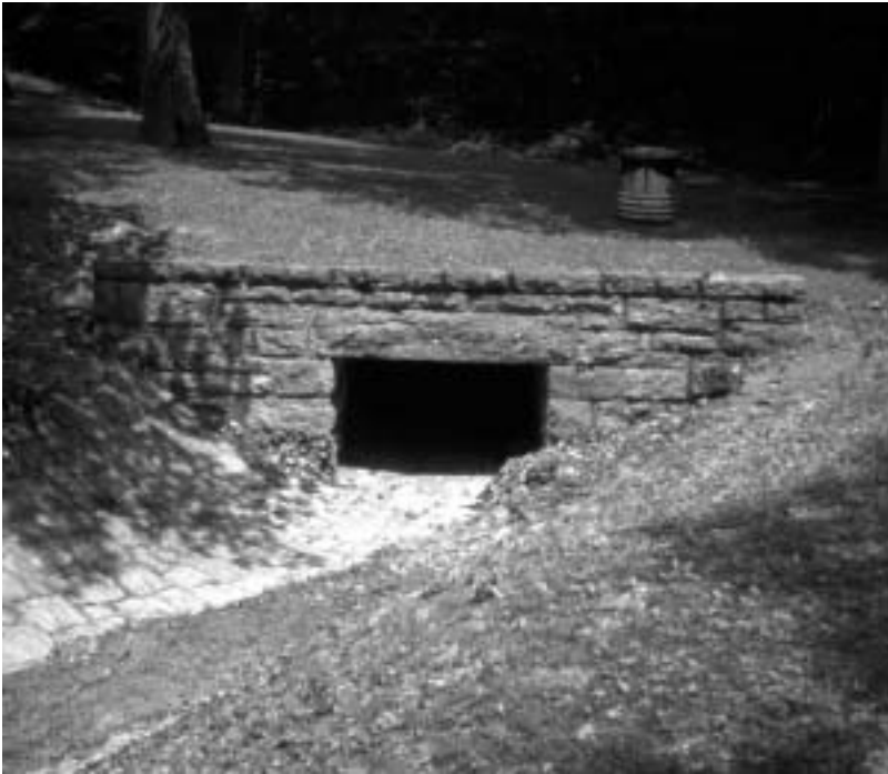
Figure 64. Stone detailing at Old Spring picnic area, 2001.
