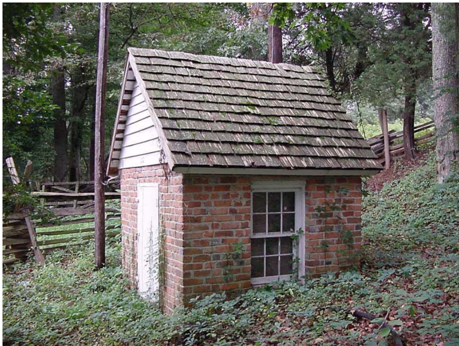
Photo 33. The brick pump house.
