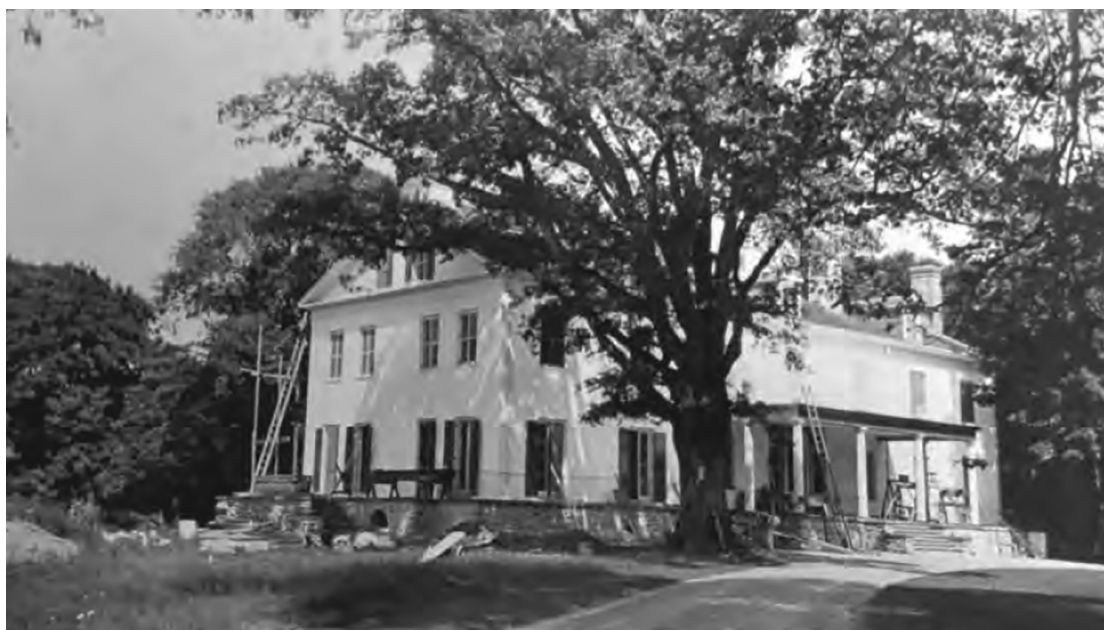
Figure 7. Expansion and renovation of Bellefield house nearing completion, looking northwest at the front and south sides, 1911. (Newbold-Morgan Collection, ROVA Archives)
