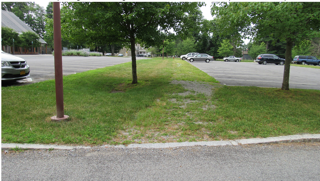
Figure 30. The mostly grass-covered gravel walkway designed to interpret the historic alignment of Estates Road through Bellefield's west field, looking south toward the FDR Library. These grass medians were designed as infiltration areas with herbaceous vegetation, which the park could not maintain. (SUNY ESF, 2019)
