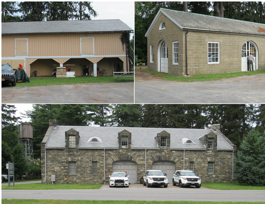
Figure 33. Outbuildings at the service yard, from upper left: Old Barn looking north across the service yard; Old Garage looking northwest from the service road; and the New Garage looking west across FDR Drive (park entry-exit road). The water tower is visible to the left of the New Garage. (SUNY ESF, 2019)
