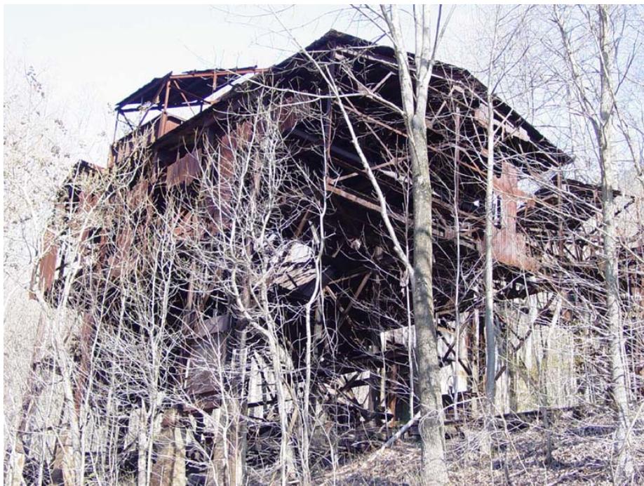
Tipple constructed by Fordson Coal Company in 1923-24 (OCLP 2003).
