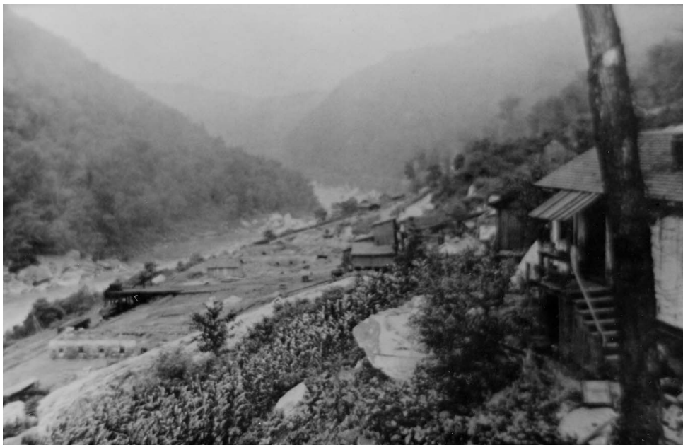
Original tipple, wooden structure with tower in midframe, in 1875. Banks of coke ovens lie perpendicular to river (NERI 315).
