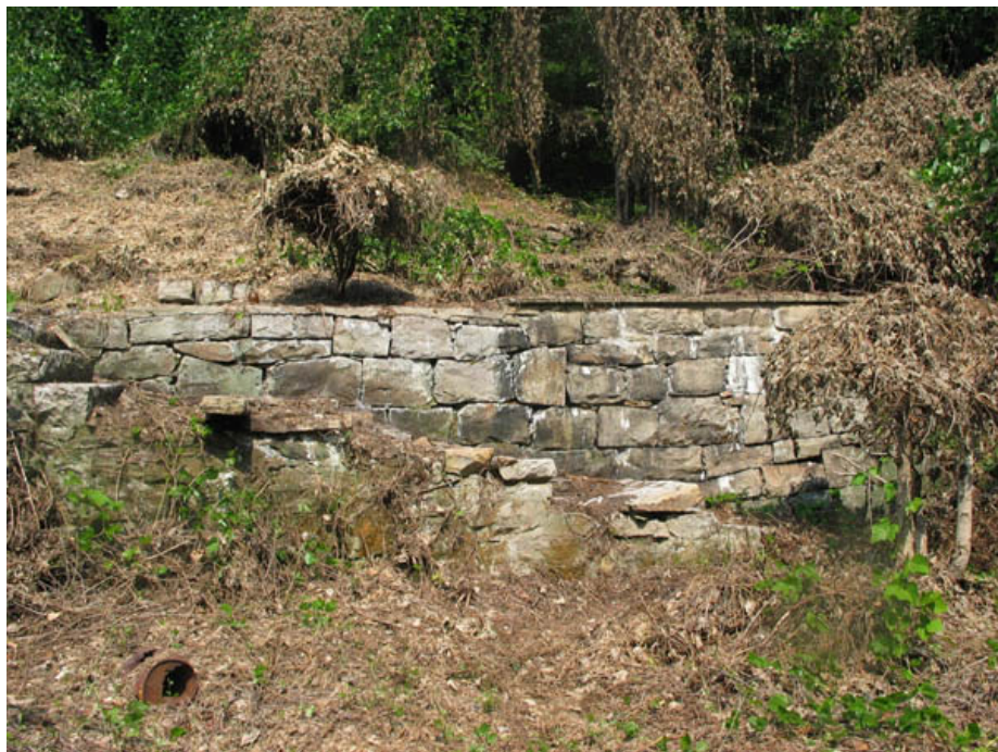
White Clubhouse retaining walls after kudzu removal in Summer 2006 (NRGMR, 2006).
