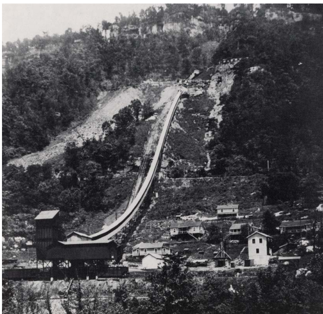
Nuttallburg, taken after completion of the new conveyor and tipple by Fordson Coal Company, 1927 (NERI 312).
