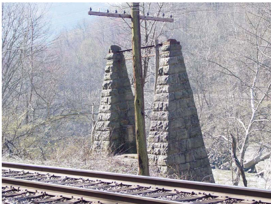
One of the existing stone towers for the Nuttallburg suspension bridge (OCLP 2003).
