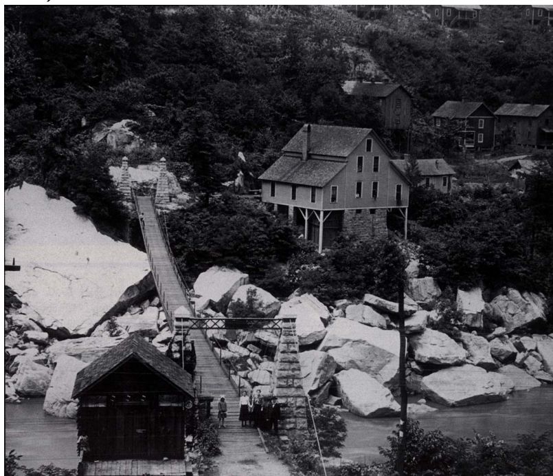
Nuttallburg Suspension Bridge shortly after completion, looking towards South Nuttall, 1899 (C&O Historical Magazine).
