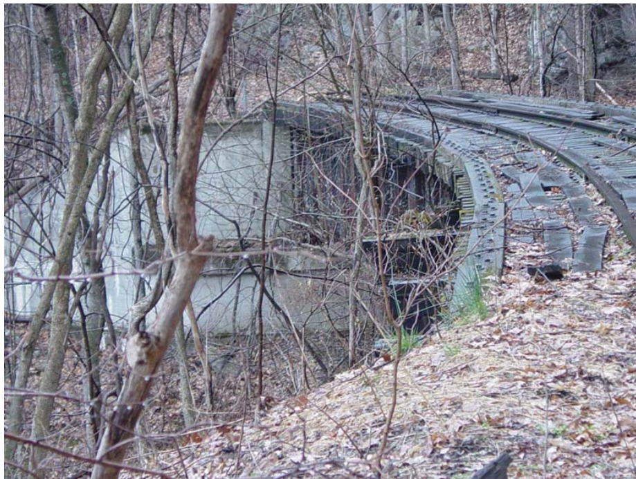
Railroad trestle bridge over Short Creek along Keeney's Creek branch line above Nuttallburg (OCLP 2003).
