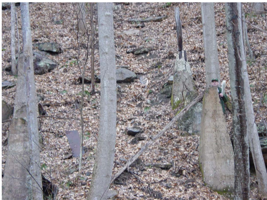
Old conveyor or tippie piers located along the upper level of the Keeney Creek branch line (OCLP 2003).
