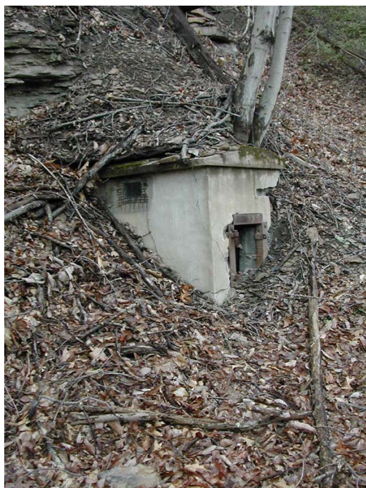
Cap House located west of the Headhouse (OCLP 2003).
