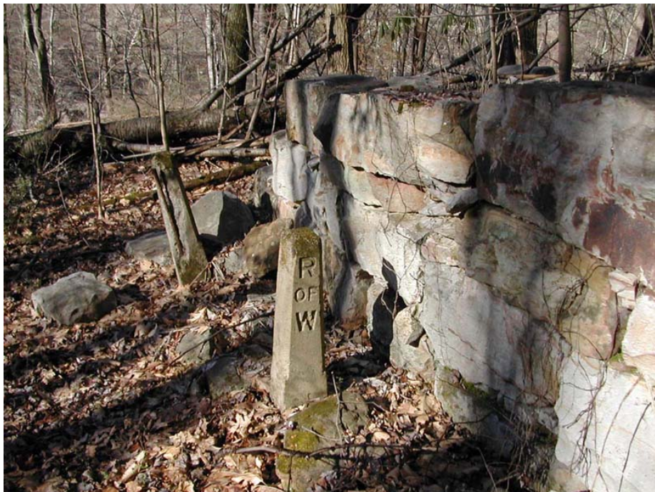
Concrete railroad marker beside the Black School foundation ruin (OCLP 2003).
