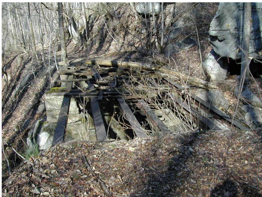
Short Creek Bridge along Nuttallburg's Town Road (OCLP 2003).
