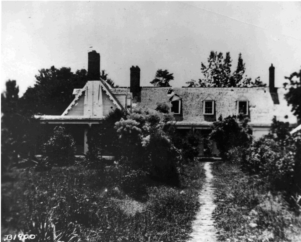
Figure 10. North facade of Appomattox Plantation House, summer 1864(?). Destruction wrought in 1862 is visible in various holes on the house. Lush grounds of overgrown lawn and flowering shrubs line the north-south path. (National Archives, 111-B-1900)
