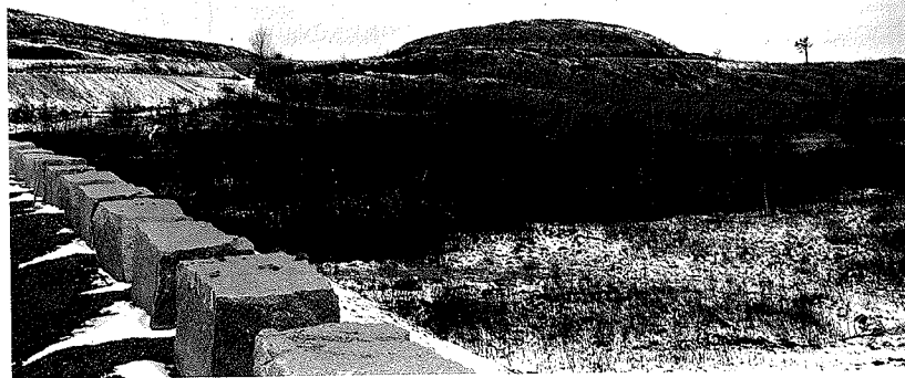
After snags were felled. Some of the snags in this area were burned to get rid of them since this particular area is so visible from the roads. Paradise Hill Road & New Eagle Lake Road underpass in distance - Bar Harbor Approach Road in foreground.
