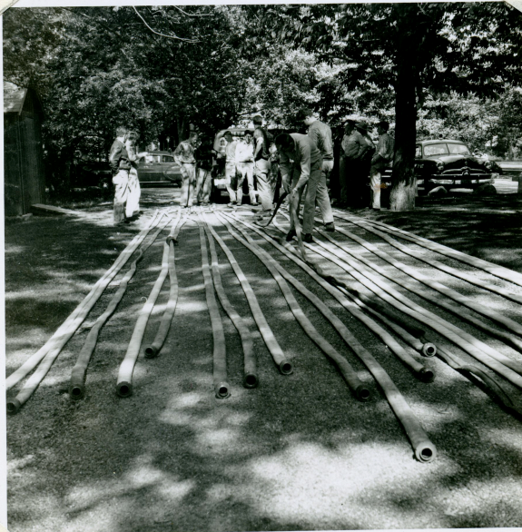
Process used in drying fire hose after training session in Acadia National Park.
