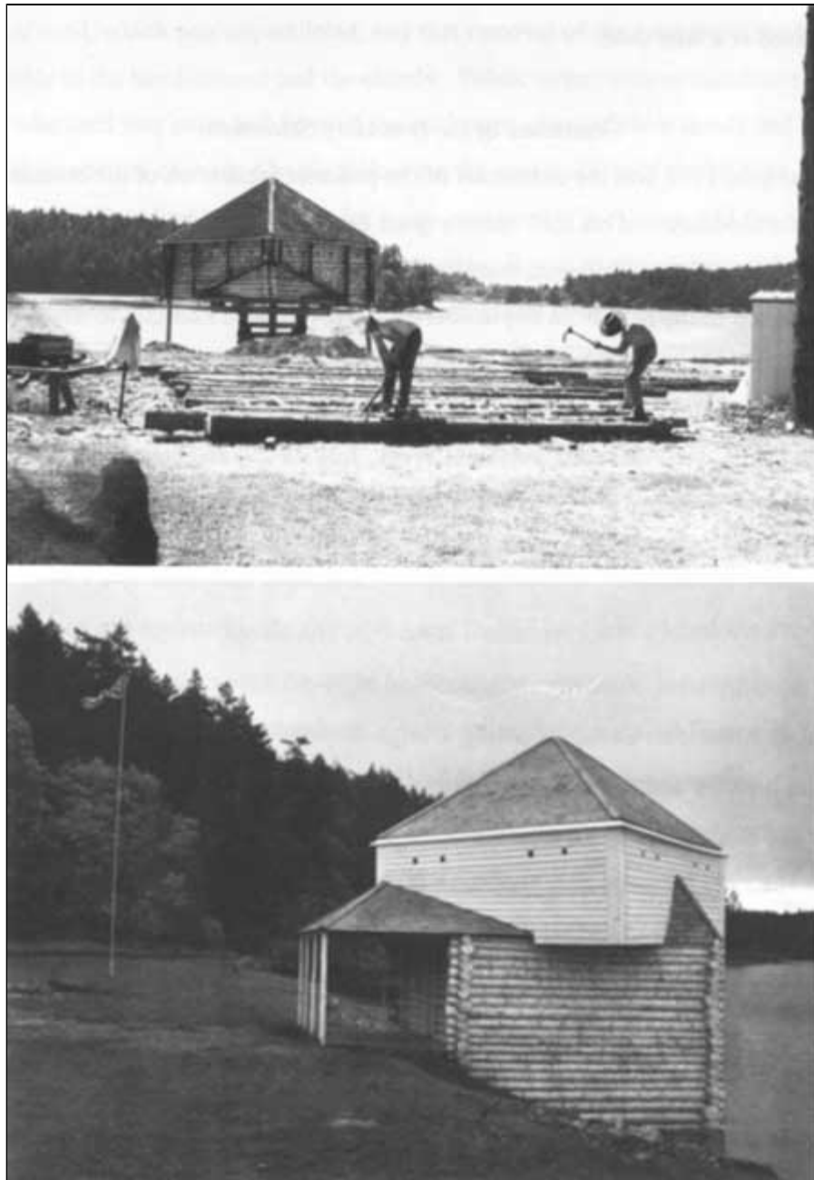
The Blockhouse during and after restoration.
