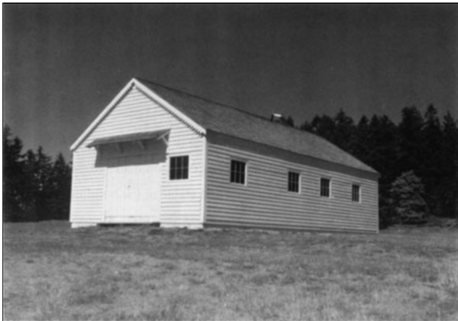
The restored Commissary.
