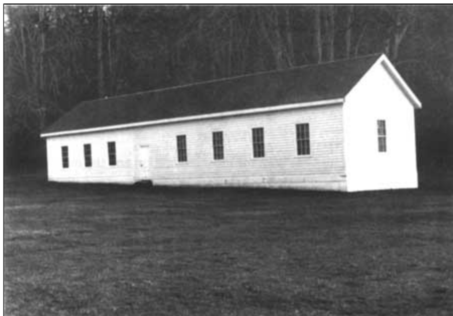
The restored Barracks building.
