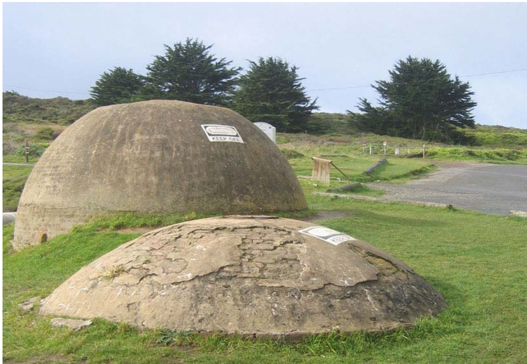
Buildings and Structures #3: View of two of the three cisterns with the Coast Guard Complex showing the brick structure revealed beneath the flaking plaster. (PWR, CLI, GOGA-D-1-25 035, 2005)
