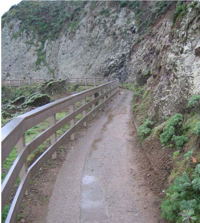
Circulation #1: View of the Lighthouse Trail and cartway, note the asphalt center strip. The wooden type of hand railing is on the left. (PWR, CLI, GOGA-D-2-25 005, 2005)
