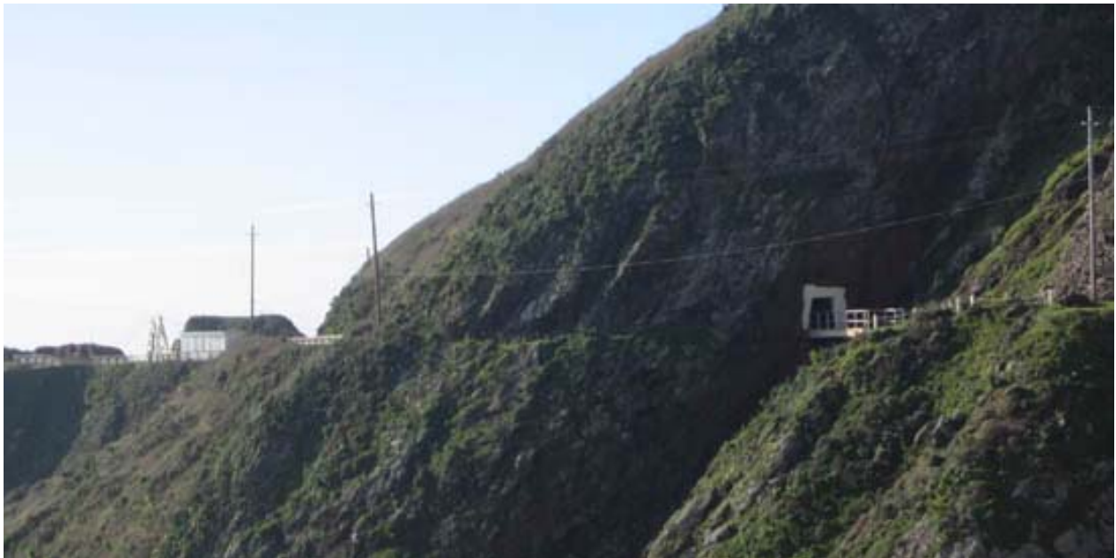
Topography #1: The cut associated with the wooden galley, which was replaced in 1876 by the tunnel following a landslide, is still visible in the cliff. (PWR, CLI, GOGA-D-2-22 043, 2005)
