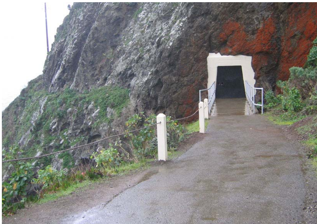
Buildings and Structures #2: View of the east entrance to the tunnel and a portion of the Lighthouse Trail. (PWR, CLI, GOGA-D-1-25 001, 2005)
