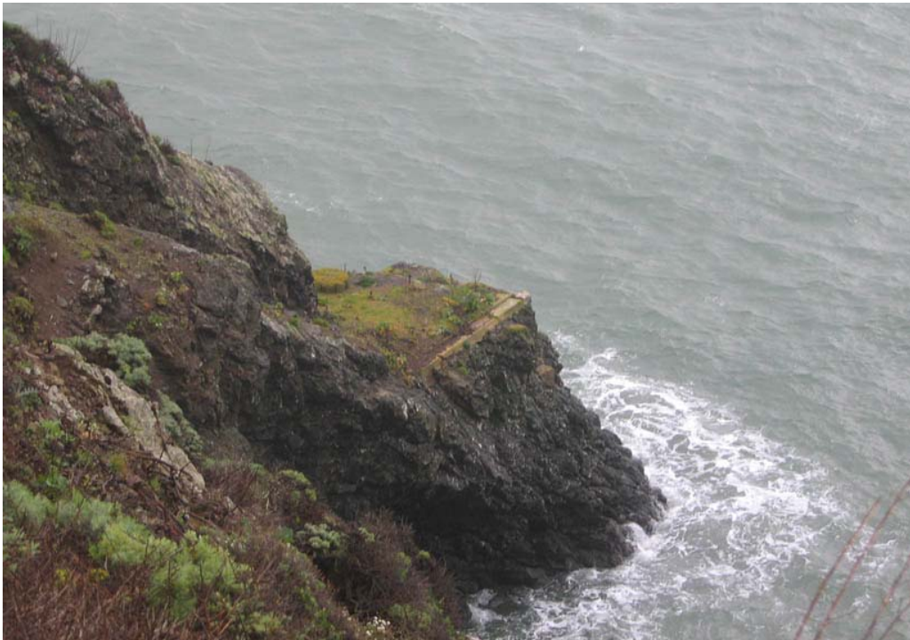
Archeological Sites #2: View of the remains of the landing structures at the bottom of the incline tramway. (PWR, CLI, GOGA-D-1-25 006, 2005)
