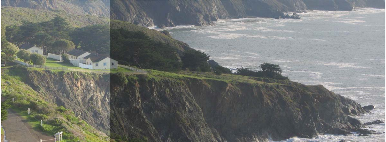
Buildings and Structures #4: Overview of the Coast Guard residential complex. All three residential structures, copses of Monterey cypress and the picket and board fences can be seen. (PWR, CLI, GOGA-D-2-22 011/012, 2005)
