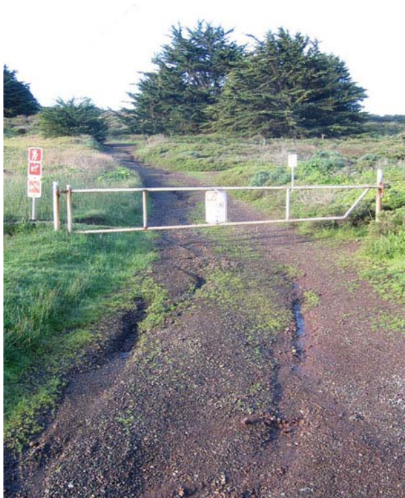
Circulation #3: View of the east end of the Bonita Ridge Access Road, the red chert gravel is typical of the road surface during the period of significance. (PWR, CLI, GOGA-D-2-22 001, 2005)
