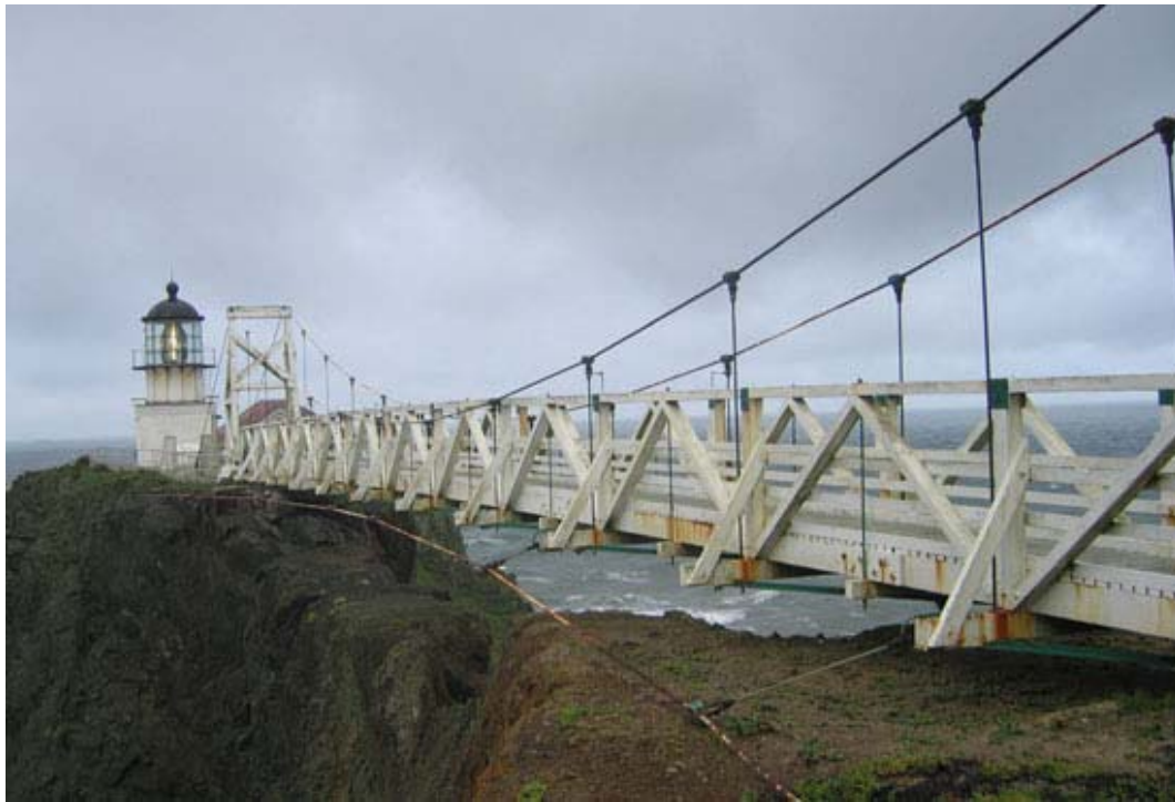
Buildings and Structures #1: View of the Lighthouse Tower and suspension bridge, the roof of the fog-signal building is visible in the background. (PWR, CLI, GOGA-D-1-25 014, 2005)
