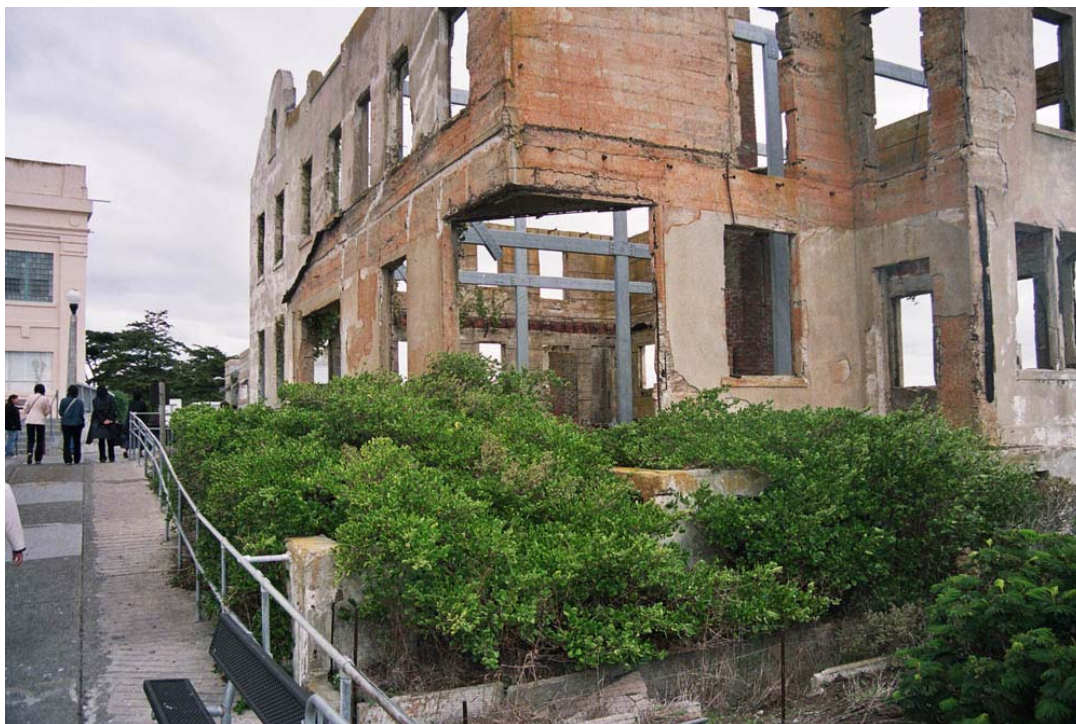
Remains of the greenhouse foundation on south side of Warden's house (No. 79). View to E. (112_11_0049, D. Bradley, 2004)
