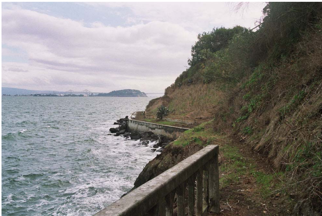
View of the perimeter walk on the east side of island, taken from the Building 79. View to SE. (115_4_0121, D. Bradley, 2004)
