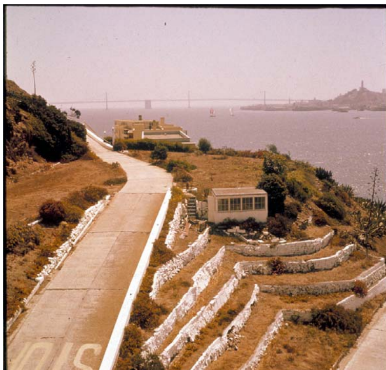
West Lawn and Tool Shed Terraces in ca. 1960 during the Federal Prison Era. (Source: Fischetti Photographs in GOGA Archives No. 18352-049)
