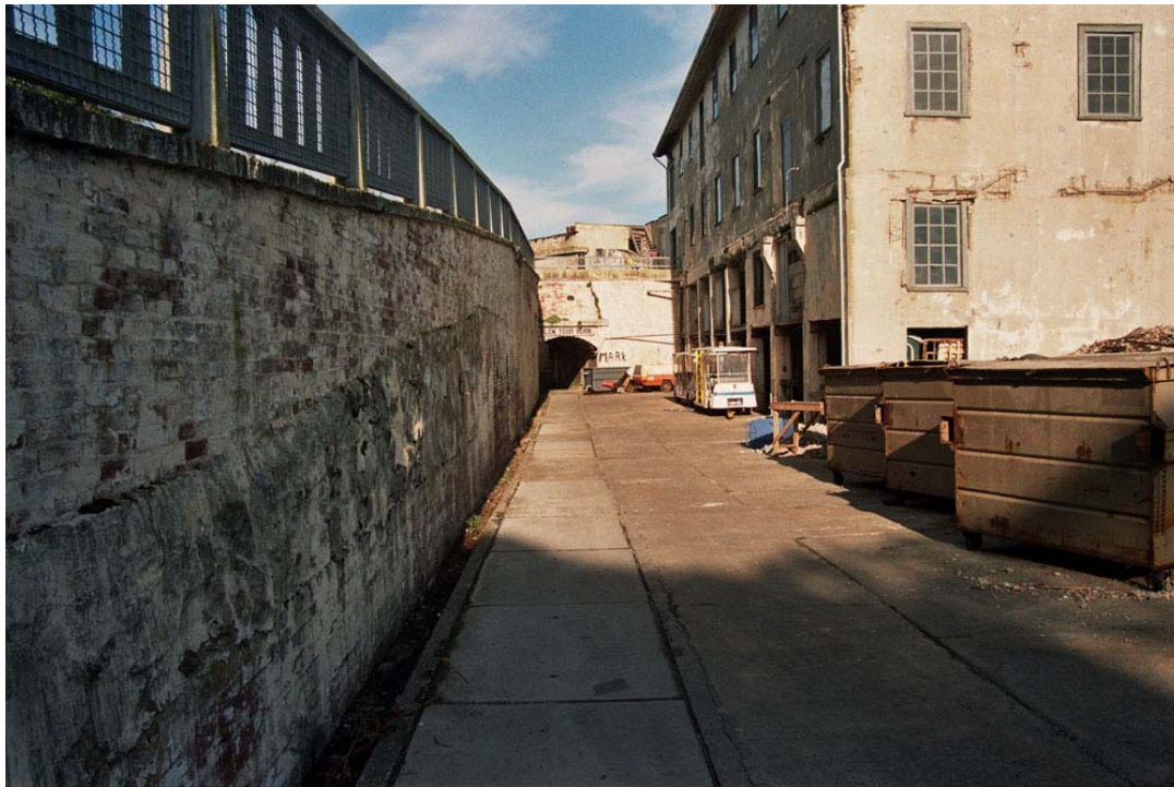
View of No. 79 (right side), brick retaining wall of fortifications (left side), and tunnel of fortifications (background). View to N. (935_12A_0043, D. Bradley, 2004)
