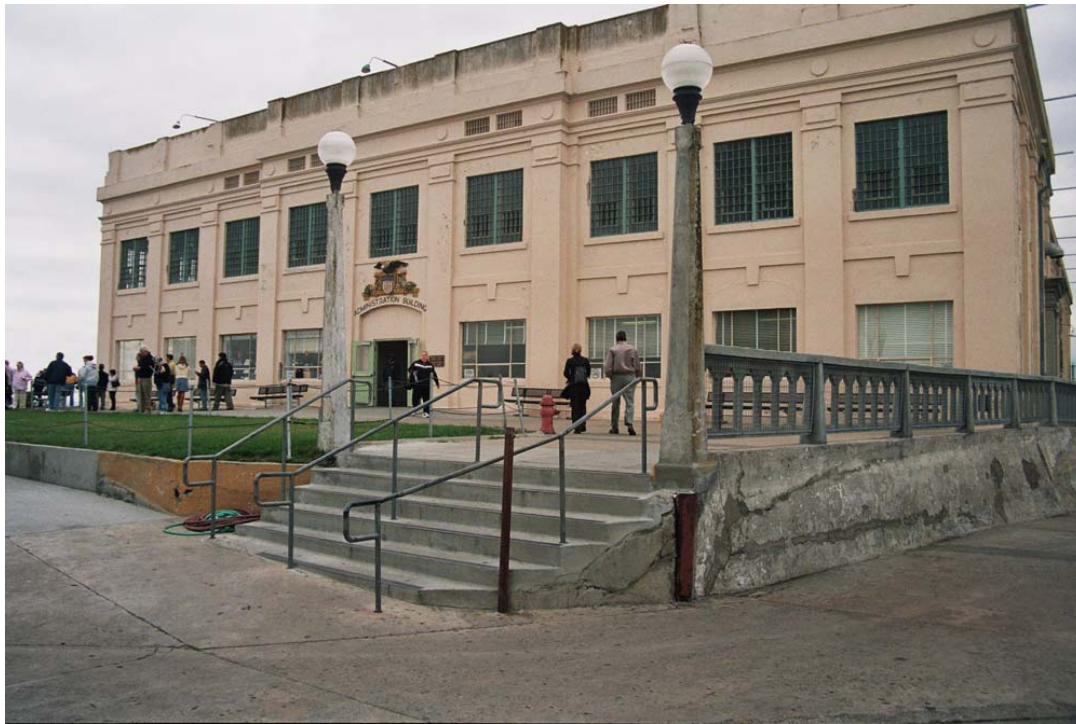
Cellhouse (No. 68) and front terrace. View to W. (115_22_0139, D. Bradley, 2004)
