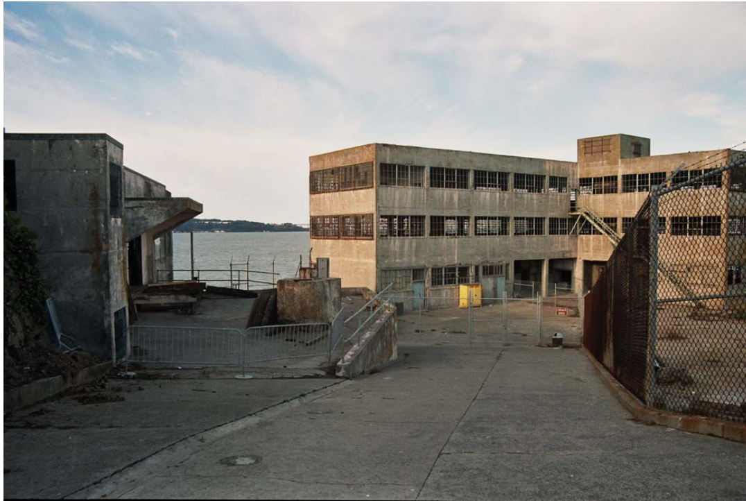
Overview of north end of island – Model Industries Building (No. 82) (background) and New Industries Building (No. 84) (left). View to W. (935_4A_0035, D. Bradley, 2004)
