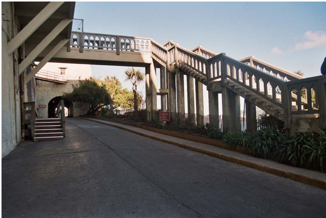
Road to Sallyport (in background) with view of raised concrete overpass (in foreground). View to N. (113_15_0077, D. Bradley, 2004)
