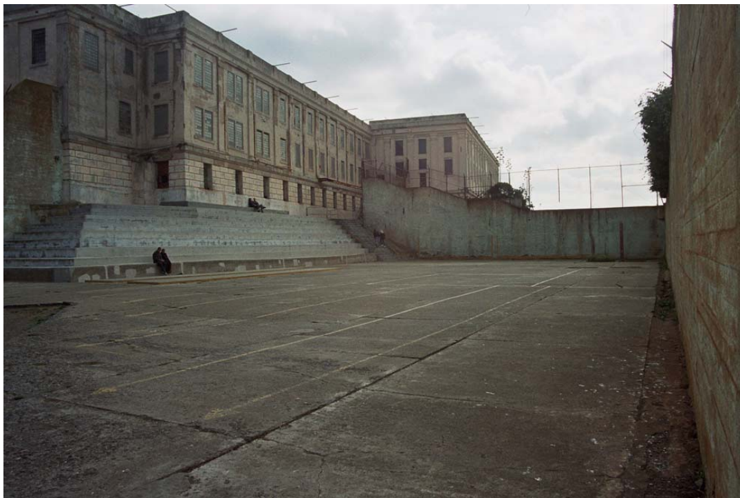
Recreation Yard. View to E. (752_17A_0020, D. Bradley, 2004)
