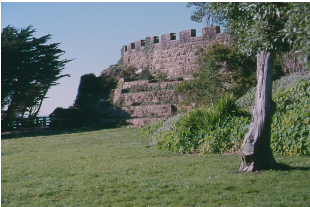
Buildings and Structures #2: View of the Parapet from the South Esplanade. (PWR, CLI, GOGS-S-0002-29, 2004)
