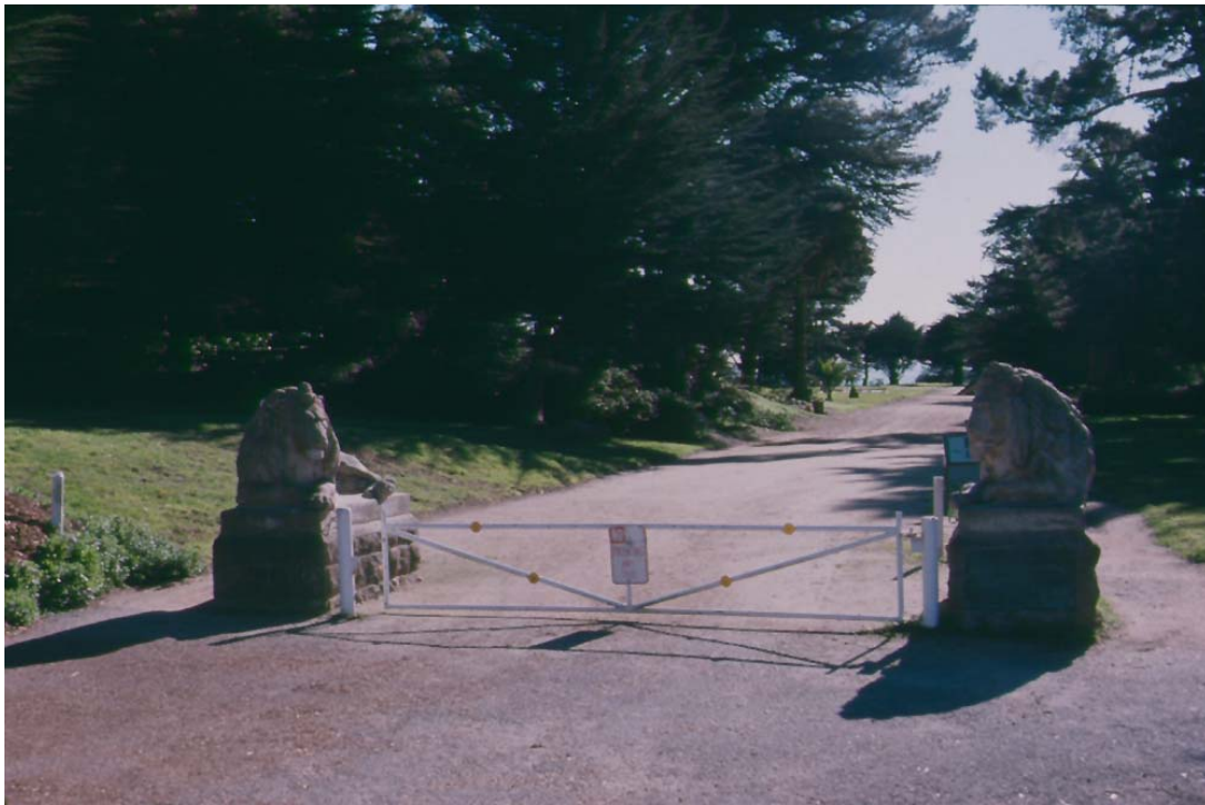
Circulation #1: View of Palm Avenue looking toward the southwest. (PWR, CLI, GOGS-S-0002-23, 2004)
