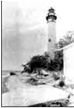
Erosion threatened the South Manitou lighthouse in 1986.
