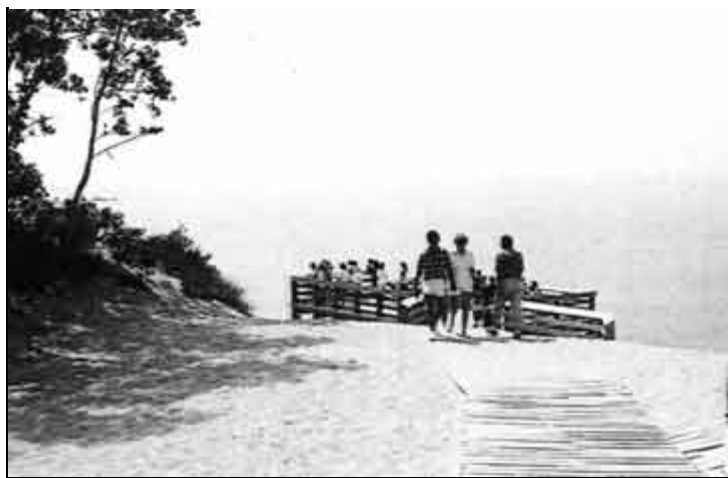
The Lake Michigan overlook platform, Pierce Stocking Drive, 1989.
