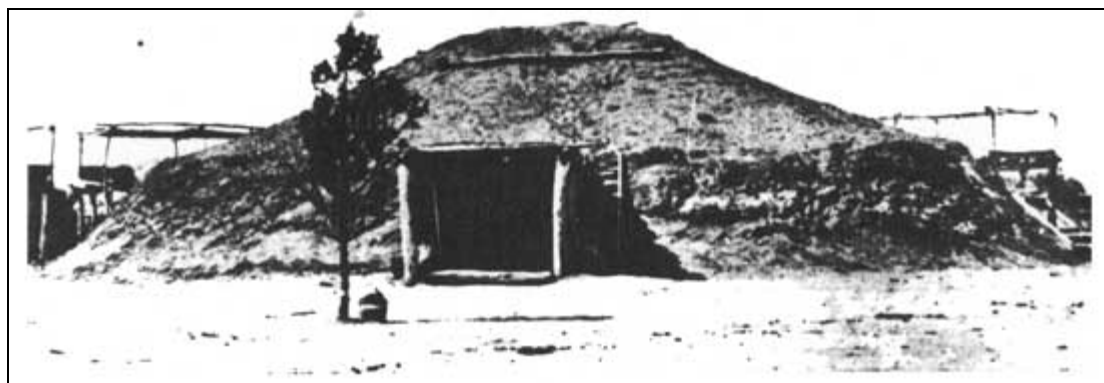
An historic, Arikara earth lodge photographed in 1870 at Like-a-Fishhook Village in central North Dakota. This ceremonial lodge though larger than the ordinary house, is much like the circular lodges of the Coalescent Tradition uncovered by archeologists. (Photo courtesy of the State Historical Society of North Dakota).
