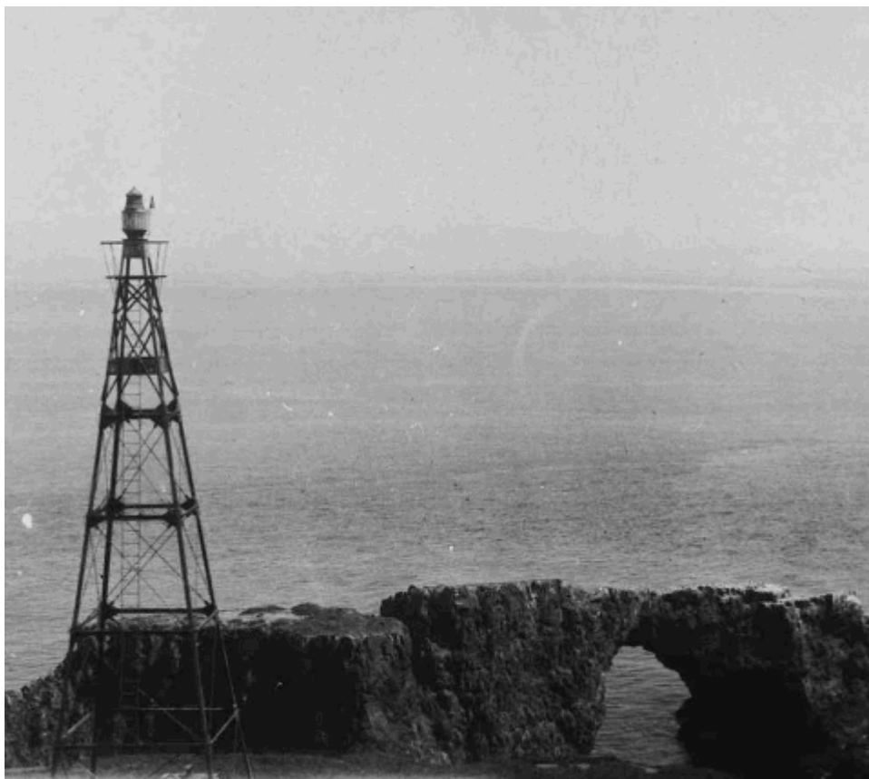
History #2: Circa 1911 to 1932 photo of the original acetylene light was a simple steel skeleton tower, fifty feet east of the present lighthouse. (US Coast Guard Historians Office collection)
