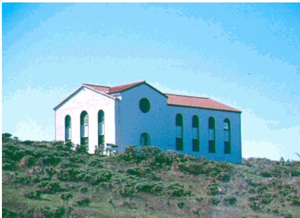
Buildings and Structures #3: Note the stepped roof line and half-barrel chimney cap on the power house. (PGSO, LCS, 2001)
