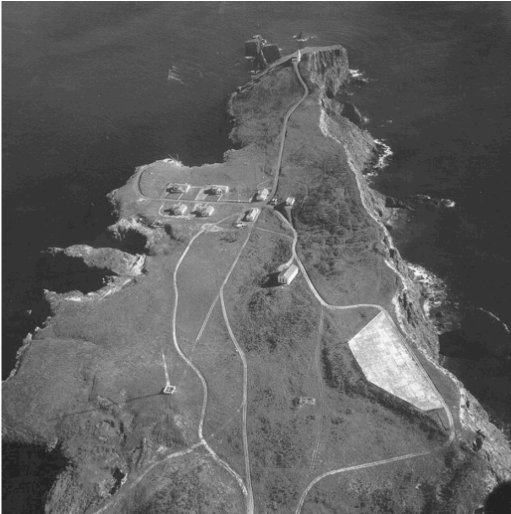
History #5: An aerial view of Anacapa Island Light Station, December 6, 1963, before the demolition of the three residences, paint storage shed and lower derrick building. (U.S. Navy photograph, Channel Island National Park archives)
