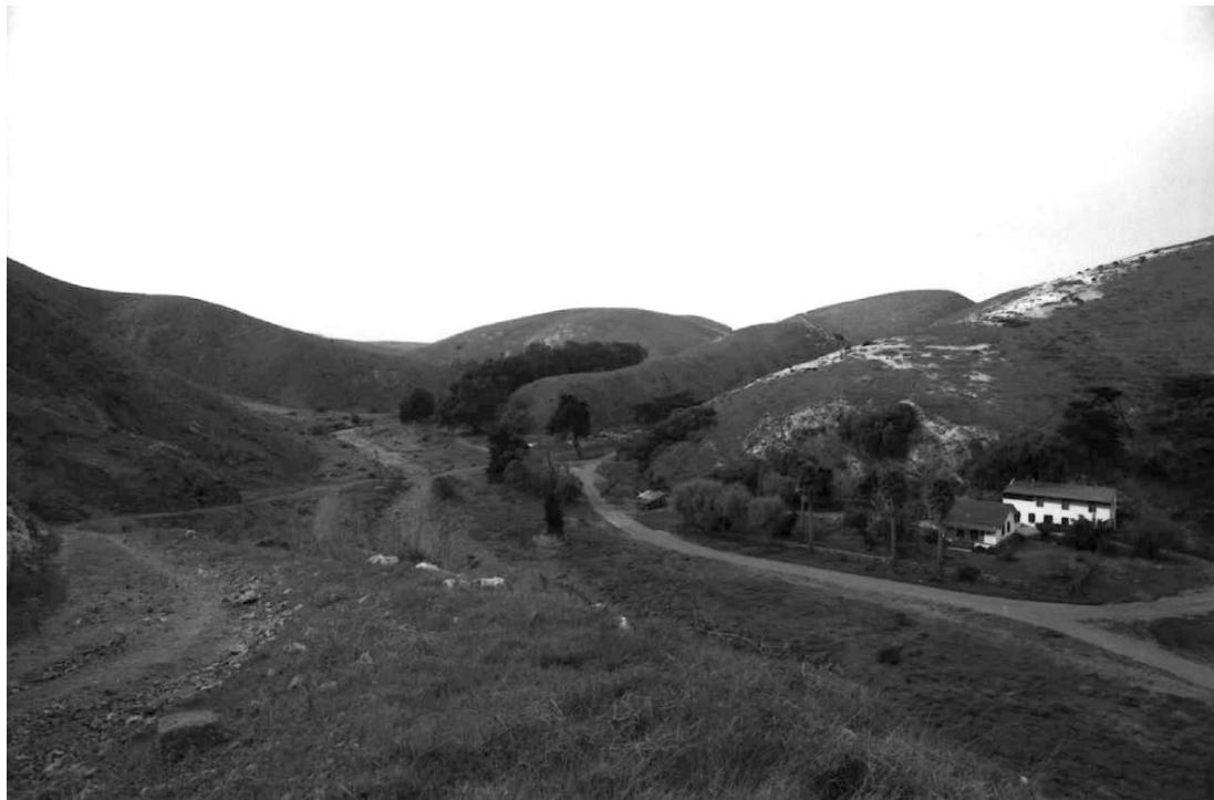
Circulation #1: View of some of the branches of Scorpion Canyon Road. The intersection of Smugglers Road, Scorpion Canyon Road, and the Service Road is at the center of the photo. (PGSO, CLI, CHIS-N-0013-33, 2003)
