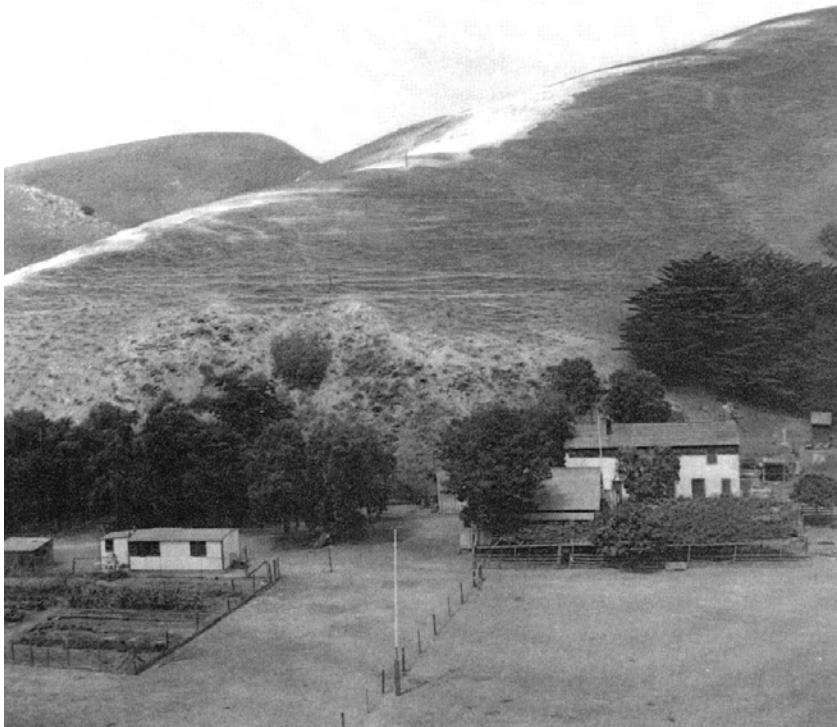
History #9: Historic view of Scorpion Ranch residential area, September 1959. (Photo courtesy of John Gherini)
