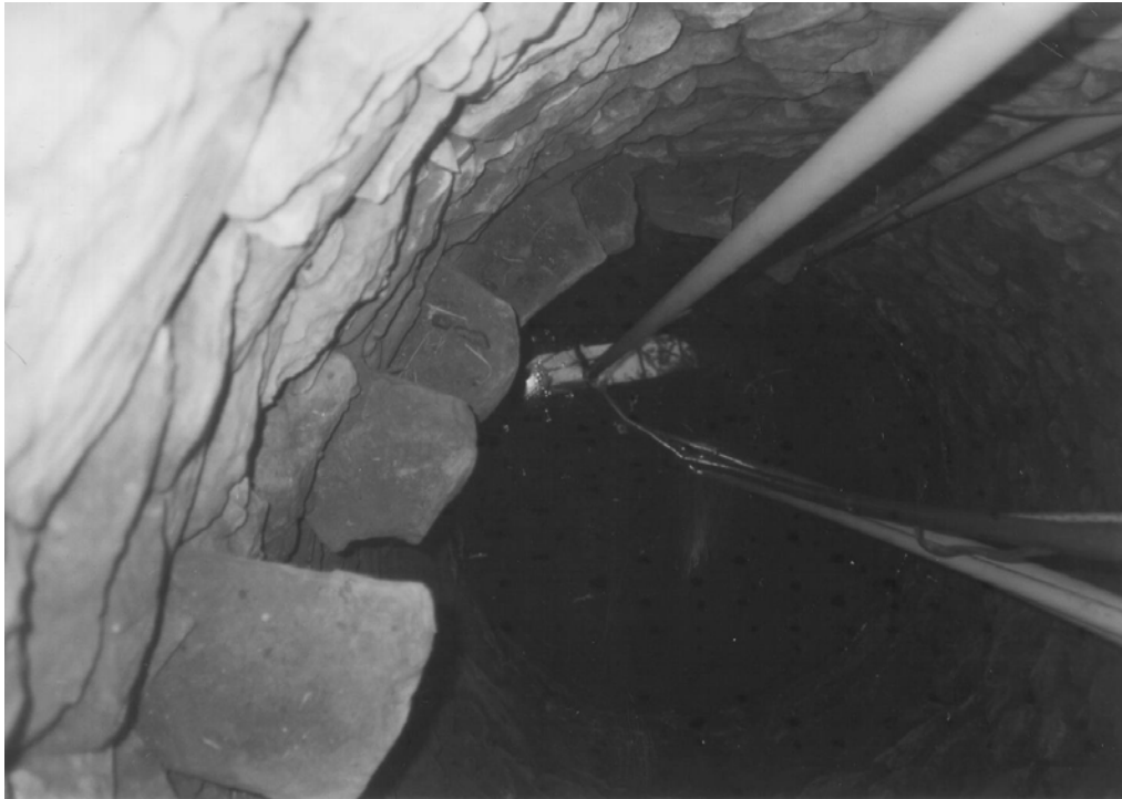
Small Scale Features #4: View down the Smugglers Ranch well. Note the stone steps. (PGSO, LCS files, 1999)
