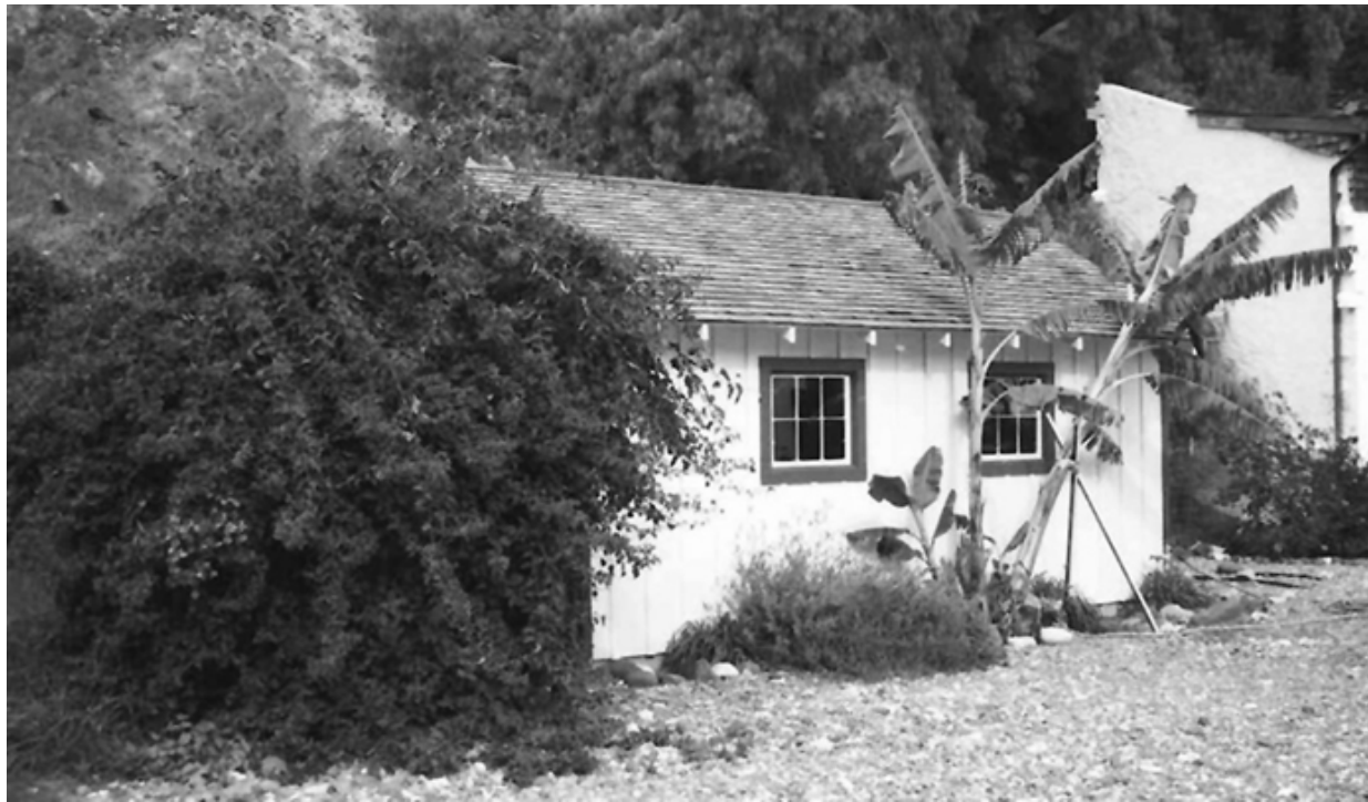
Buildings and Structures #2: View of the kitchen at Scorpion Ranch. Non-contributing bougainvillea and banana has been planted on the south side of the building. Scorpion ranch house is on the far right. (PGSO, CLI, CHIS-N-0013-20, 2003)
