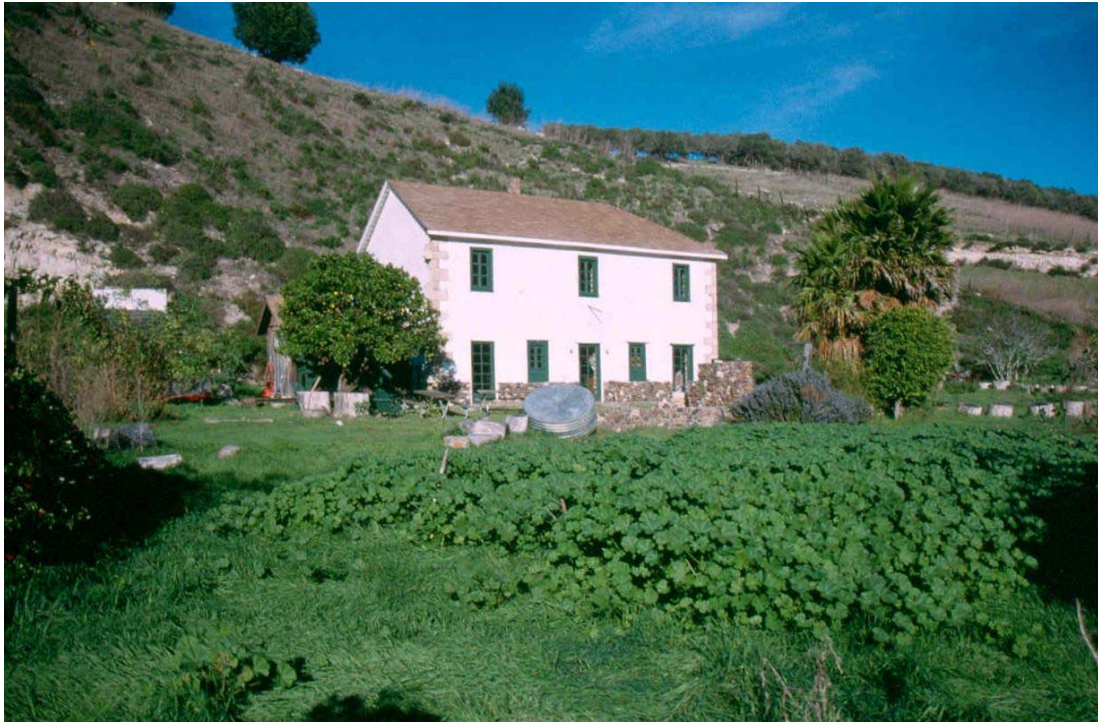
Buildings and Structures #6: View of Smugglers ranch house. (PGSO, CLI, CHIS-S-0007b-18, 2003)
