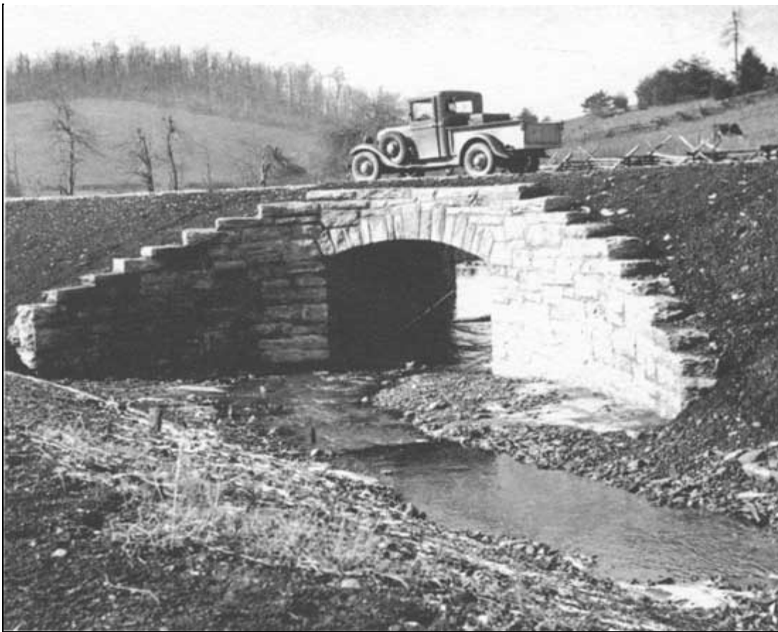
A 1936 view of a culvert headwall, single box culvert.
