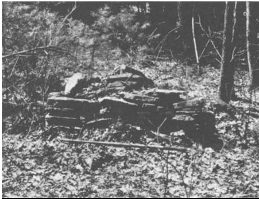
Plate 3. Historic house foundation, French Broad County, North Carolina.
