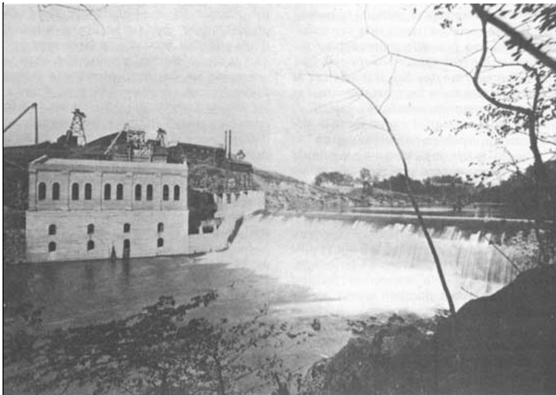
Plant of the Tennessee Eastern Electric Company on the Nolichucky River, nine miles south of Greeneville Source: Tennessee Division of Geology bulletin 17 (1914).
