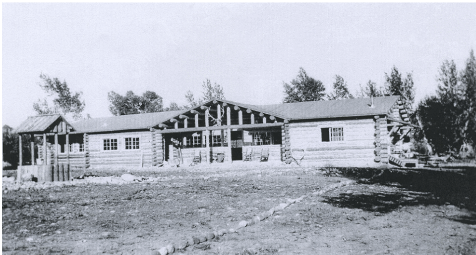
View looking east at front façade of lodge and well house during construction, 1927. Note the line of stones in foreground. Source: Jackson Hole Historical Society and Museum, [1958.1815.001].
