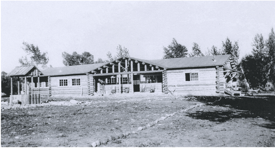
Figure 1. Looking east toward the front of the Lodge nearing completion. Note the well housing in front of the building. Source: Jackson Hole Historical Society and Museum, [1958.1801.01N].
