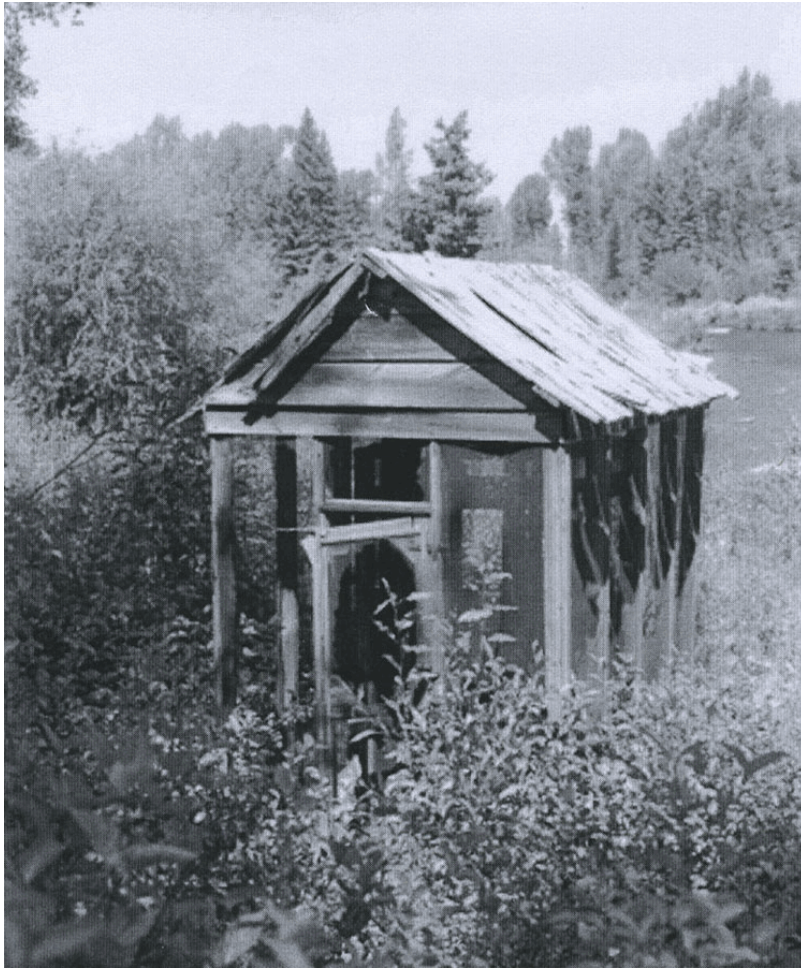
View looking north at curing house and Snake River, no date. Source: Jackson Hole Historical Society and Museum, [1989.2295.001].
