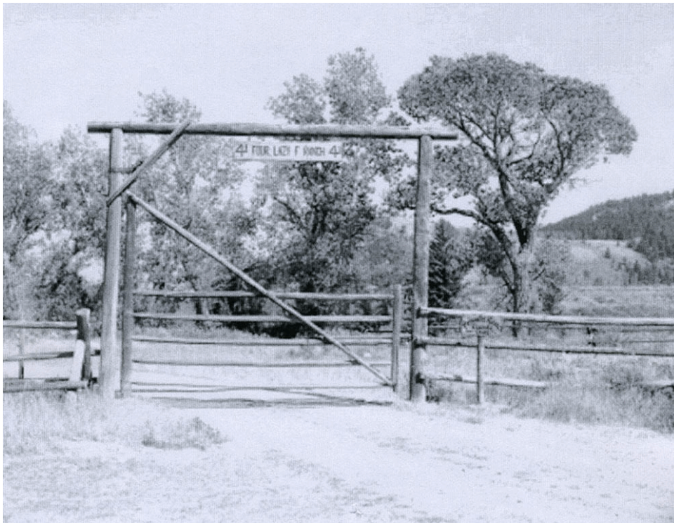
View looking north/northeast at ranch gate along road from Menor's Ferry, no date. Source: Jackson Hole Historical Society and Museum, [1989.2298.001].
