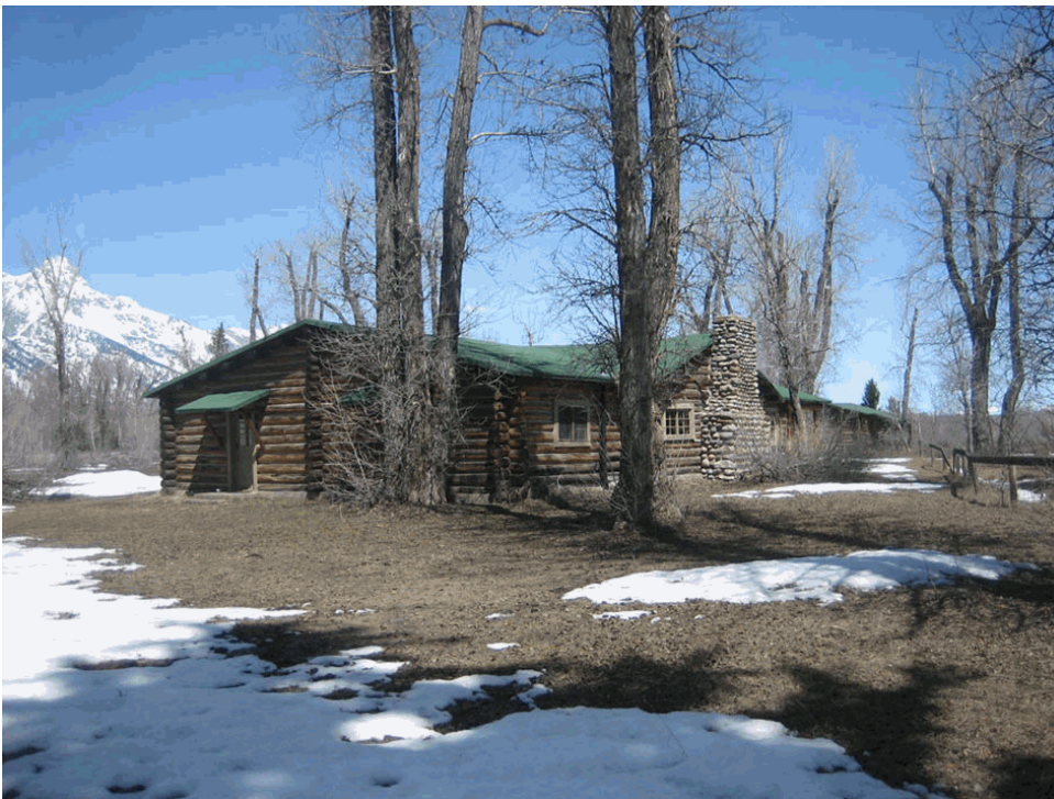
View looking northwest at south and east elevations of lodge, 2010. Note the growth in vegetation. Source: C. Mardorf, NPS.
