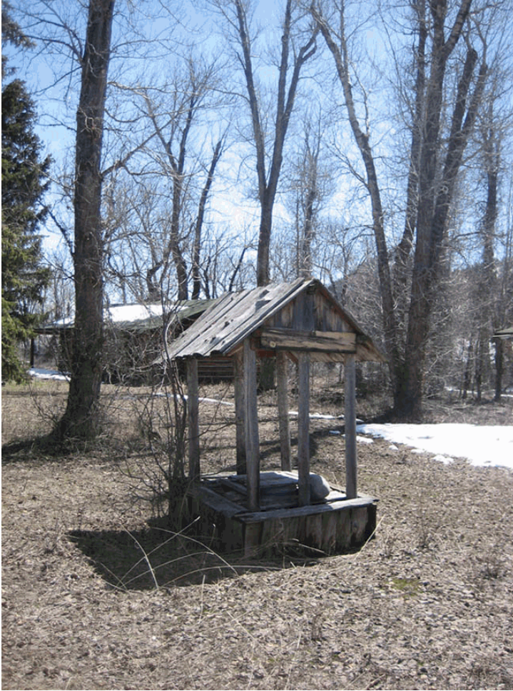
View looking east toward well house near Middle Cabin. Mrs. Oliver's cabin in background, 2010. Note significant deterioration of the structure. Source: C. Mardorf, NPS.
