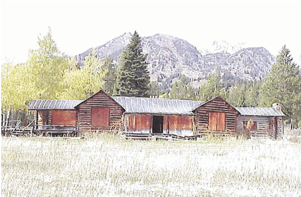
East (front) wall of HS-1168, the Main Cabin, 2004. Source CLR.
