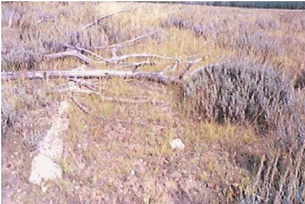
Looking north, the concrete foundation wall marking the site of the Messler Cabin, north of Cabin 8, 2004. Source CLR.
