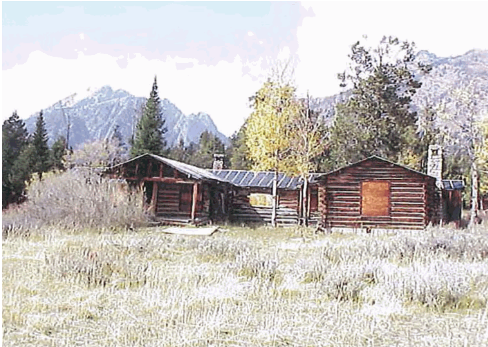
Front (east) wall of HS-1156, Hammond Cabin, 2004. Source CLR.
