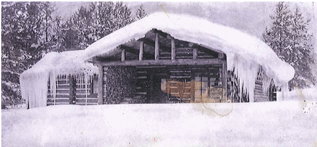
Hammond Cabin, HS-1156, circa 1925, prior to additions. Source CLR.
