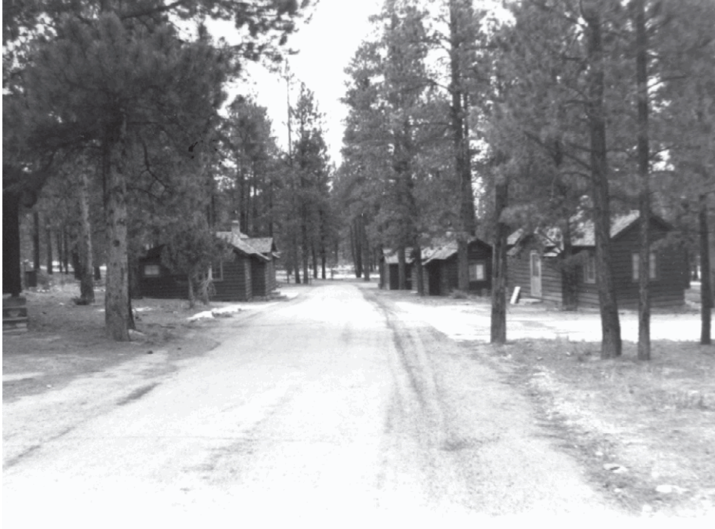
View of the Old NPS Housing Area, 1990 (BRCA Archives 3943 BRCA-00408).
