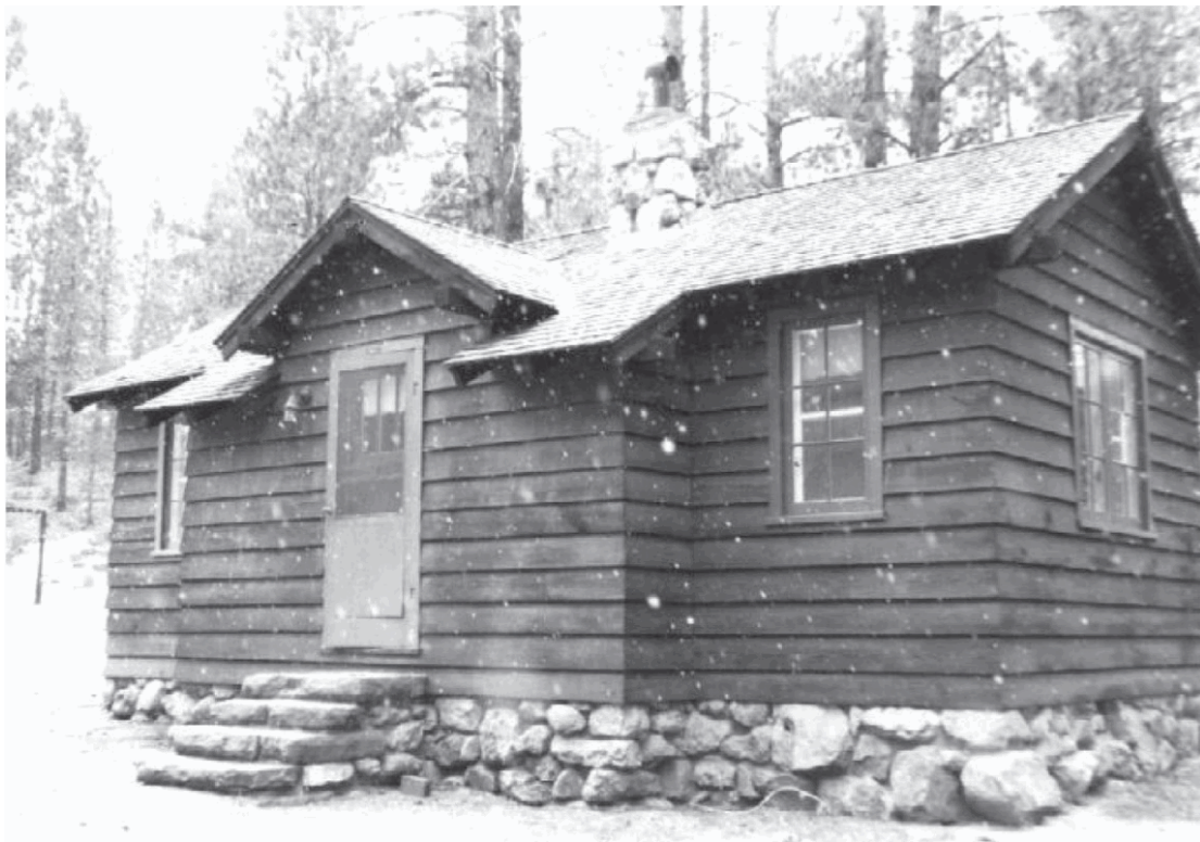
Employee Residence in Old NPS Housing Area with simplified rustic design, nd. (BRCA Archives, BRCA 3943 BRCA-00408).
