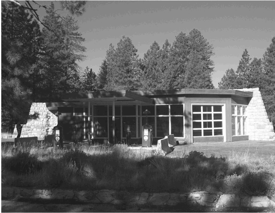
View of Service Station, HS-117 (2009 CLR).
