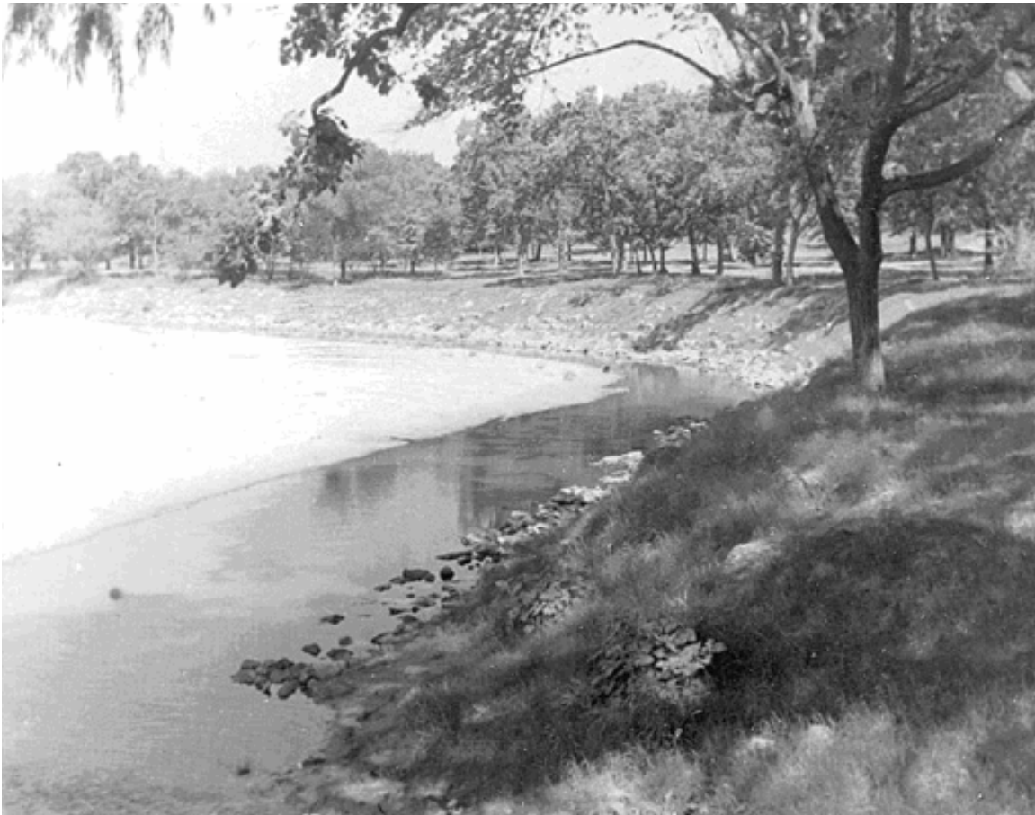
Two views of the completed bank stabilization along Rock Creek, with Flower Park in background, circa 1935
