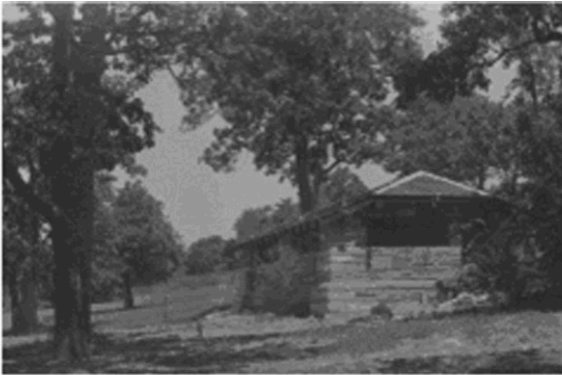
Completed Flower Park comfort station, 1935. (CNRA archives, photograph CMST-FP)
