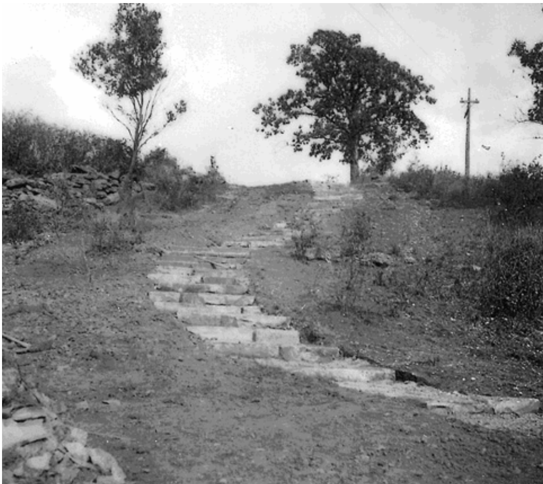
Stone stairs west of comfort station, circa 1935. (CNRA archives, photograph fac19)
