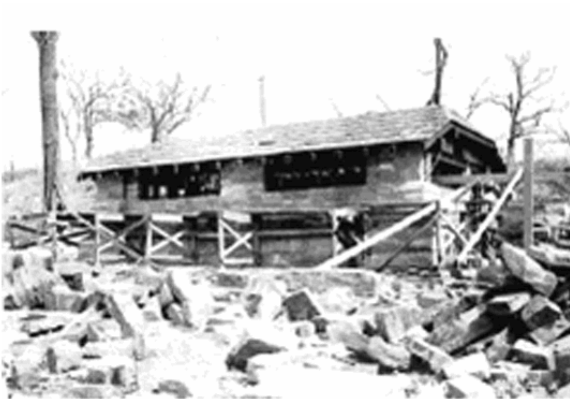
Flower Park comfort station under construction, 1934. (CNRA archives, photograph. CMST-FP2)
