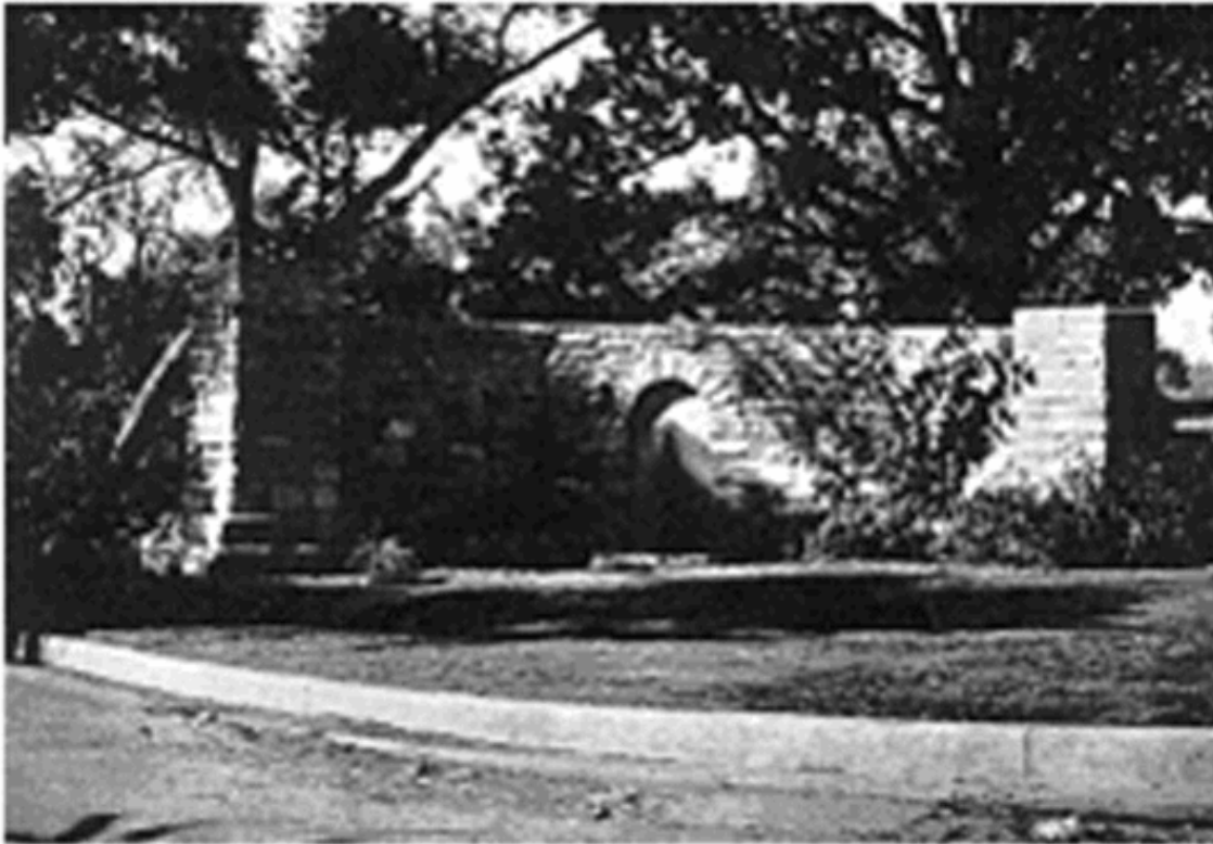
Completed wall and pier composition at the Main Entry, circa 1934. Note the ornamental plantings around the masonry structure. (Photograph from Park and Recreation Structures by Albert Good)
