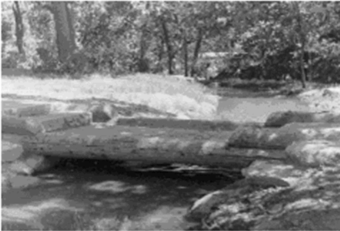
Log Bridge at end of Vendome stream, circa 1935. (CNRA archives, photograph fac04)
