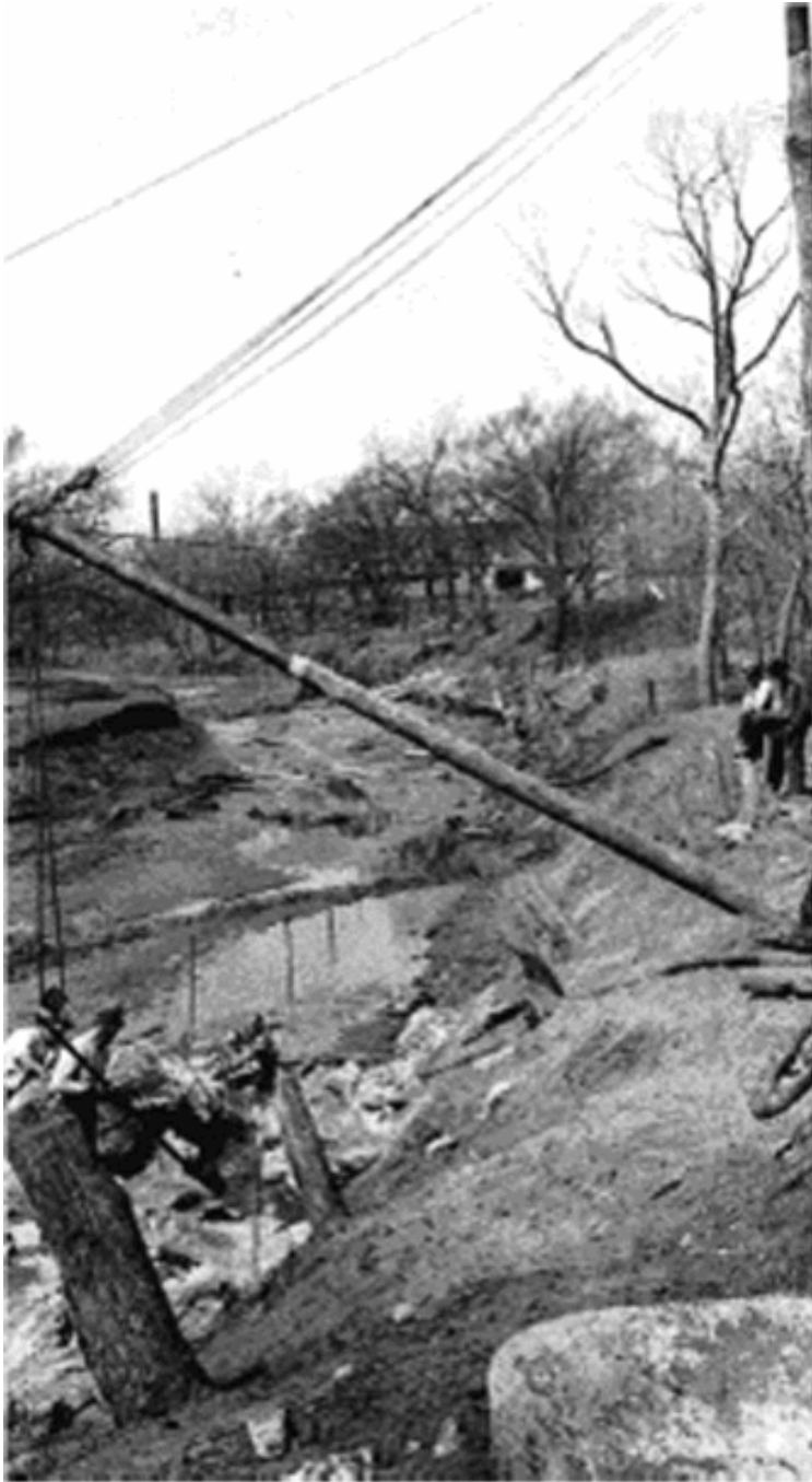
Placement of rip-rap using winches at the Flower Park revetment wall, 1934. (CLR 2004, 92)
