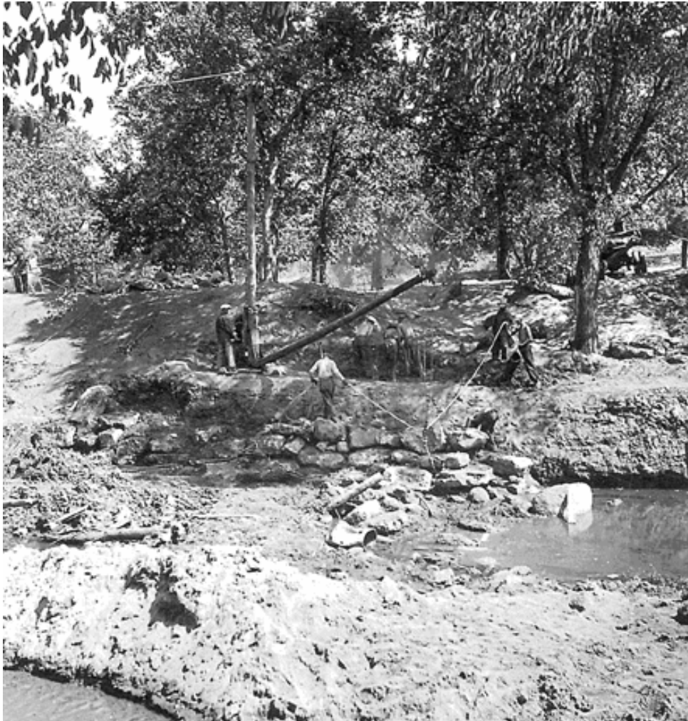
Revetment wall construction, 1934. (CNRA archives, photograph fac 16)
