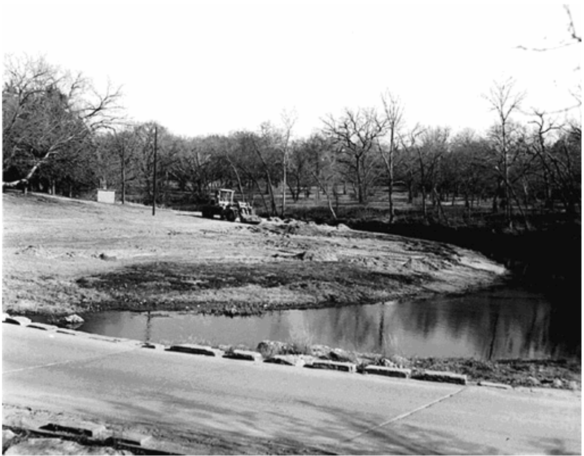
Post-flood sand removal at beach below Black Sulphur Springs Pavilion (prior to causeway reconstruction), date unknown. (CNRA archives, photograph 514)
