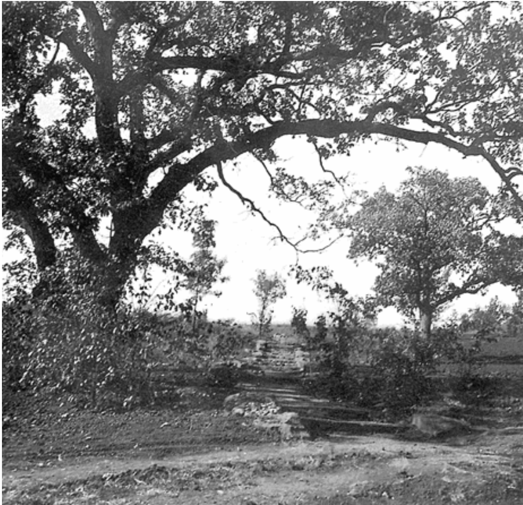
Stone stairs east of comfort station, circa 1935. (CNRA archives, photograph fac20)
