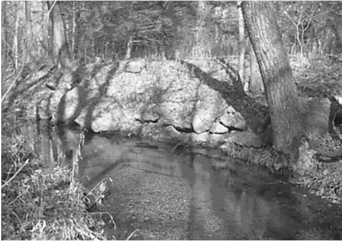
Rip-rap of Travertine Creek bank near Antelope and Buffalo Springs area, no date. (CNRA archives, GIS photograph)
