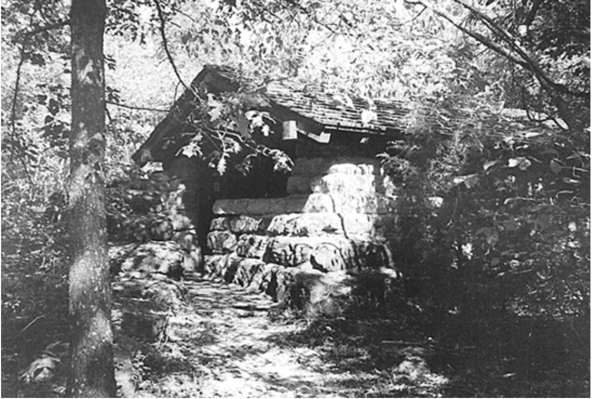
Buffalo Springs Comfort Station, 1992. (CNRA archives, LCS photograph)
