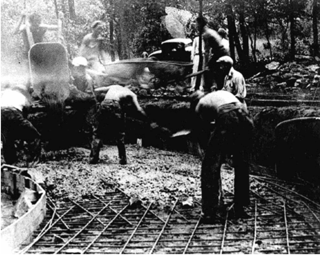
Pouring concrete at Buffalo Springs, circa 1934. (CNRA archives, LCS photograph)
