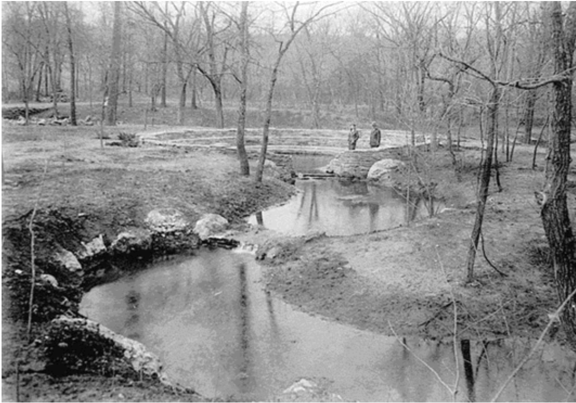
"Lotus" ponds below Buffalo Spring spillway, just after construction, circa 1935. (CNRA archives, LCS photograph)
