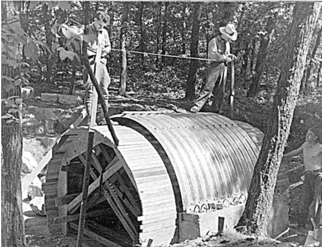
Construction of stone arched footbridge in Buffalo Springs area, circa 1934. (CNRA archives, photograph fac.05)
