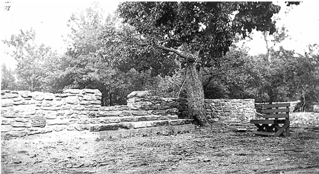
Stone wall at Buffalo Springs parking area, above picnic area, circa 1934. (CNRA archives, photograph fac27)
