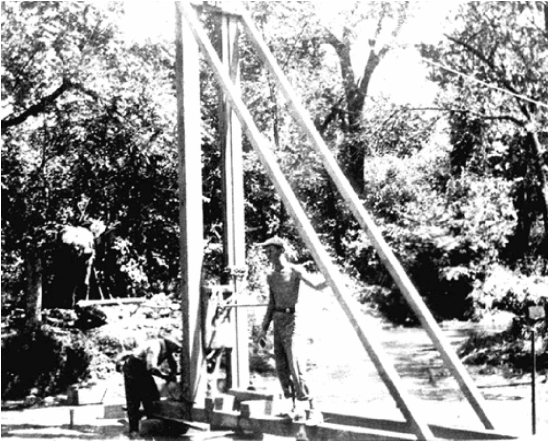
Pile driver for white pine log pilings for foundation of Buffalo Springs circular pool platform, circa 1934. (CNRA archives, LCS photograph)
