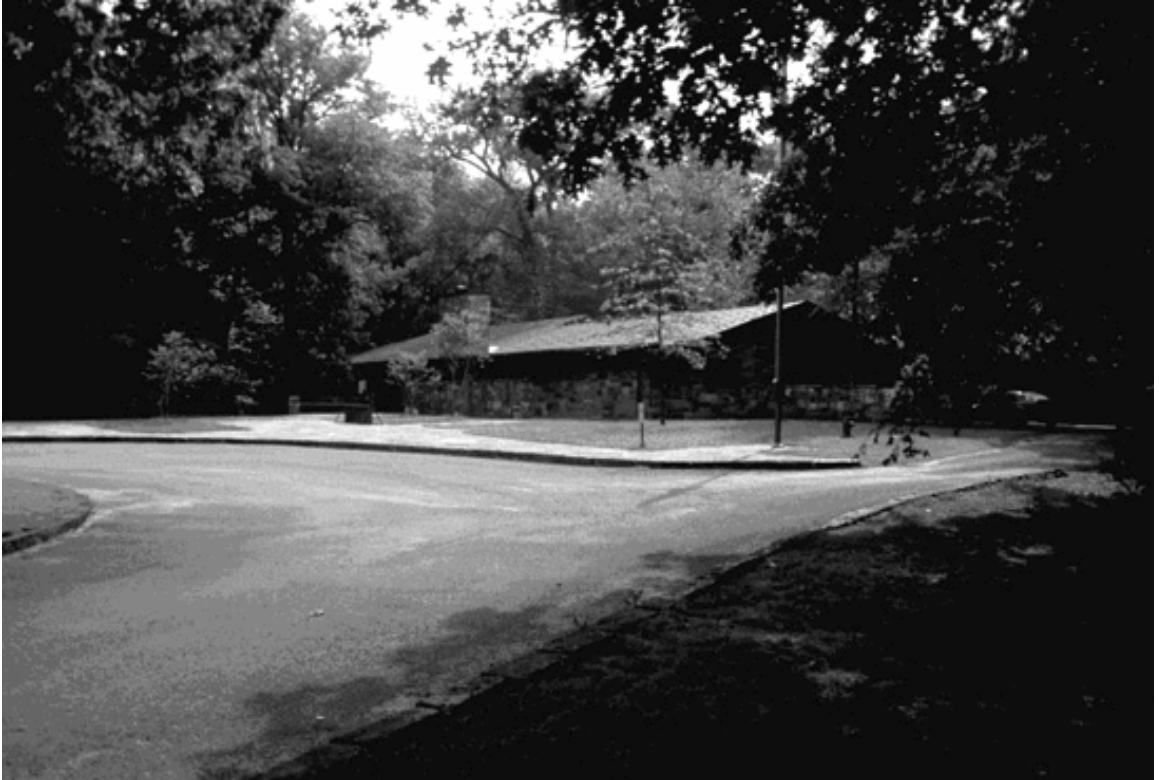
Parking area at Travertine Nature Center, looking northeast from entry, 1999. (Photograph by harlen Groe)
