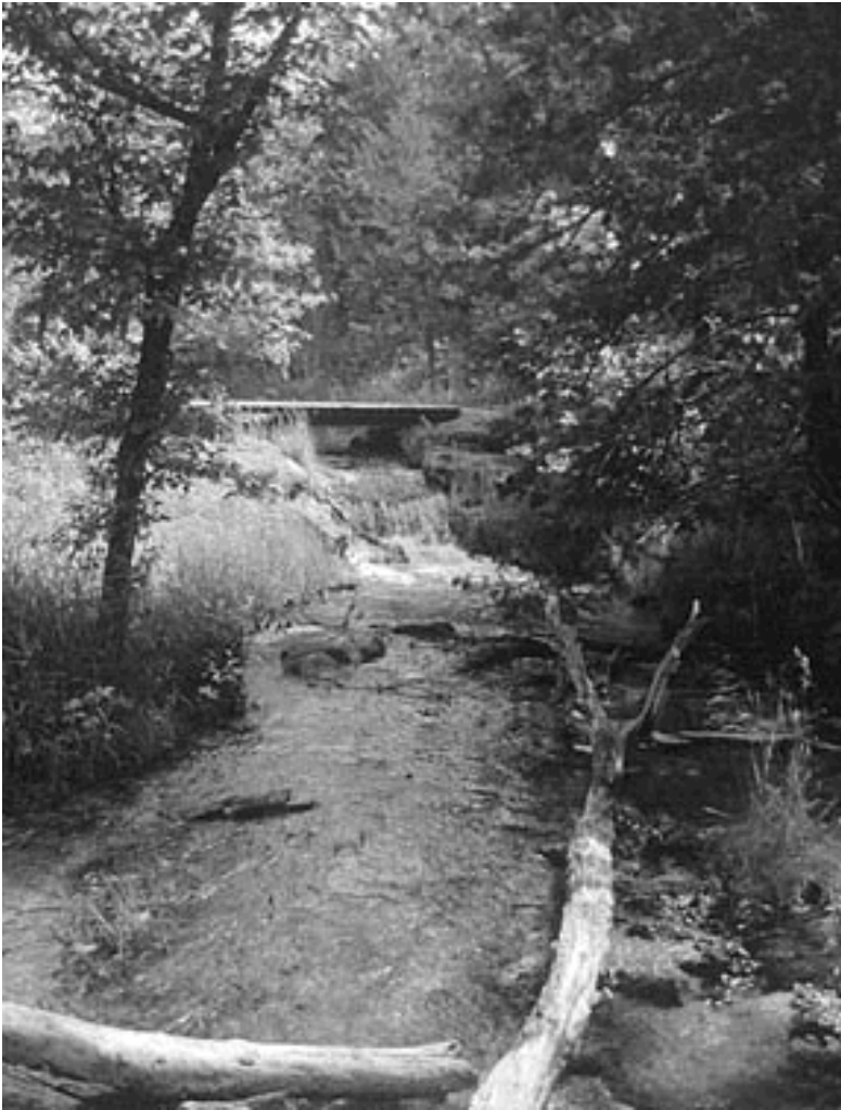
Wood footbridge crossing Travertine Creek near Antelope Springs (middle bridge); likely replacement. (photograph by harlen Groe)
