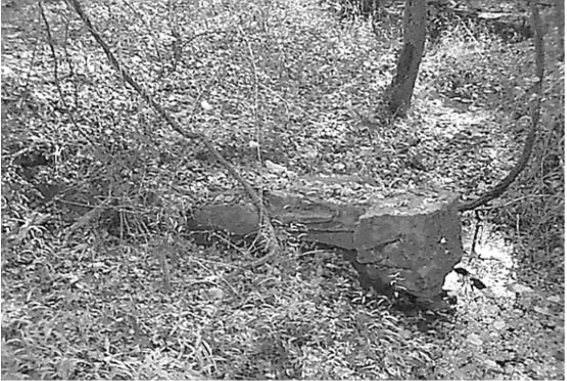
Stone stream dam (second of three), no date. (CNRA archives, GIS photograph)
