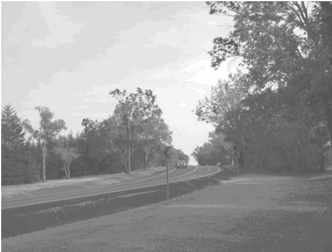
Highway 177 after resurfacing, view south at curve near Buffalo Overlook, 2001. (Photograph by Iowa State University).
