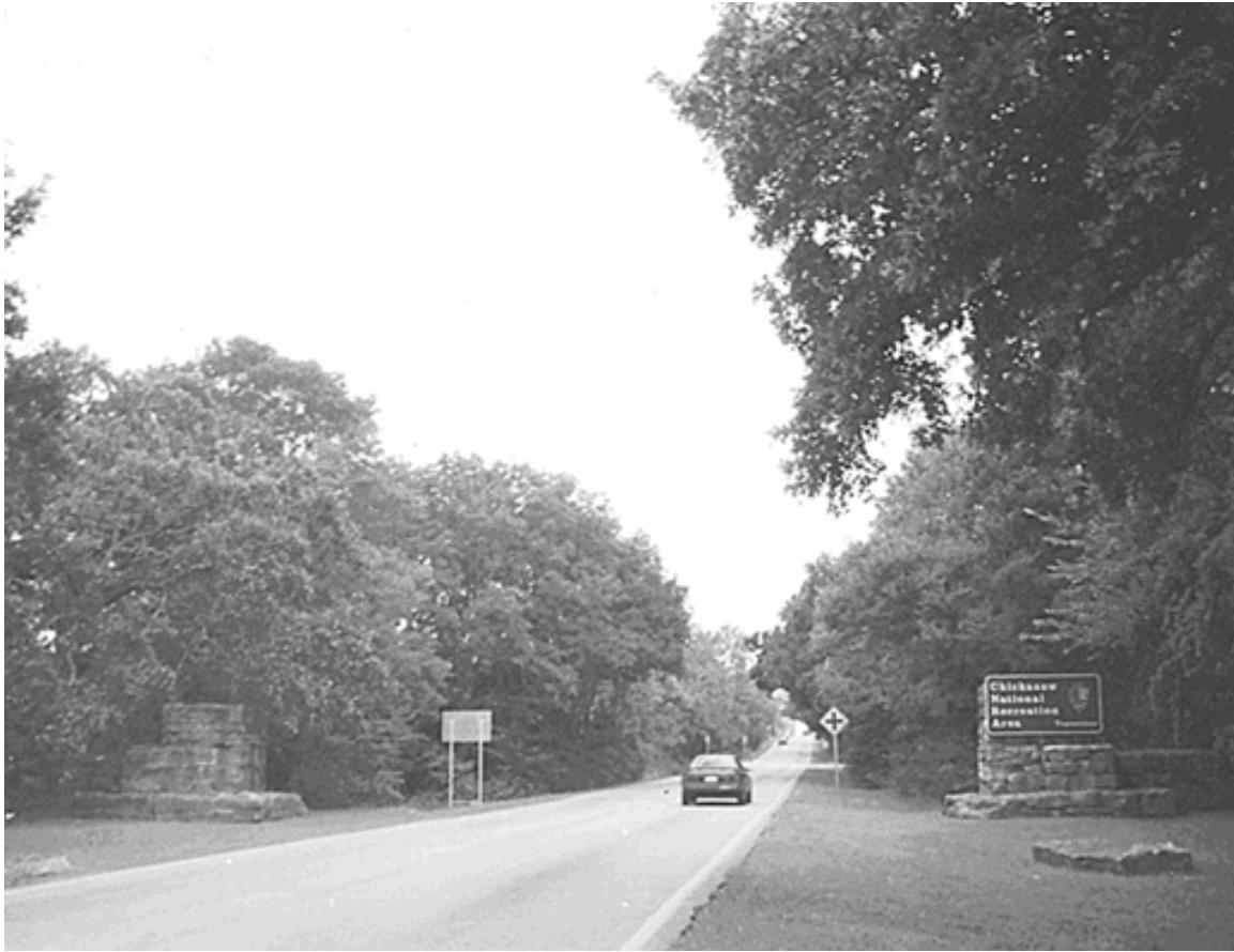
View of entry piers at the park's south entrance along Highway #177, 1992. (CNRA archives, LCS photograph)
