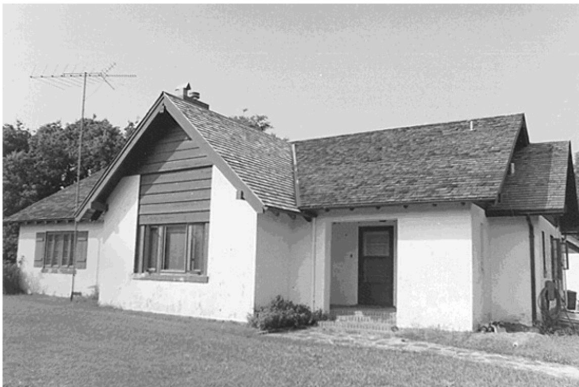
Front façade of Superintendent's Residence, 1992. (CNRA archives, LCS photograph)
