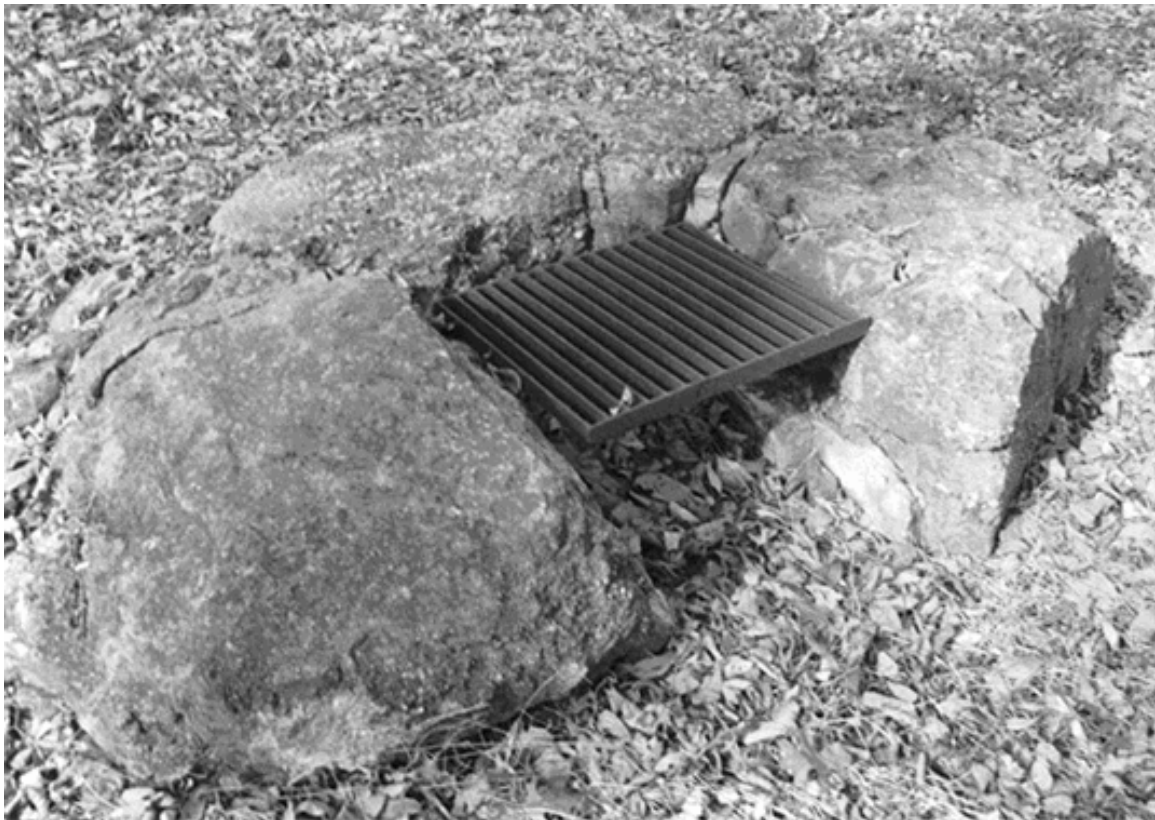
CCC fireplace at Walnut Grove (WG.A1), circa 2000. (CNRA archives, LCS photograph)
