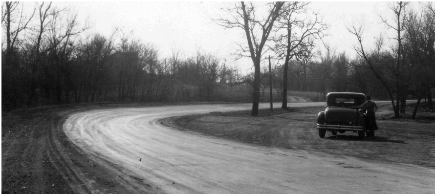
Section of Perimeter Road under construction. Source: Park files.
