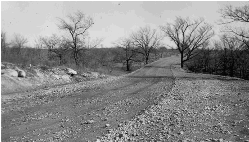
Construction of the perimeter road near Buffalo Springs road culvert, circa 1934. Picture shows completion of rough grading. Note the parking lot on the right. Source: Park files; CLR 2004, 70.
