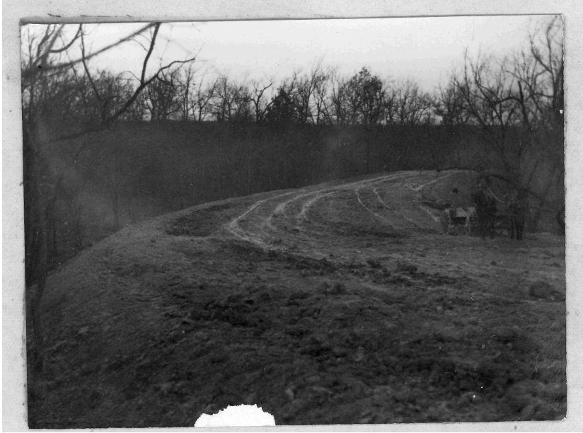
Perimeter road under construction (nd). Source: Park files.
