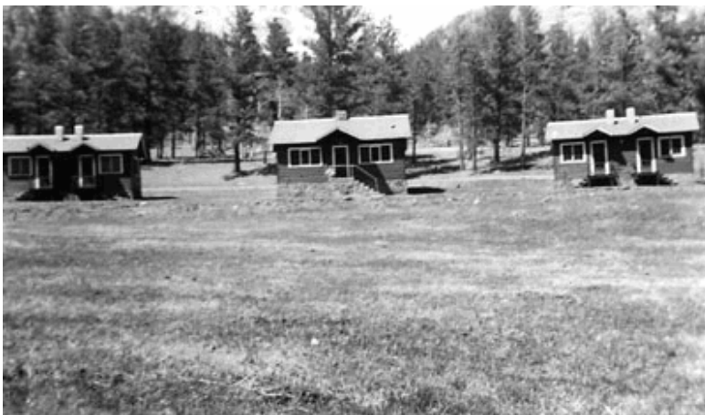
Photo 9: View of newly constructed guest cabins, ca. 1936. Source: McGraw family.
