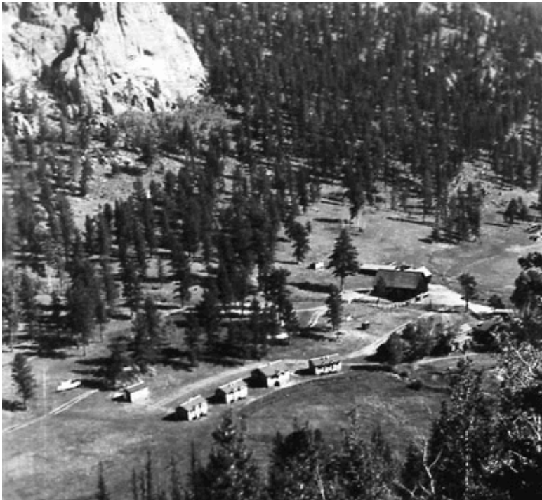
Photo 8: Oblique view of Ranch from the southwest, ca. 1936. The pond in this view is very small, on the west center right of the photo. It may have been partially drained to build the cabins. Source: McGraw family.
