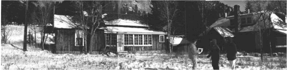
Photo 18(a): Bunk House and Main House, view from the south, 1998. Source: Shapins Associates.
