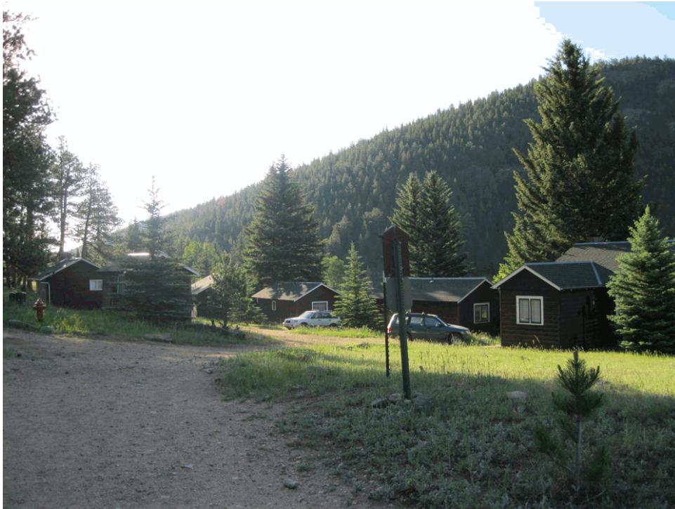
Access drive and parking areas adjacent to cabins, June 2012. Source: Meg Frisbie, NPS.
