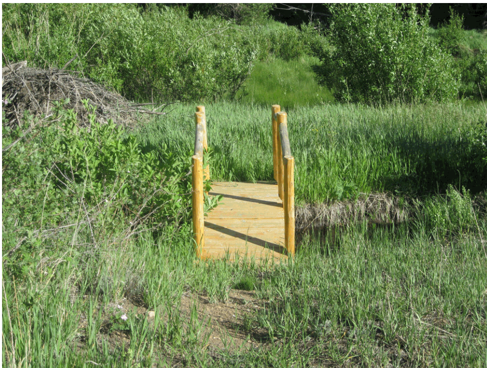
Wood bridge over Cow Creek, June 2012. Source: Meg Frisbie, NPS.
