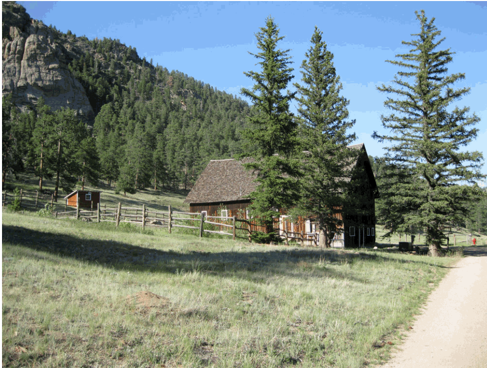
Barn, corral fence, June 2012. Source: Meg Frisbie, NPS.
