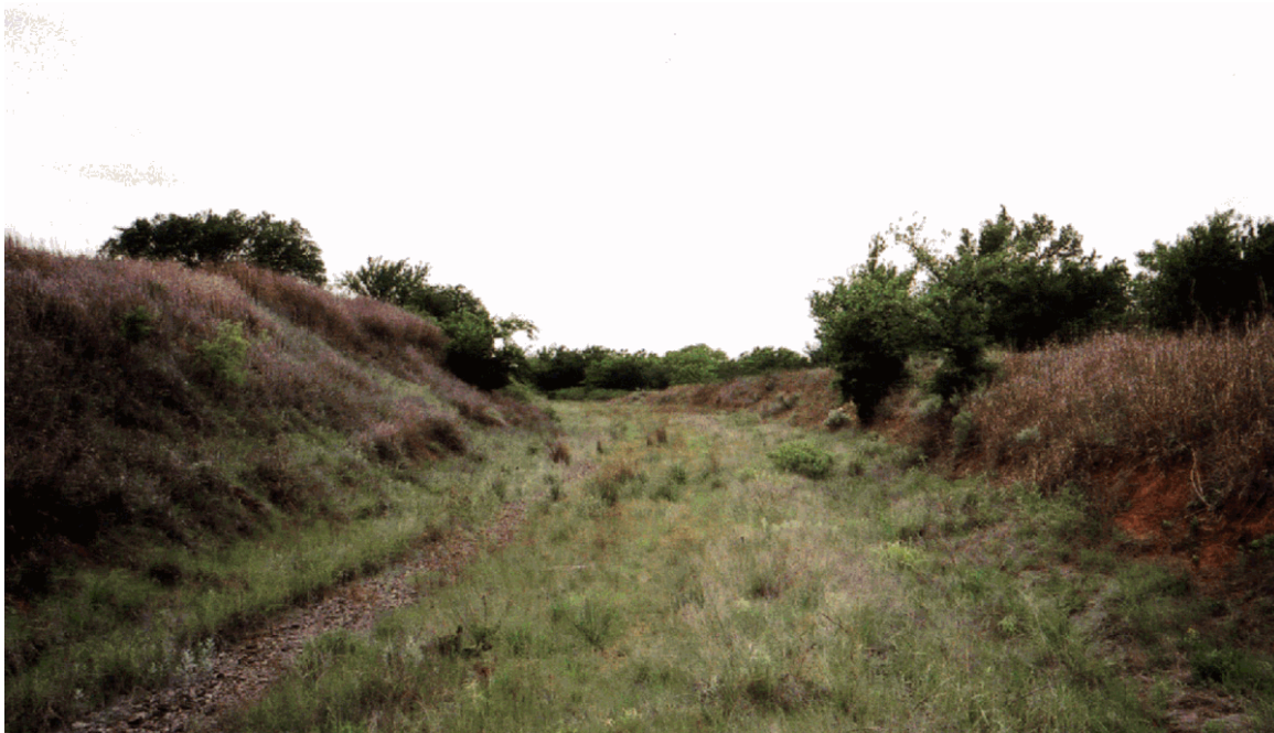
Eastern Railroad Grade, looking west, 2002. Source: John Milner Associates, CLR.
